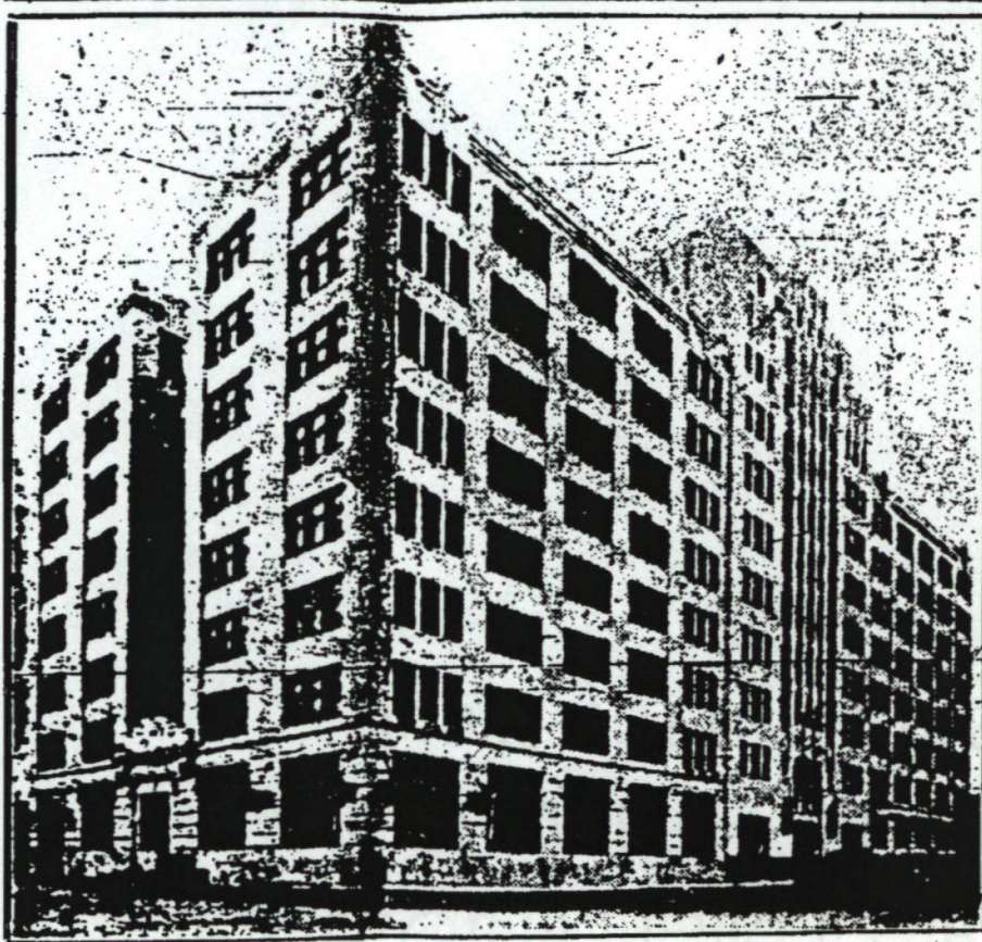
Galveston's Newest Office Building
