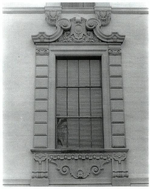
Figure 10. Detail of original multi-light casement window on Facility 900.
