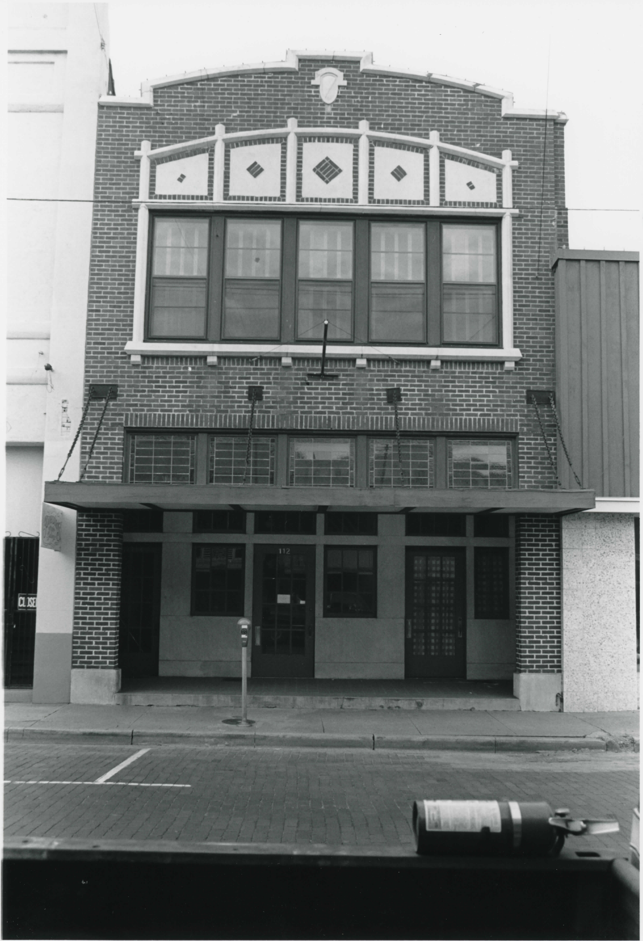
HAYTER OFFICE BUILDING NACOGDOCHES CO., TEXAS 4 OF 30
