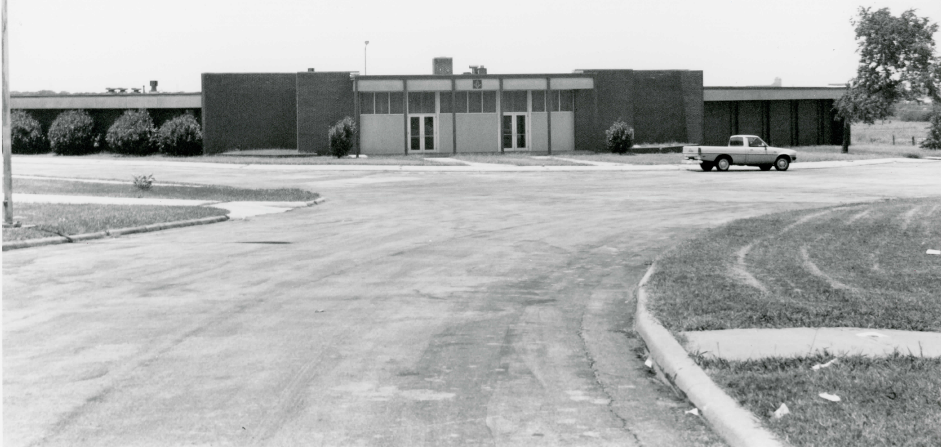
"SUB" - MASONIC HOME H.O. FORT WORTH, TARRANT CO., TEXAS PHOTOGRAPH 21 OF 26
