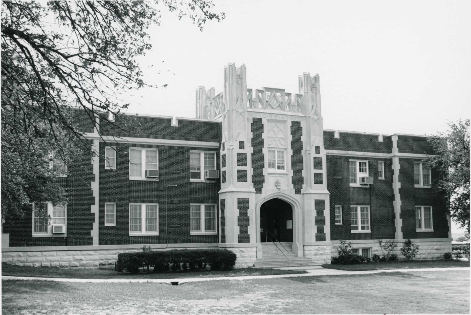
ADMINISTRATION BUILDING - MASONIC HOME H.O. FORT WORTH, TARRANT CO., TEXAS PHOTOGRAPH 7 OF 26
