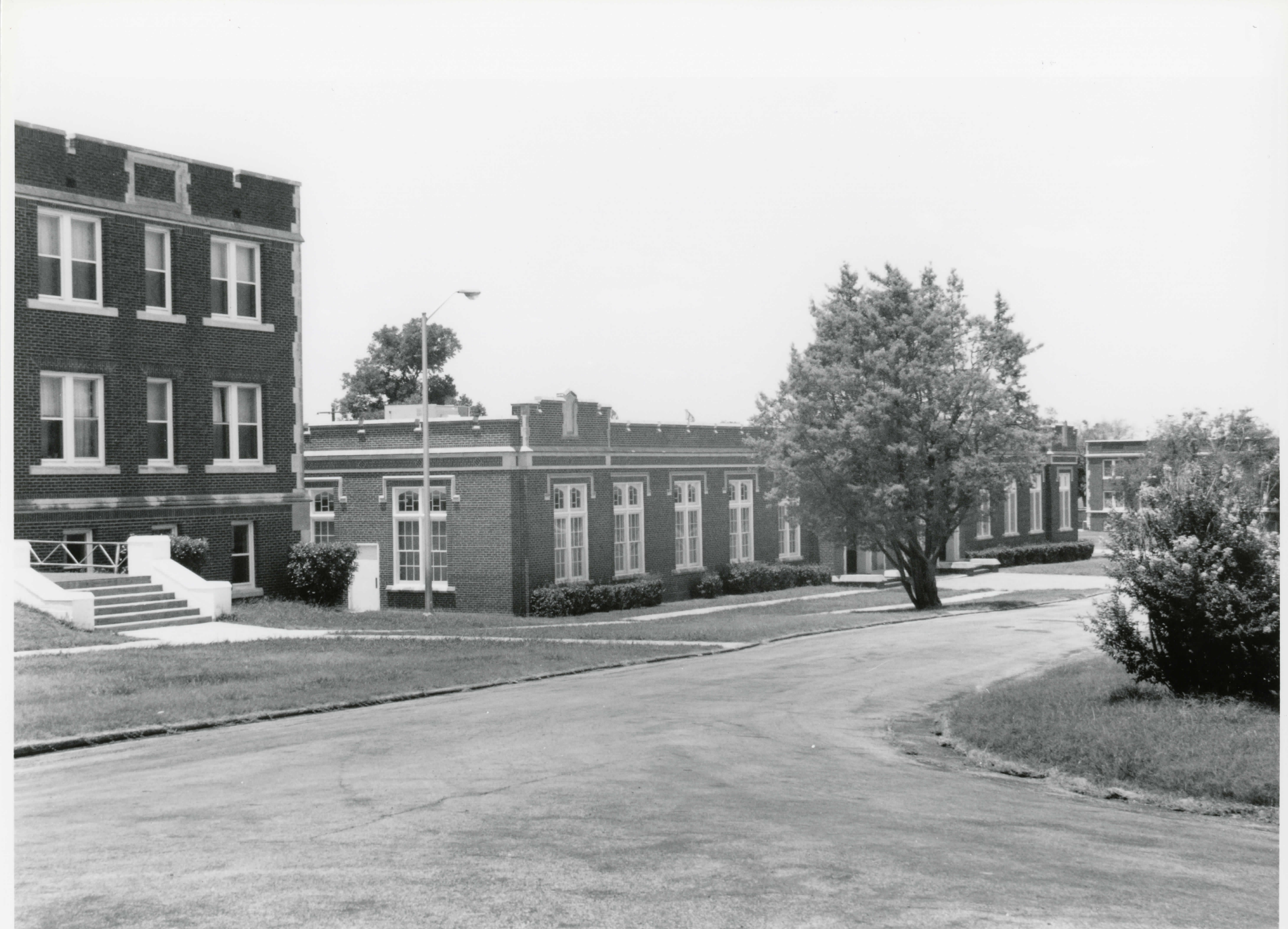
DINING HALL - MASONIC HOME H.D. FORT WORTH, TARRANT CO., TEXAS PHOTOGRAPH 9 OF 26
