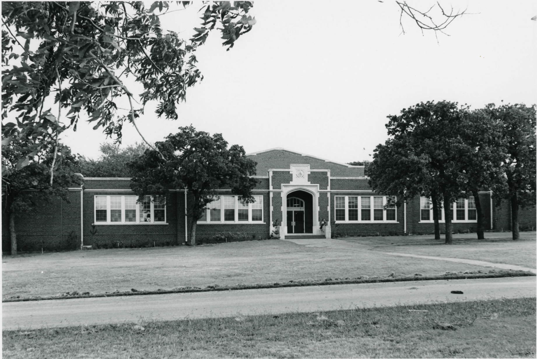
PRIMARY SCHOOL - MASONIC HOME H.D. FORT WORTH, TARRANT COUNTY, TEXAS PHOTOGRAPH 3 OF 26
