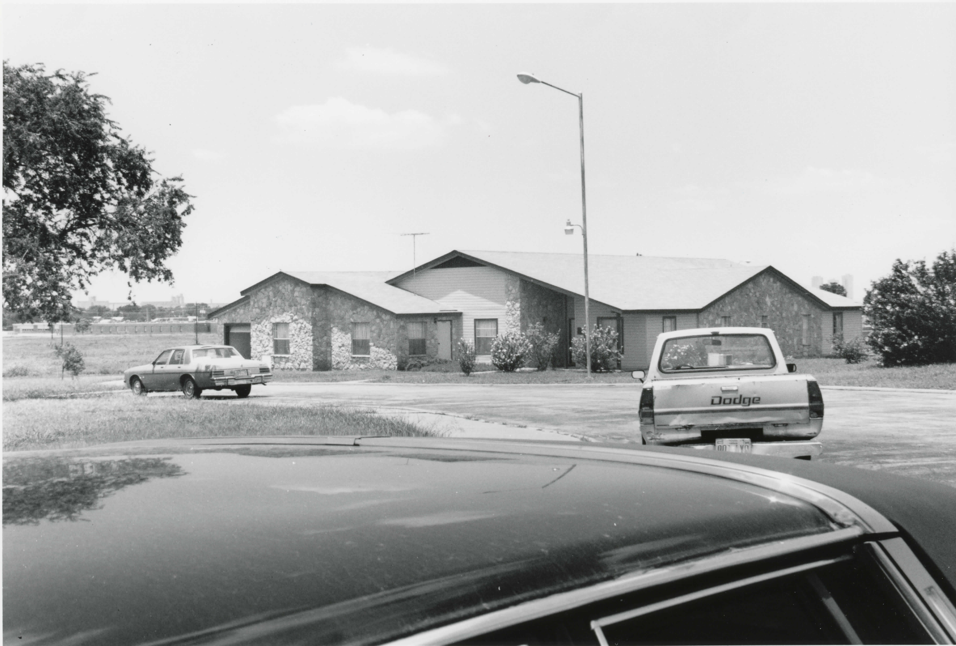
COTTAGE, SITE NO. 20, - MASONIC HOME H. FORT WORTH, TARRANT CO., TEXAS PHOTOGRAPH 23 OF 26
