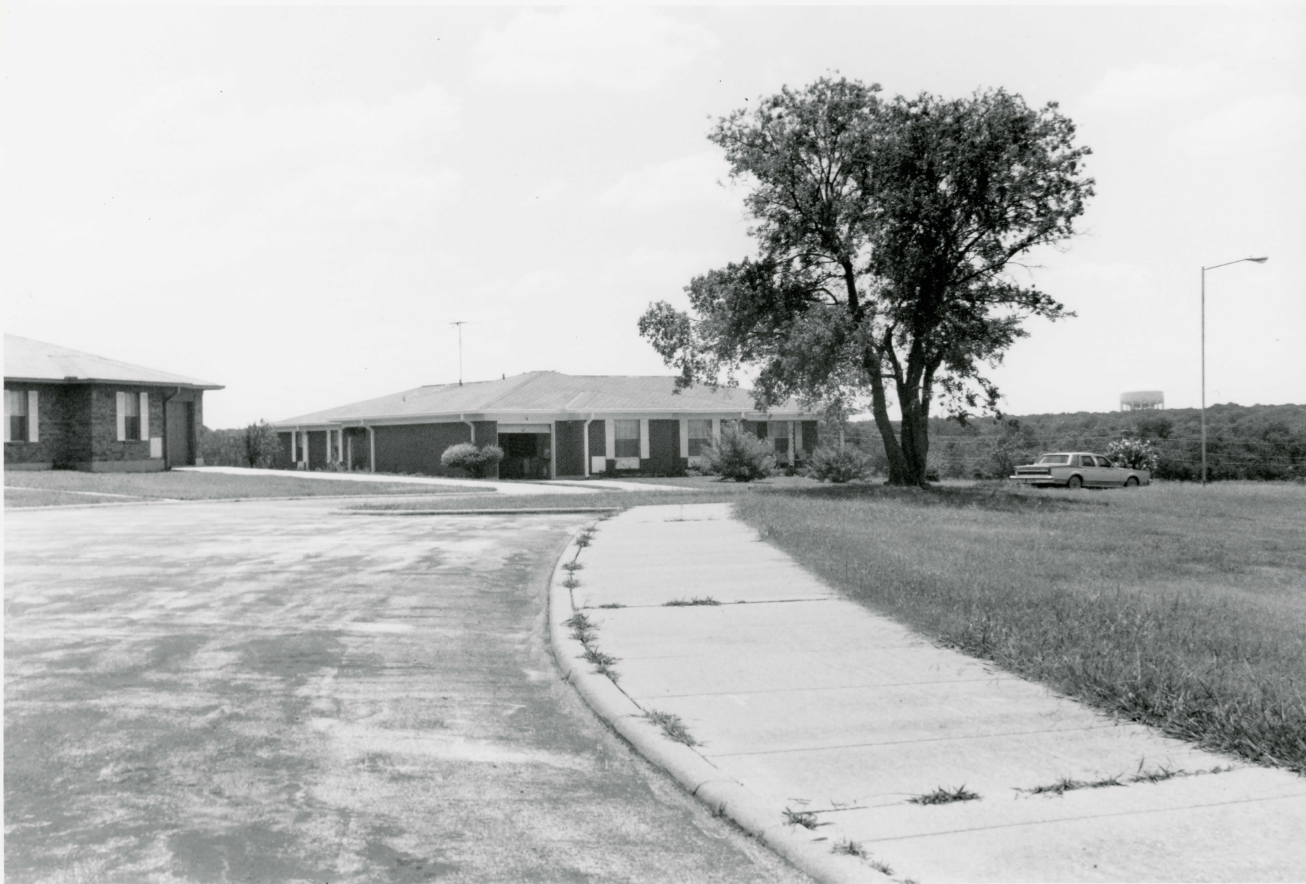
COTTAGE, SITE NO. 24, - MASONIC HOME H.O. FORT WORTH, TARRANT CO., TEXAS PHOTOGRAPH 25 OF 26
