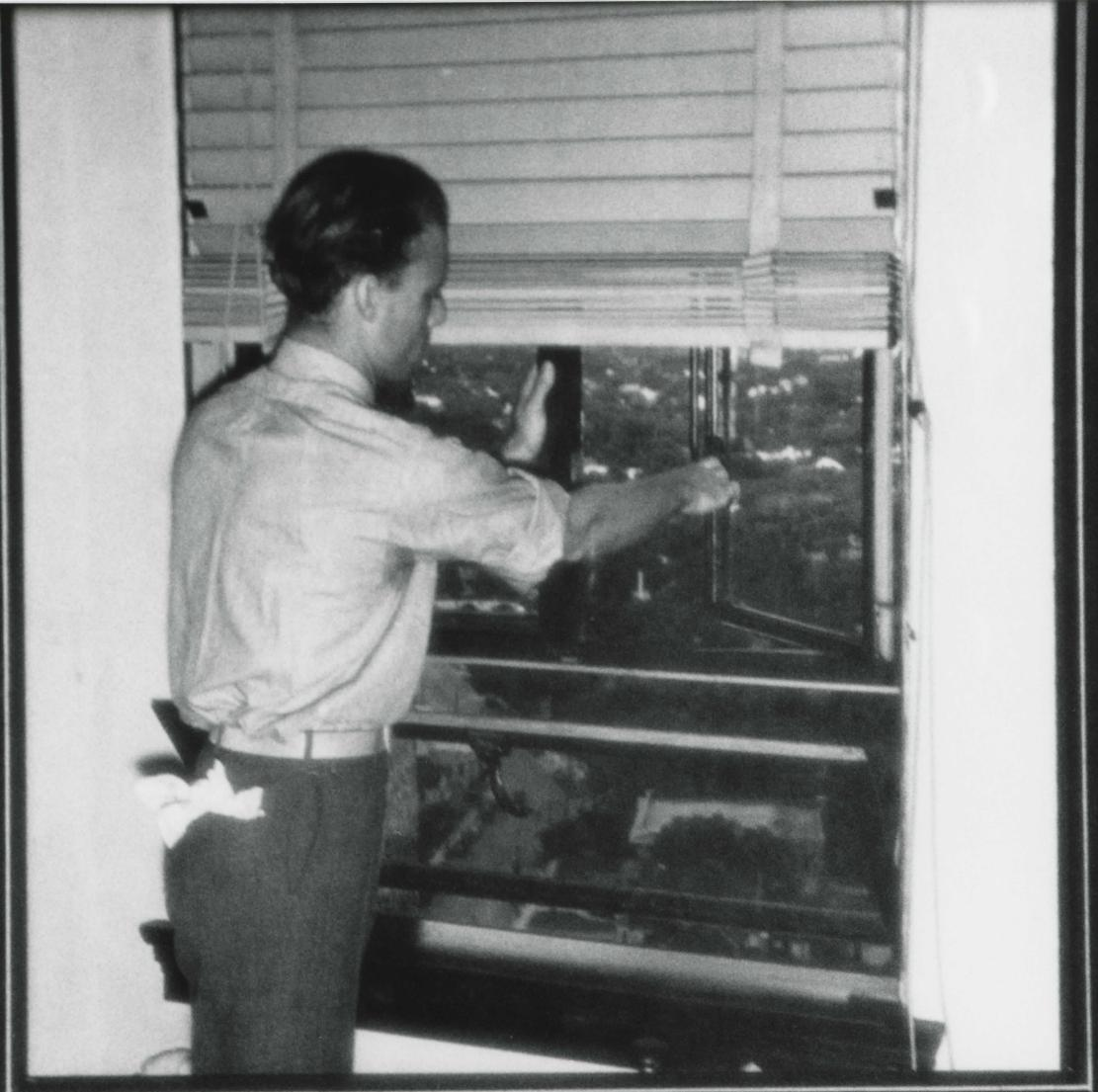
LUPTON COMBINATION STEEL CASEMENT WINDOWS THAT RUN NEARLY TO CEILING, ARE PLACED CLOSE TO EACH OTHER TO GIVE AN **EXTRA** ABUNDANCE OF LIGHT. THE LOWER SECTION OF THE WINDOW OPENS IN AND ACTS AS A WIND GUARD, WHILE THE UPPER SECTION OPENS OUT. THIS SPECIAL TYPE ALONG WITH THE OCTAGONAL TOWER CONSTRUCTION INSURES **100%** VENTILATION, WITH EVERY OFFICE AND OUTSIDE ROOM.
