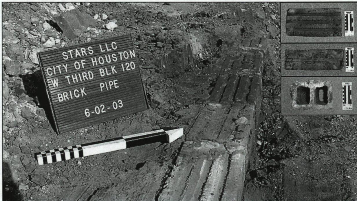
Figure 13. Section of Feature 6 hollow brick pipe exposed during STARS investigation. Bricks were each about 14 inches long, 8 inches wide, and 6 inches tall. Although no sources or dates of manufacture were established, apparently these bricks were installed during the late nineteenth or early twentieth century.
