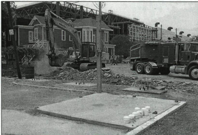
Figure 3. Trackhoe removal of concrete and asphalt overburden within the revised project area. Photo faces south. Note remnants of former gasoline service station foundations and parking areas in foreground and the historic Arthur B. Cohn house in background at upper left.
