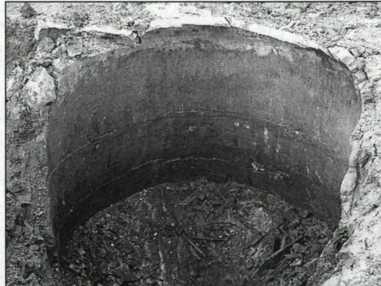
Figure 10. Oblique view of Feature 4 as partially sectioned using a trackhoe during the STARS investigation. Approximately the upper six feet are shown in this photograph. Feature 4 was another remnant of a large, bottle-shaped cistern lined with low-fired, hand-made brick set and sealed with fine-grained mortar. Archival evidence indicates that the original cistern was probably built by Alfred Hulbert at roughly the same time as the Feature 3 (Figure 8 and 9) cistern, in about 1859.
