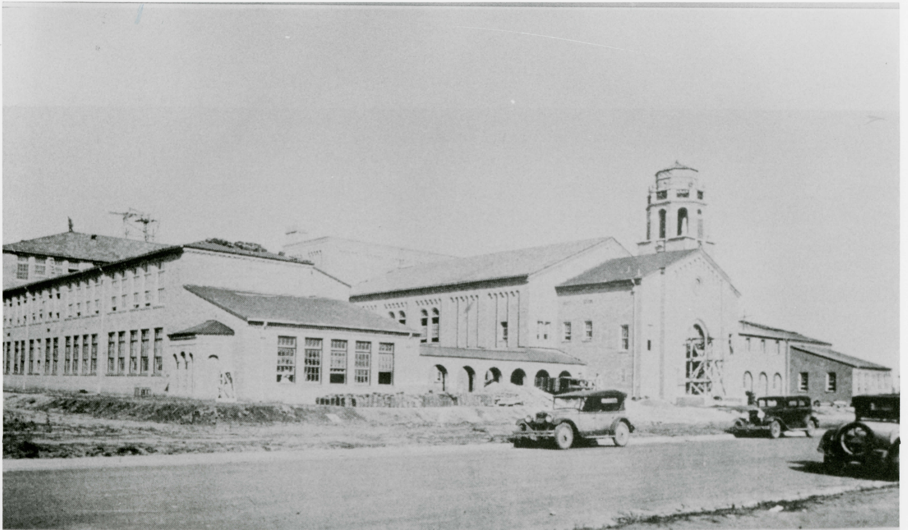
34. Lubbock High School Under Construction in 1931.
