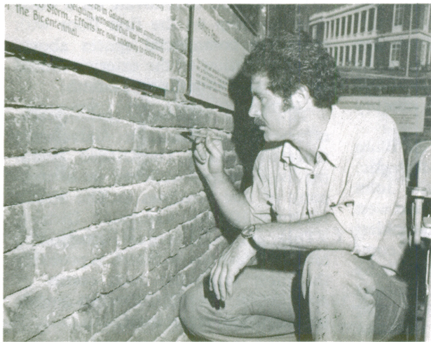
Building Conservation Technology's Joe Herndon inspected the mortar of the Ashton Villa carriage house as part of the firm's longterm maintenance survey on the landmark.
