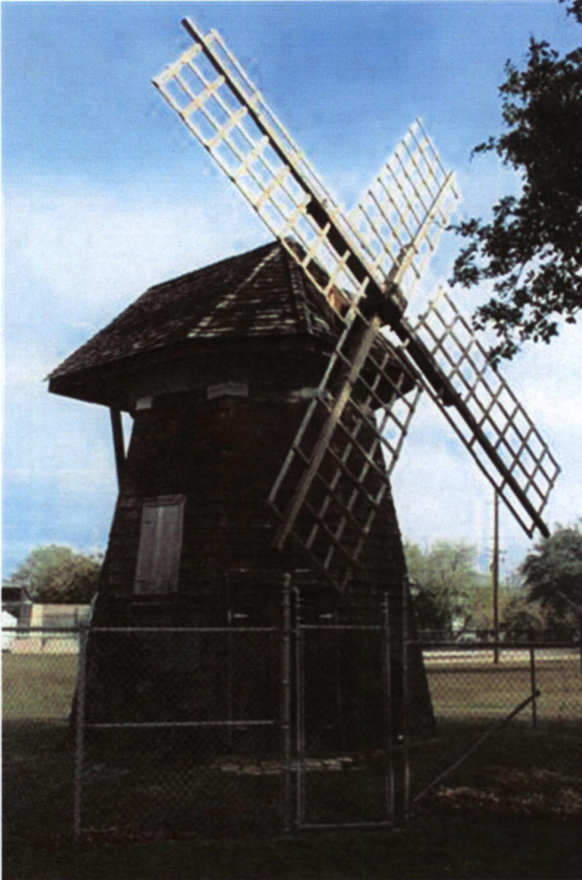
Figure 3 Windmill in its current location Camera Facing northeast
