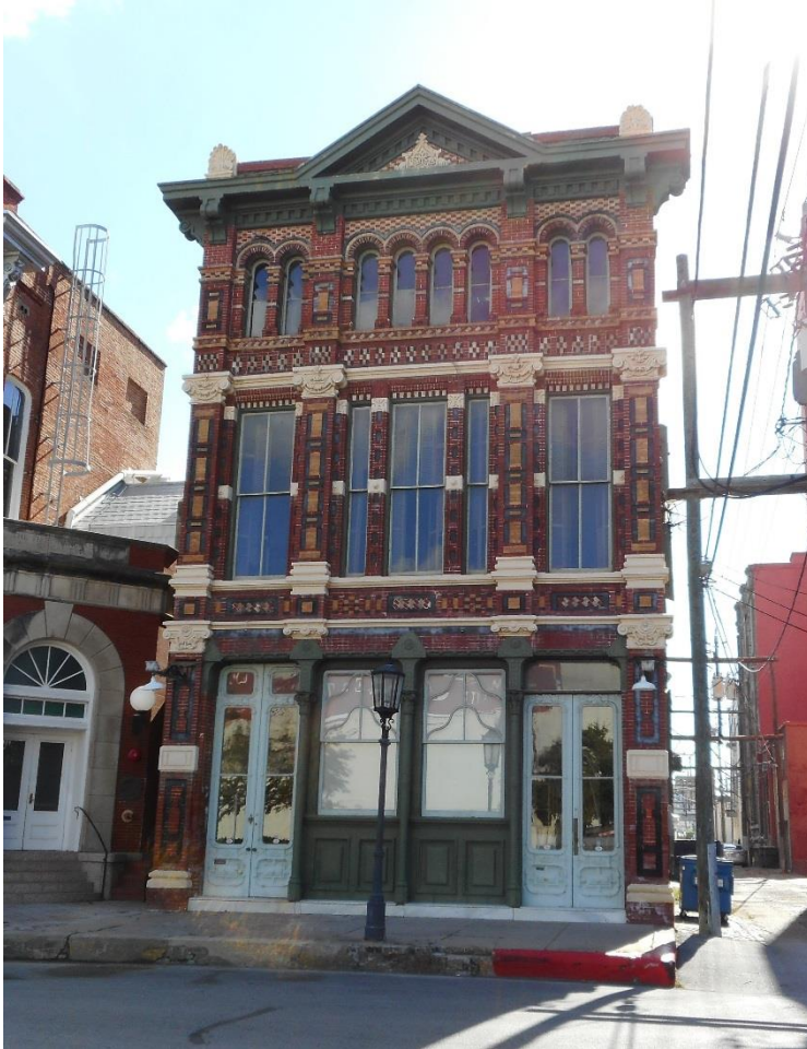
Photo 20 The Trueheart and Company Building at 212 22 nd Street, looking east.
