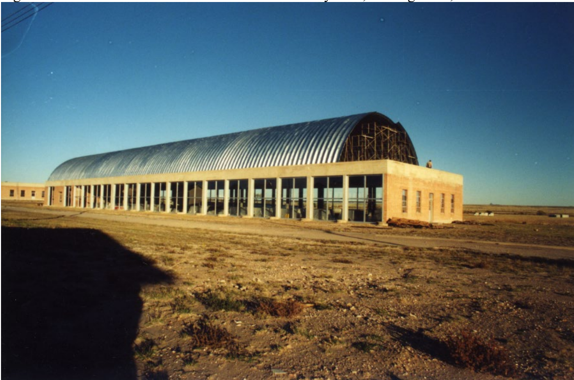
Figure 20: Barrel vault installation on the south artillery shed, looking north, 1984.
