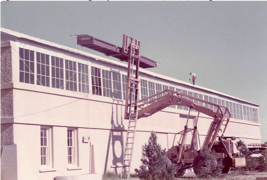
Figure 16: Contractors installing roof panels on the Arena, c. 1981, looking west.
