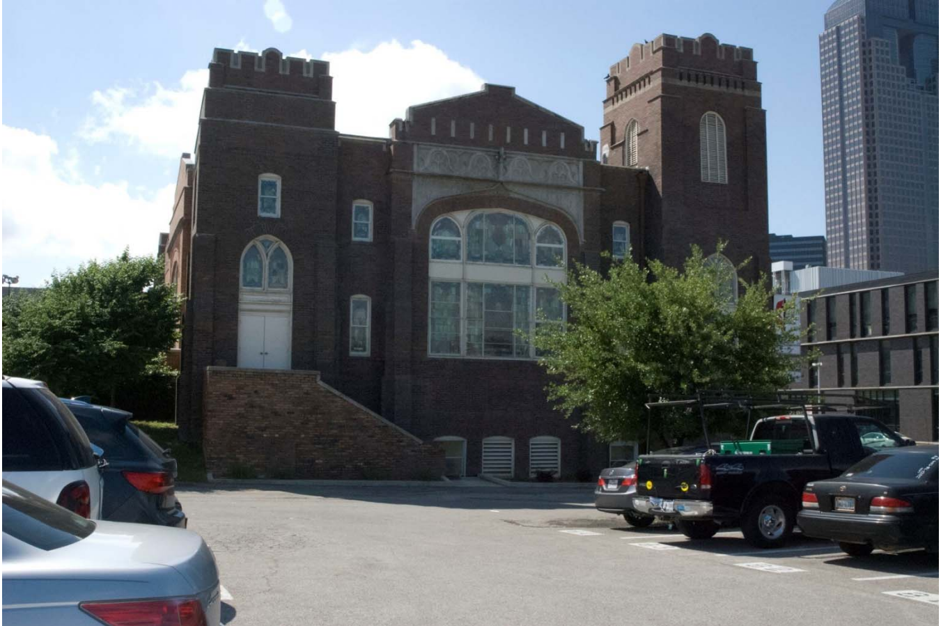
Photo 5: Side (Northwest) Elevation, camera facing southeast.
