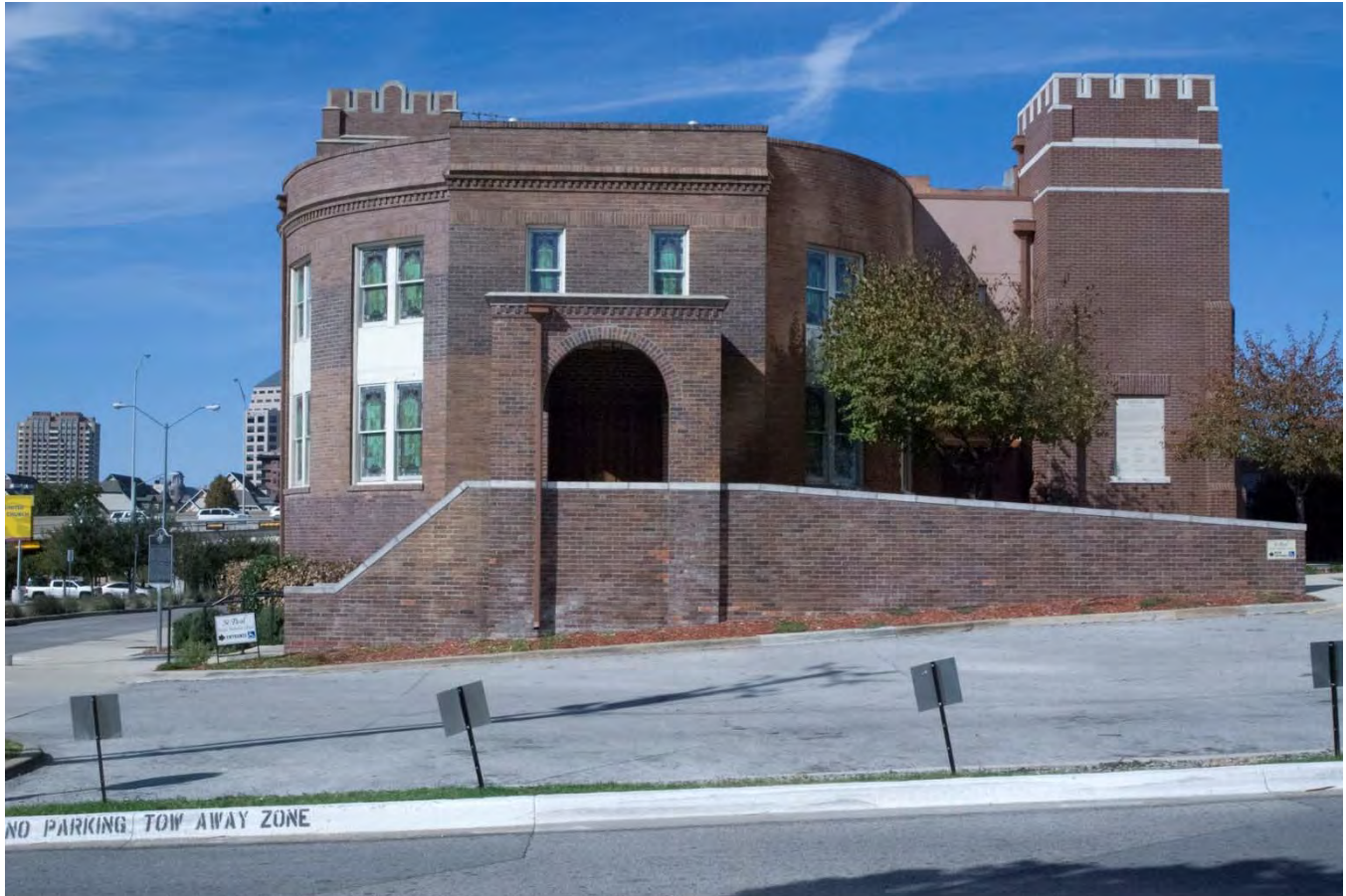
Photo 11: Side (Southeast) Elevation and Church Parking Lot, camera facing northwest.
