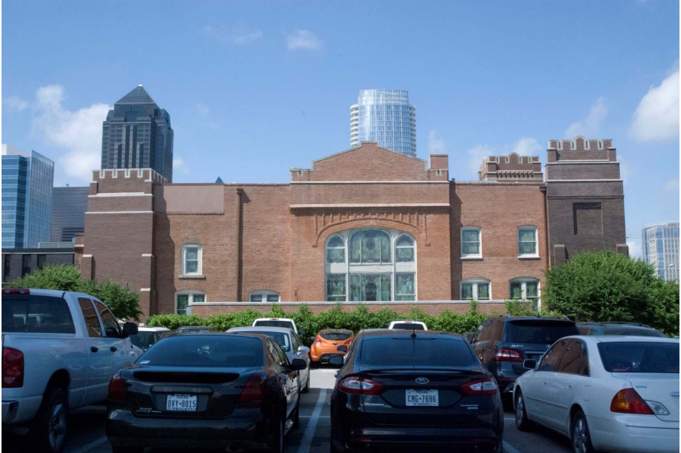
Photo 4: Rear (Northeast) Elevation, camera facing southwest.
