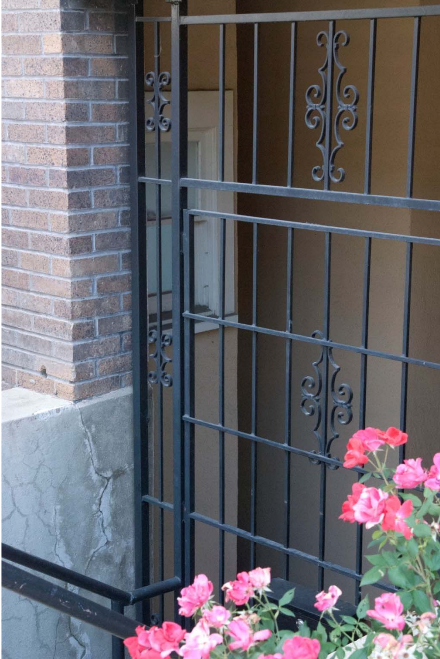
Photo 9: Front (Southwest) Elevation, Detail, Basement Door with Window, camera facing north.
