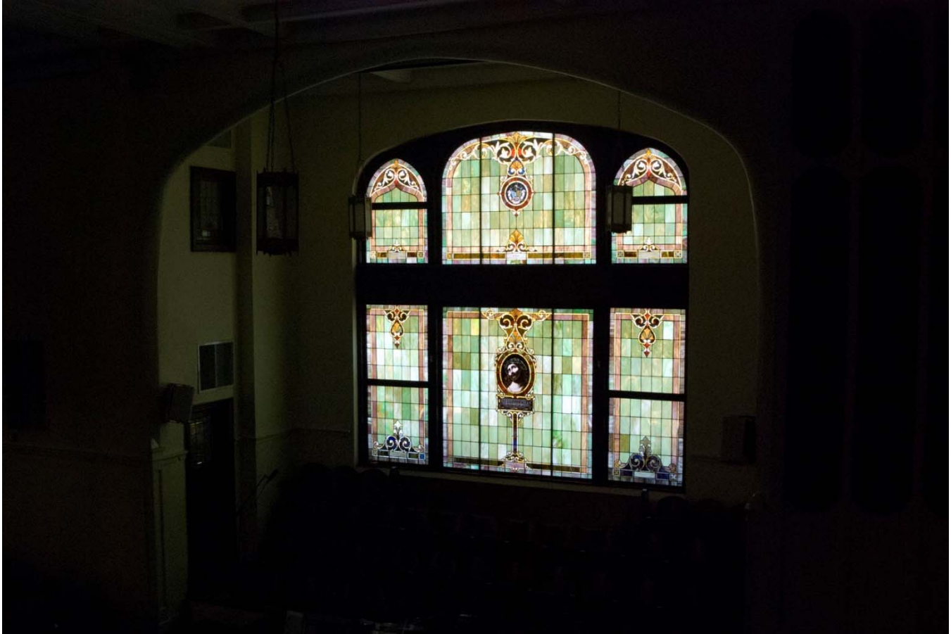
Photo 17: Interior View, Northeast Sanctuary Wall, Stained Glass Window, camera facing northwest.
