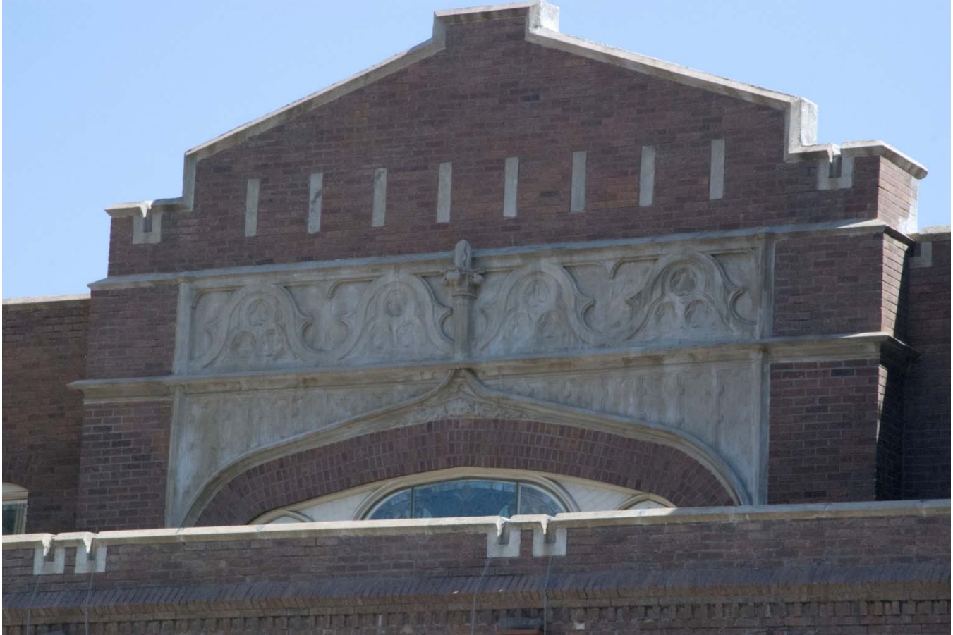
Photo 3: Front (Southwest) Elevation, Detail, Gable, camera facing north.
