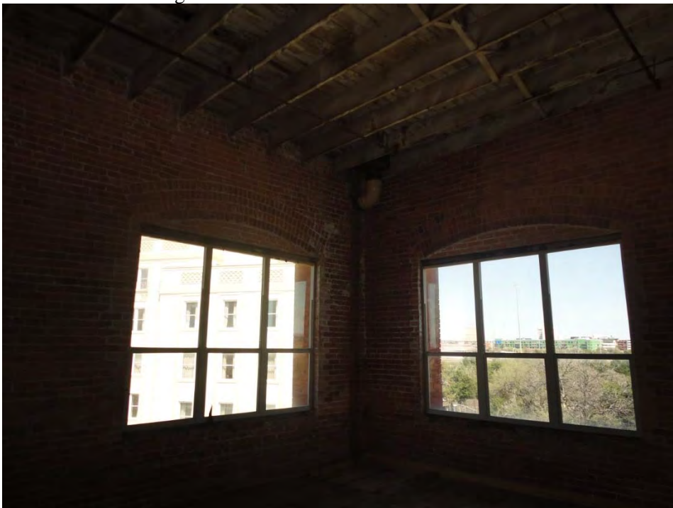
Photo 16 Floor 5 camera facing northeast corner
