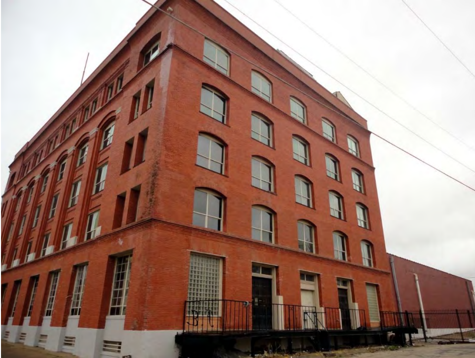
Photo 3 North and west facades
