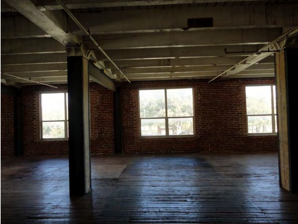
Photo 11 Floor 2 camera facing east
