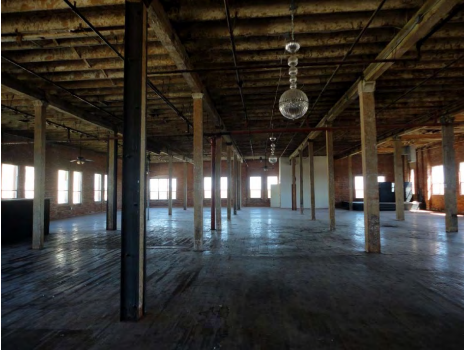
Photo 15 Floor 5 camera facing east
