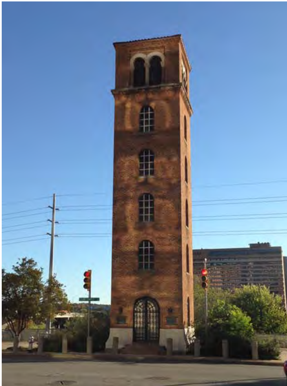
Photo 1: North façade. Camera facing south.
