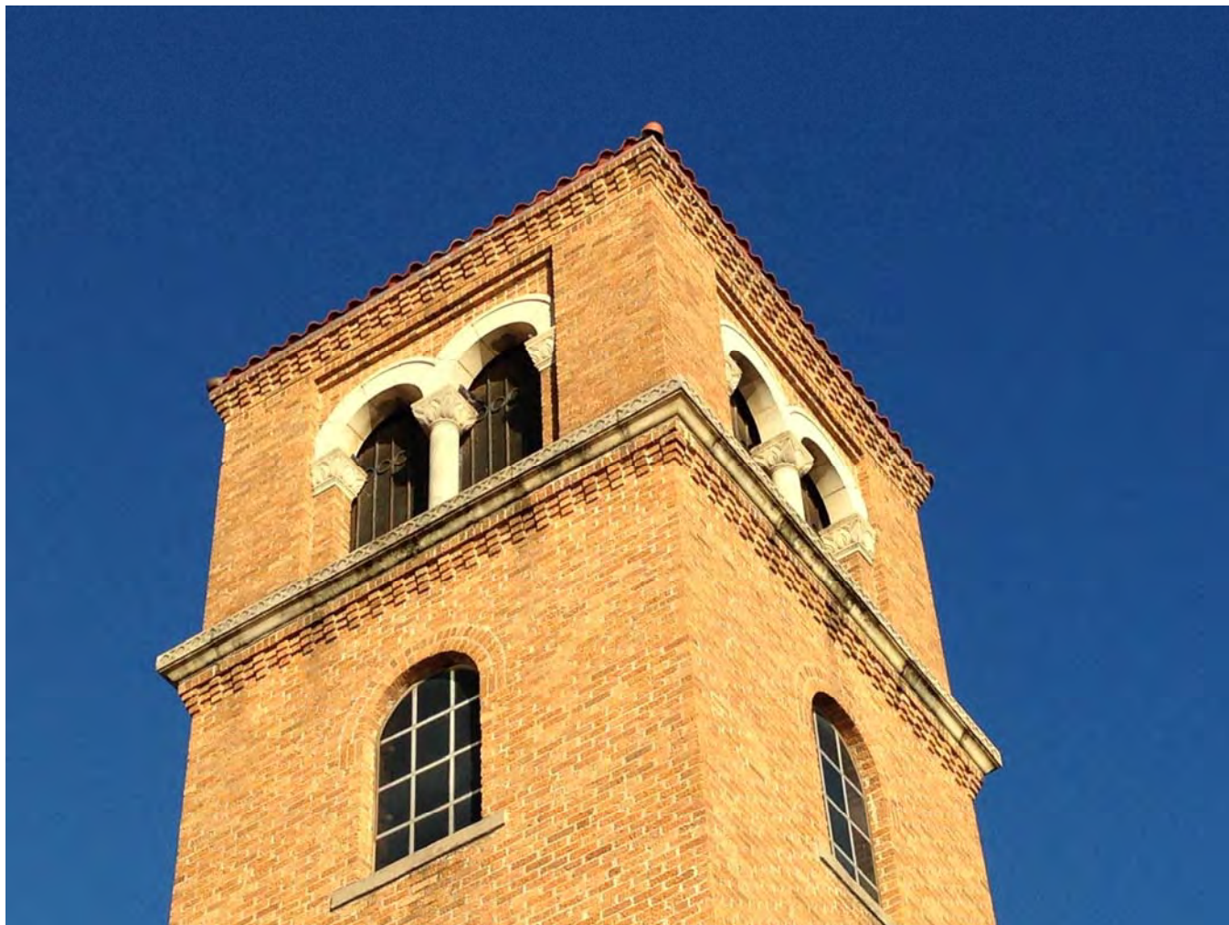
Photo 11: Detail, fifth and sixth floors.
