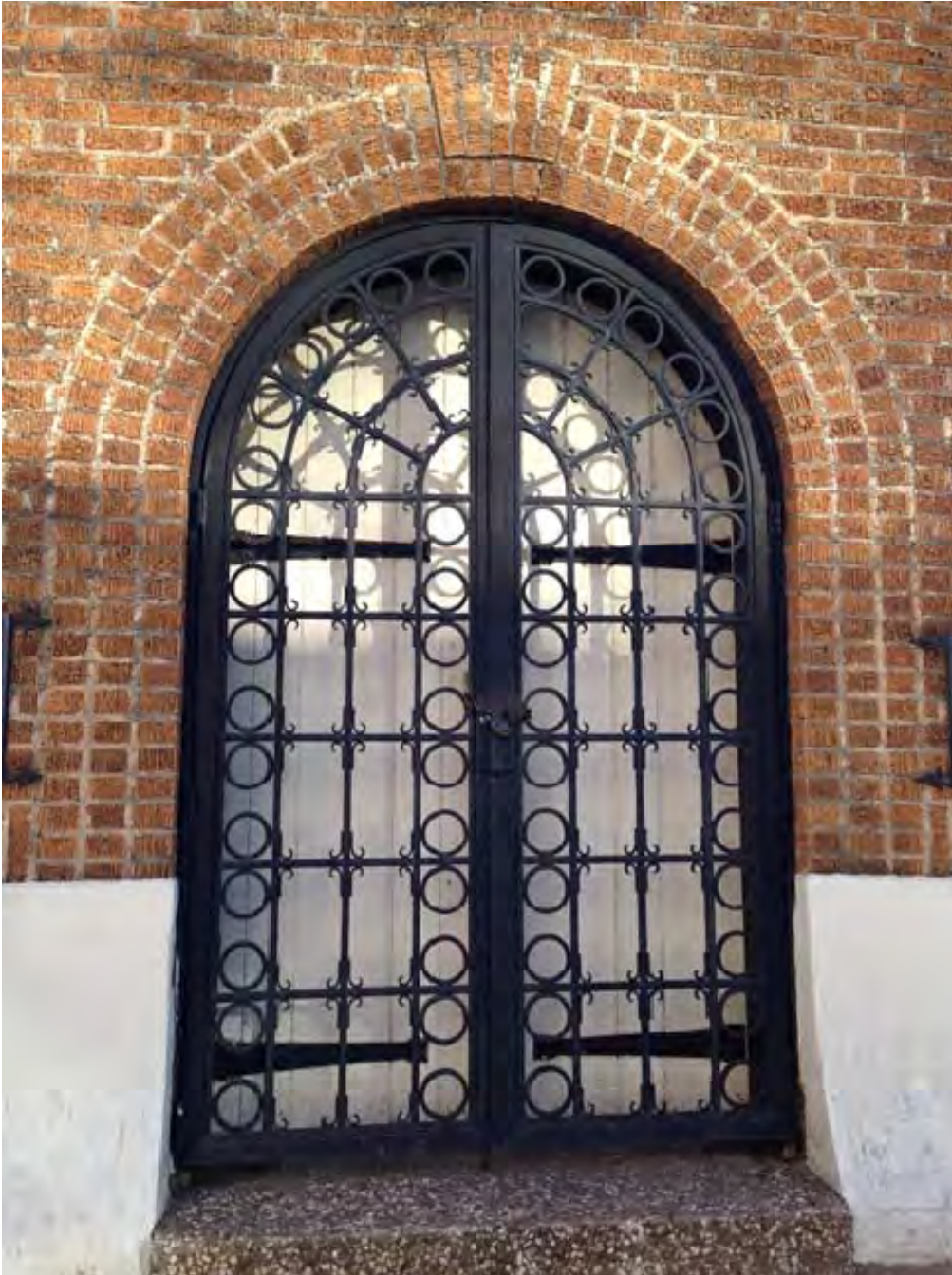
Photo 6: North elevation, door grill detail. Camera facing south.
