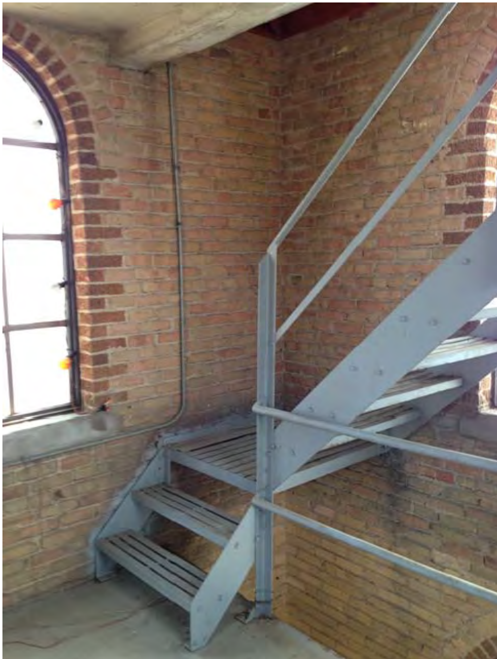
Photo 8: Fourth floor interior steel staircase. Camera facing southeast.
