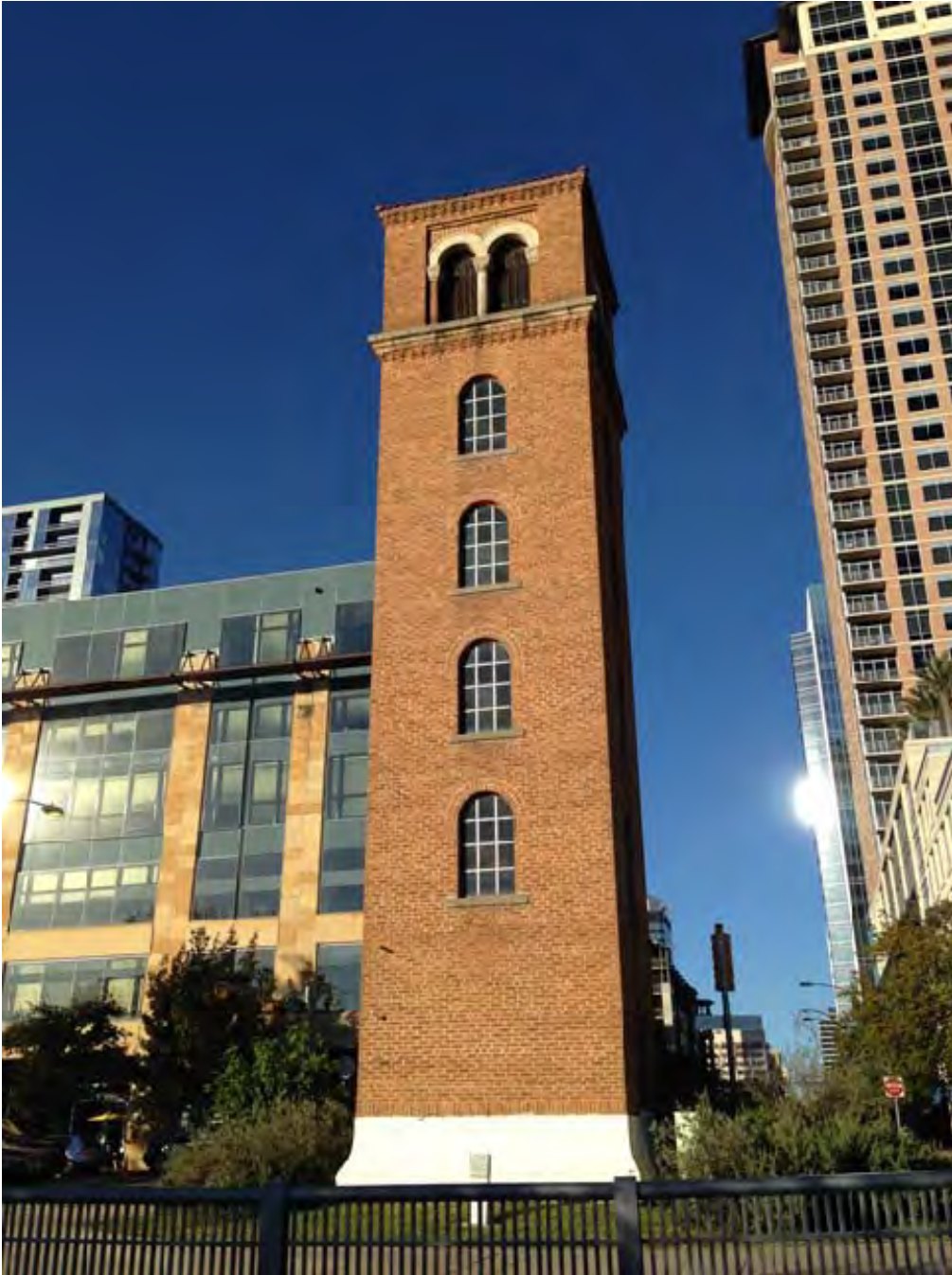
Photo 3: South façade. Camera facing north.
