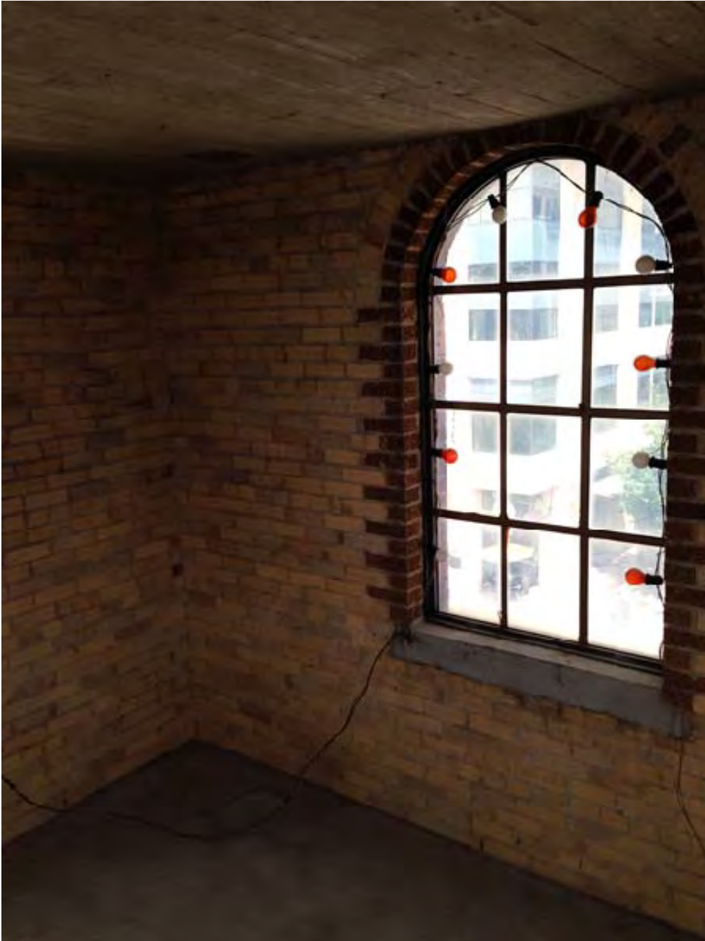
Photo 9: Third floor window. Camera facing northwest.
