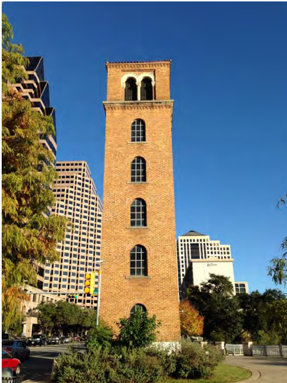
Photo 2: West façade. Camera facing east.
