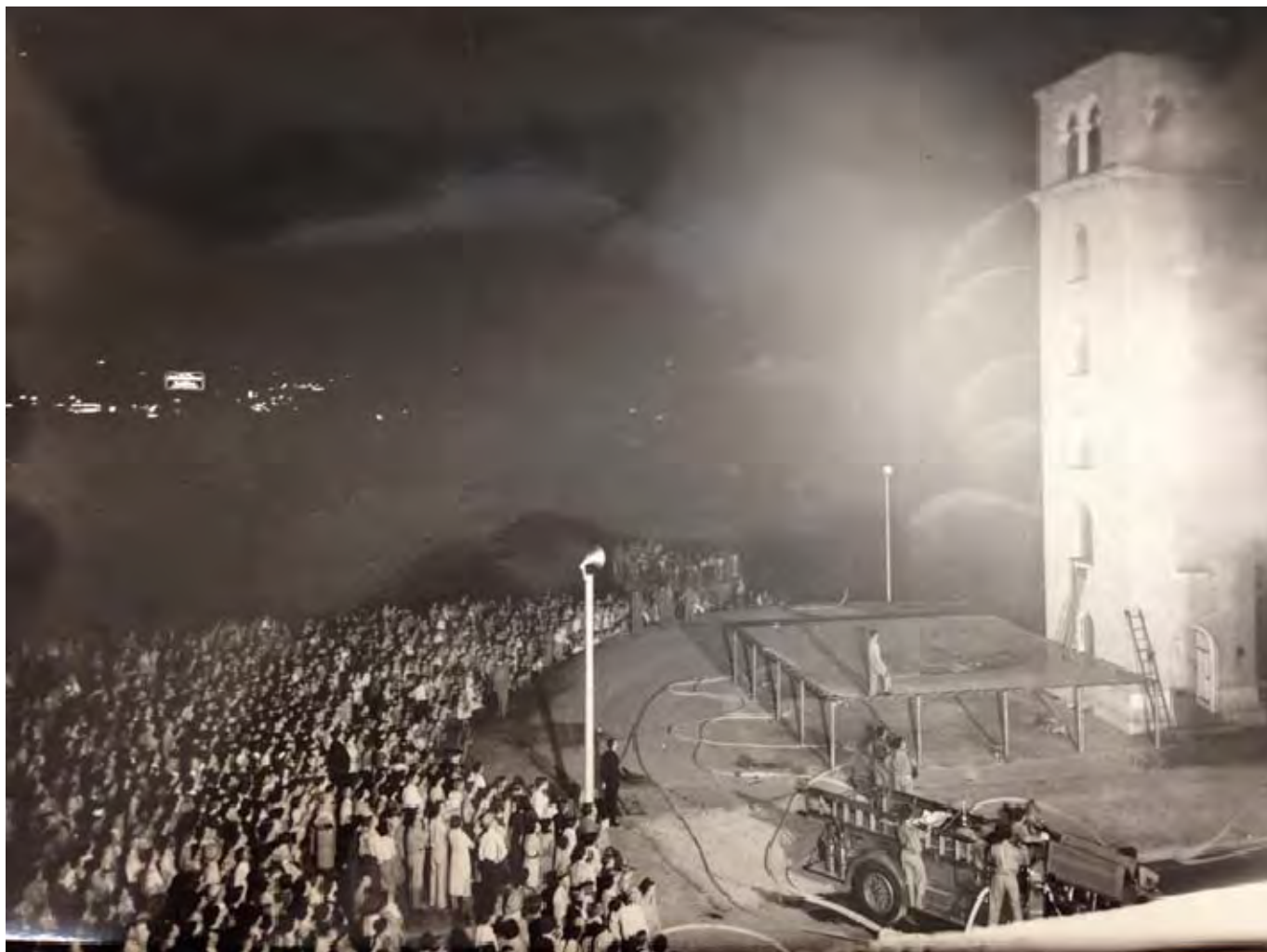
Figure 7: The Fire Drill Tower in action (1937). Courtesy Austin Fire Museum.
