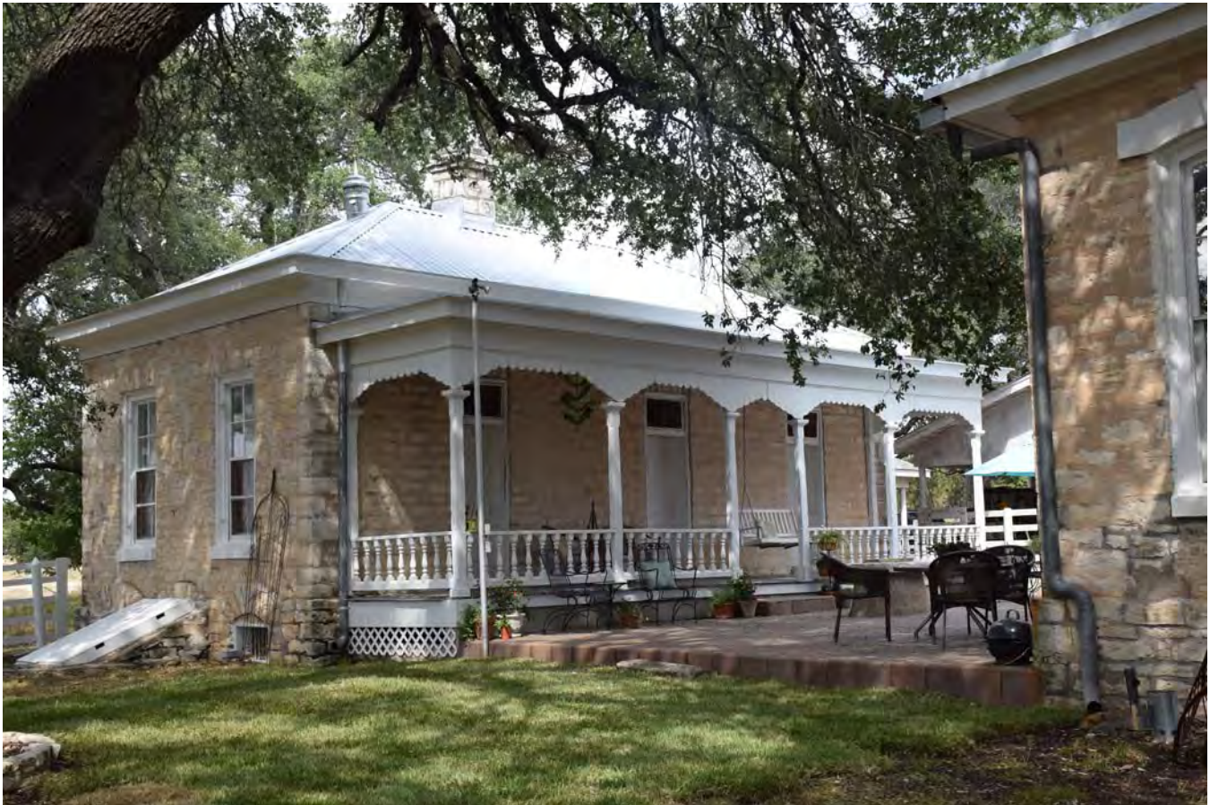
Photo 11 1875 House, south oblique Camera facing north/northeast
