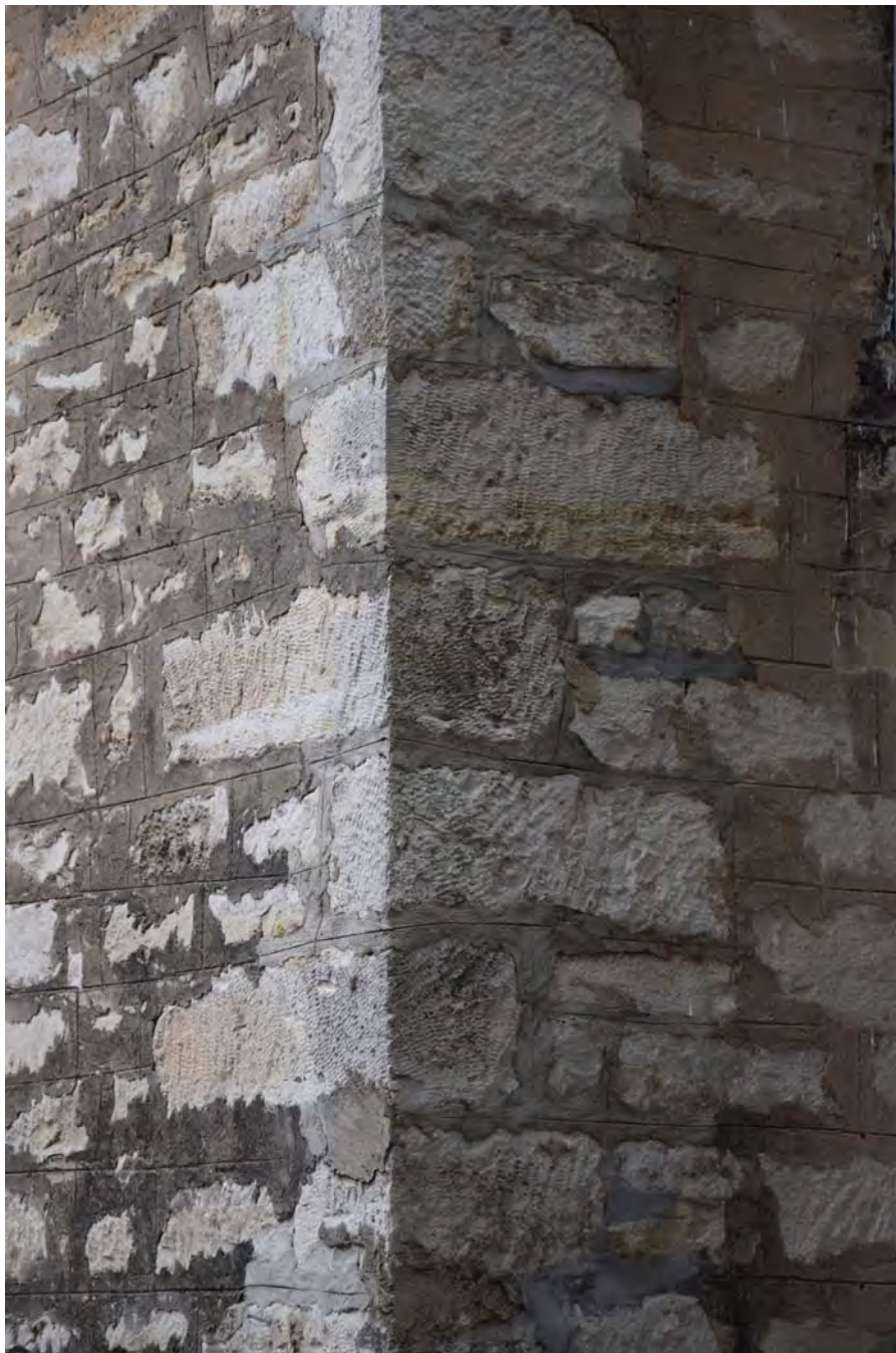
Photo 5 Main house, northwest corner showing masonry quoining Camera facing
