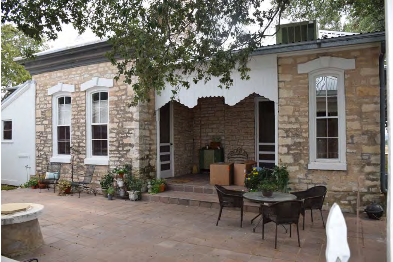
Photo 3 Main house, north oblique Camera facing south/southeast
