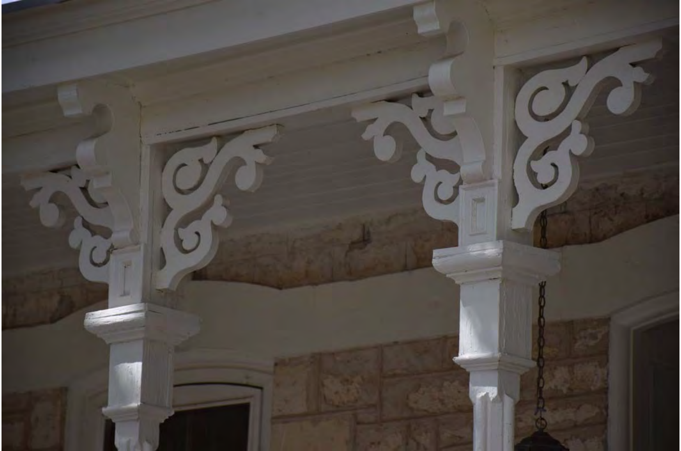
Photo 6 Main house, south elevation porch detail Camera facing north
