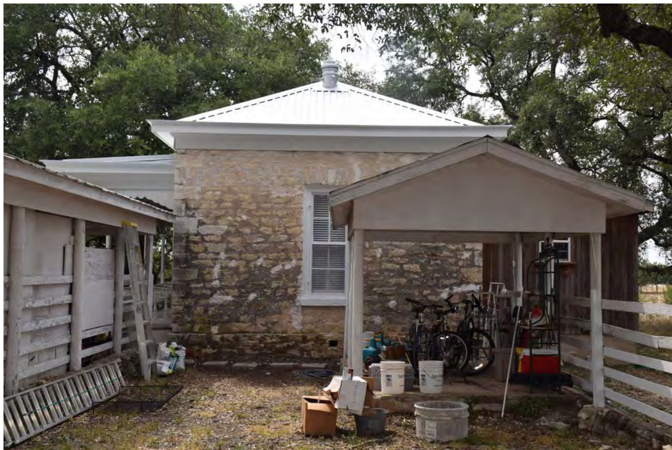
Photo 13 Open storage shed (noncontributing) Camera facing west
