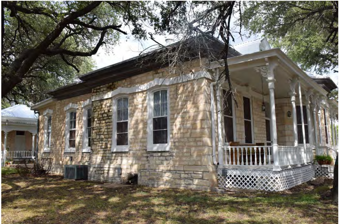
Photo 2 Main house, west oblique Camera facing northeast
