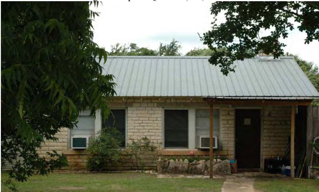
Photo 28: Camera facing S. Keeper's Quarters (#20) north elevation.
