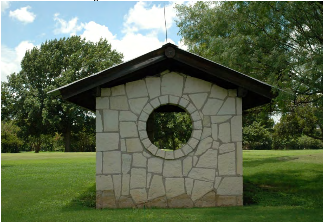
Photo 30: Camera Facing N. Limestone storm shelter (#22) between 3 rd tees and 8 th tees. South elevation.
