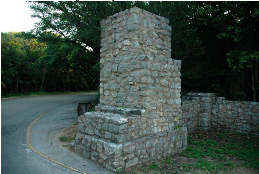
Photo 34: Camera facing SW. Entry Piers (#25).
