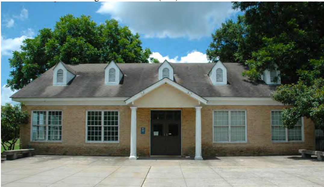
Photo 26: Camera facing S. Clubhouse (#19) north elevation.
