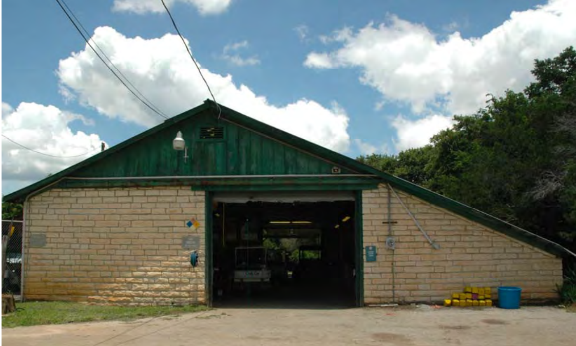
Photo 29: Camera facing N. Maintenance Building (#21) south elevation.
