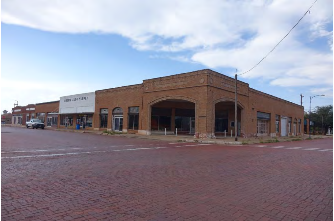
Photo 4 Avenue D at Main, facing northwest
