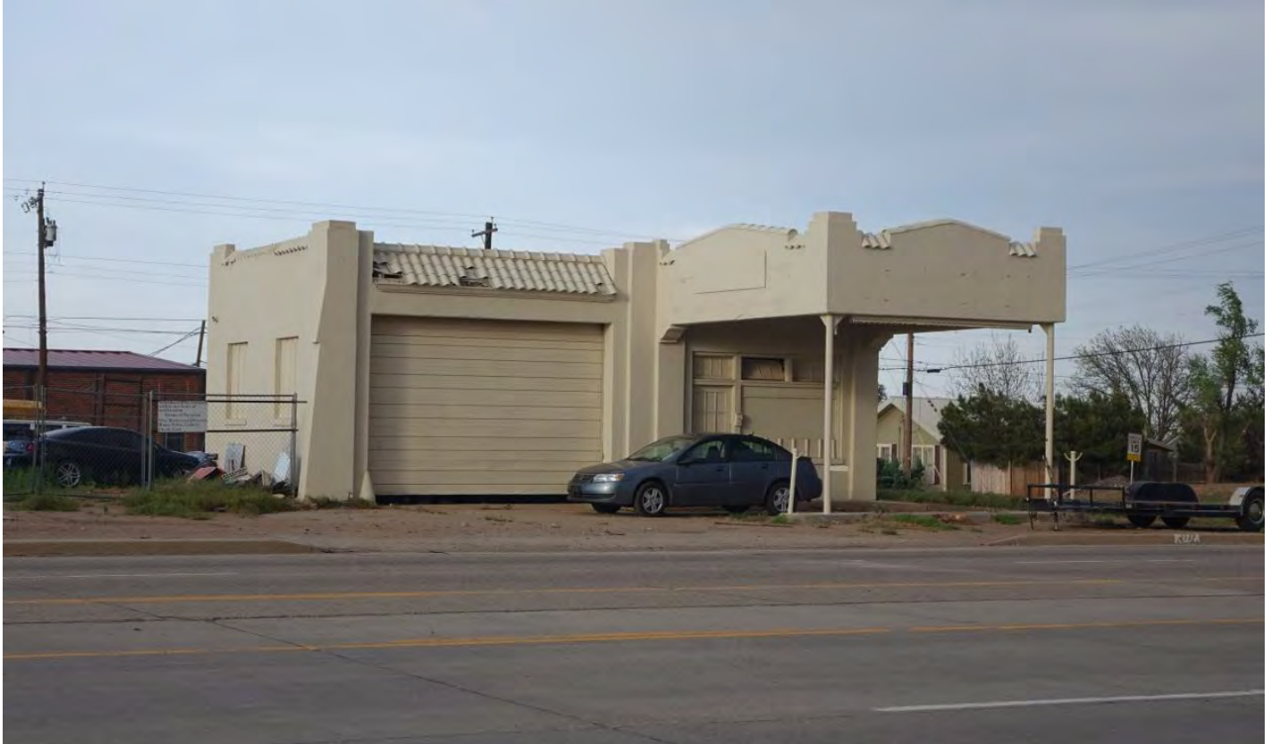
Photo 15 100 Avenue F NW (#66)
