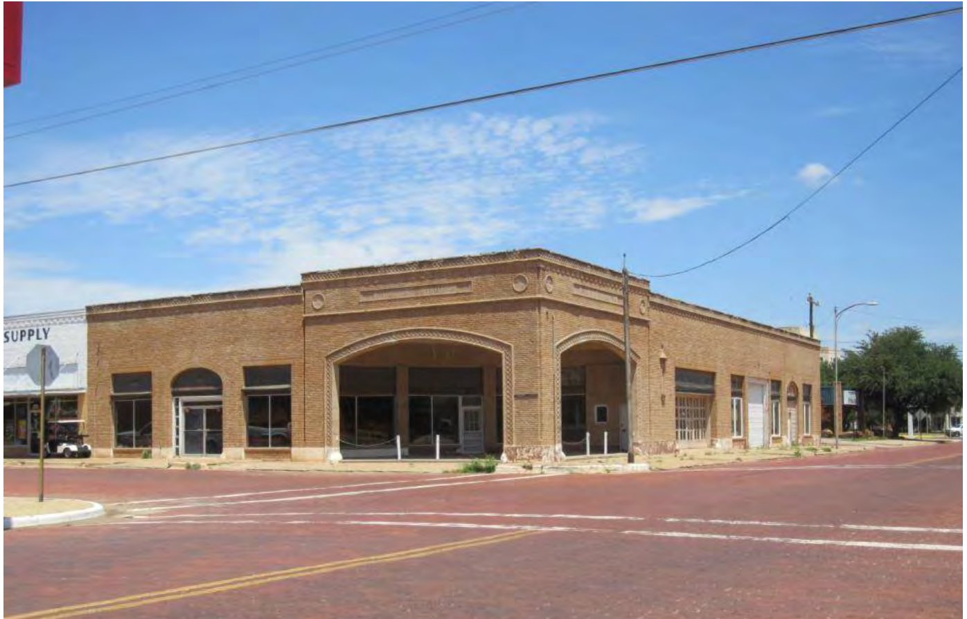
Photo 20 Michie Building, 401 Main (#123)
