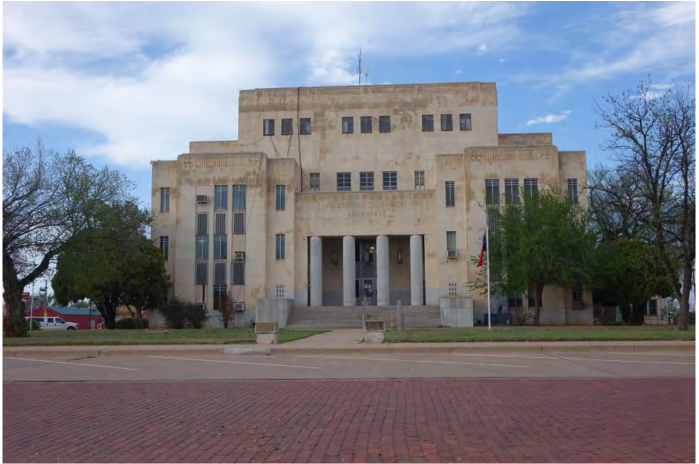
Photo 14 Childress County Courthouse, 100 Avenue E NW (#63)
