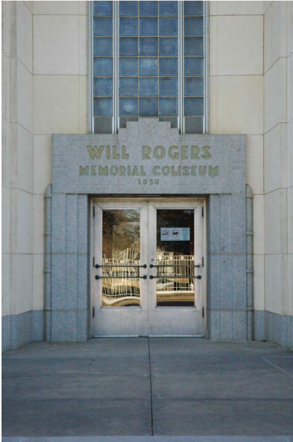
Photo 5 Will Rogers Coliseum entry door, from west side, north end
