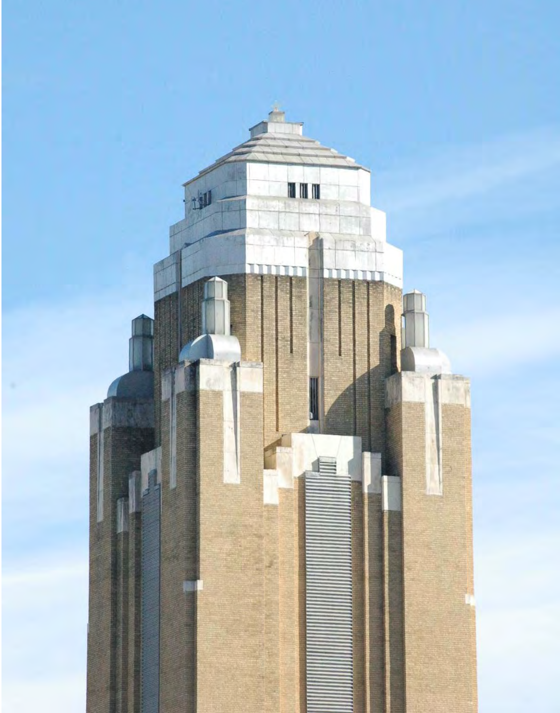
Photo 2 Tower detail Camera facing east
