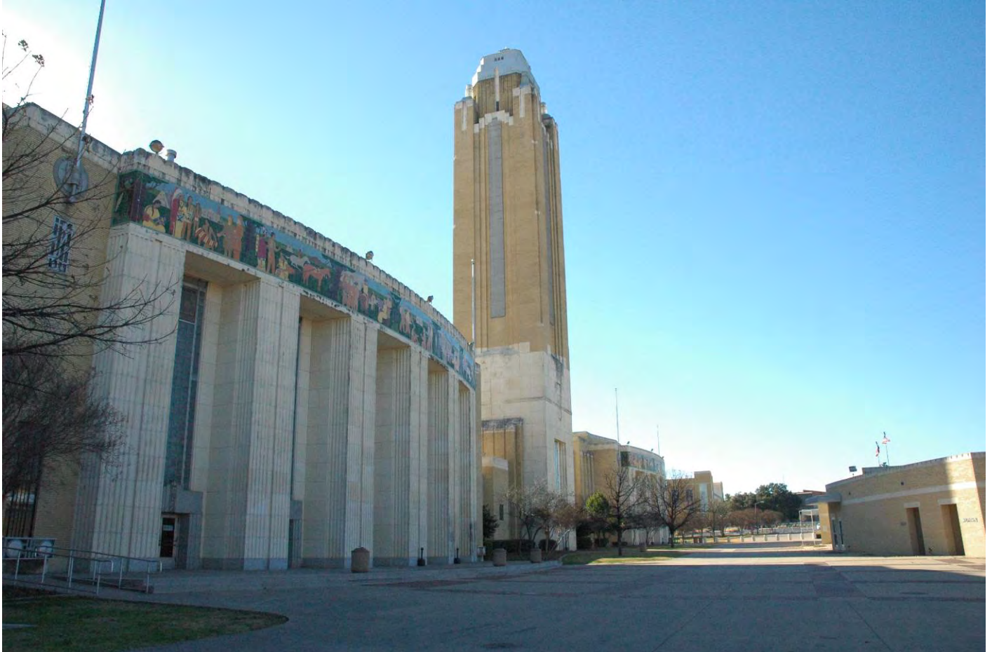
Photo 4 Will Rogers Coliseum and Tower From entry plaza on north side corner
