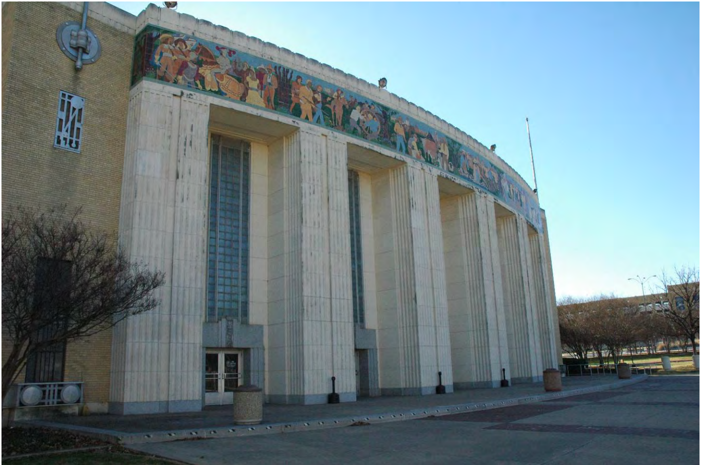
Photo 3 Will Rogers Coliseum From entry plaza on north side corner
