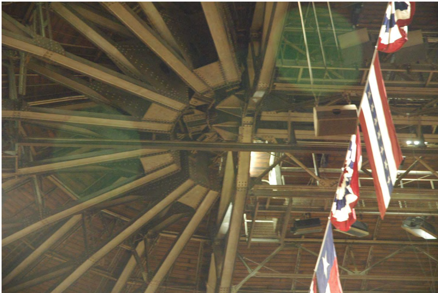
Photo 21 Coliseum looking up at doubled arch trusses at pivots for stability
