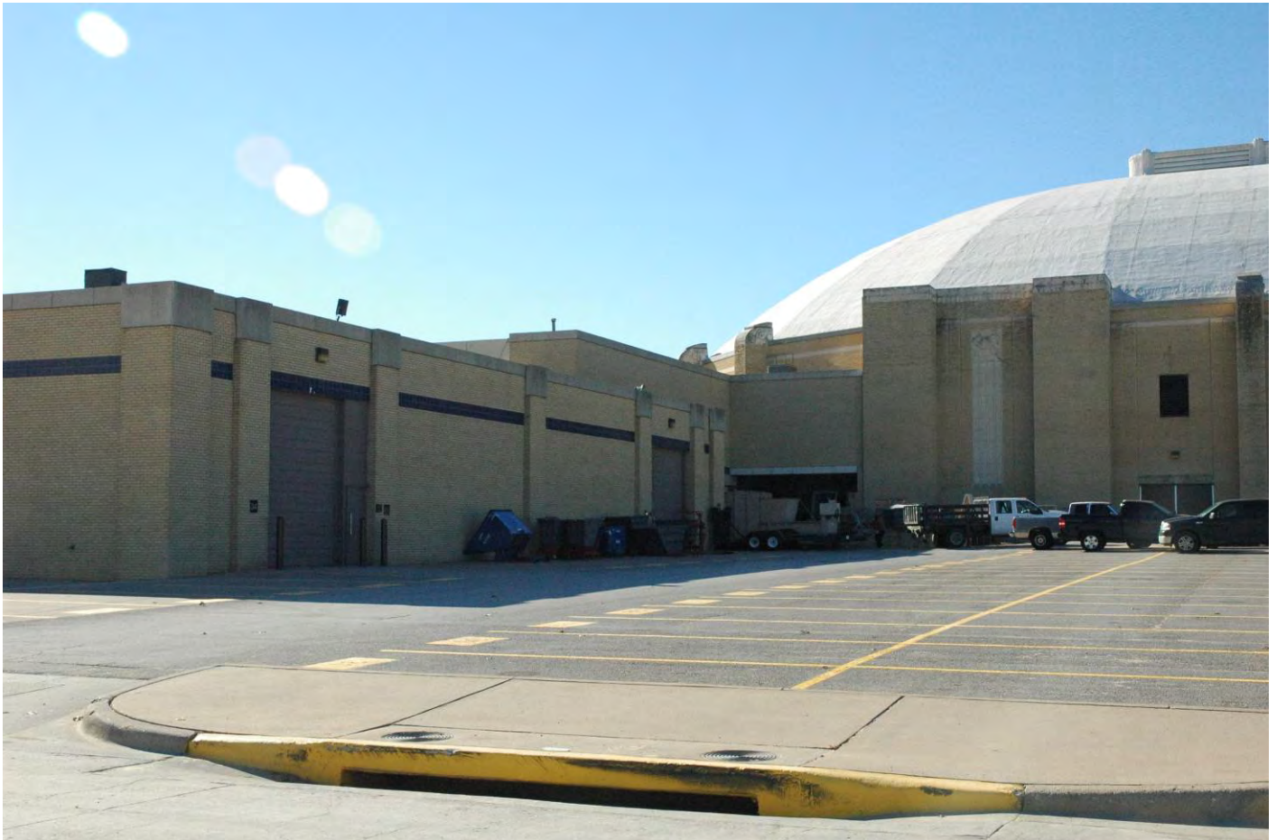
Photo 7 Will Rogers Coliseum at Burnett Building dock, looking southwest
