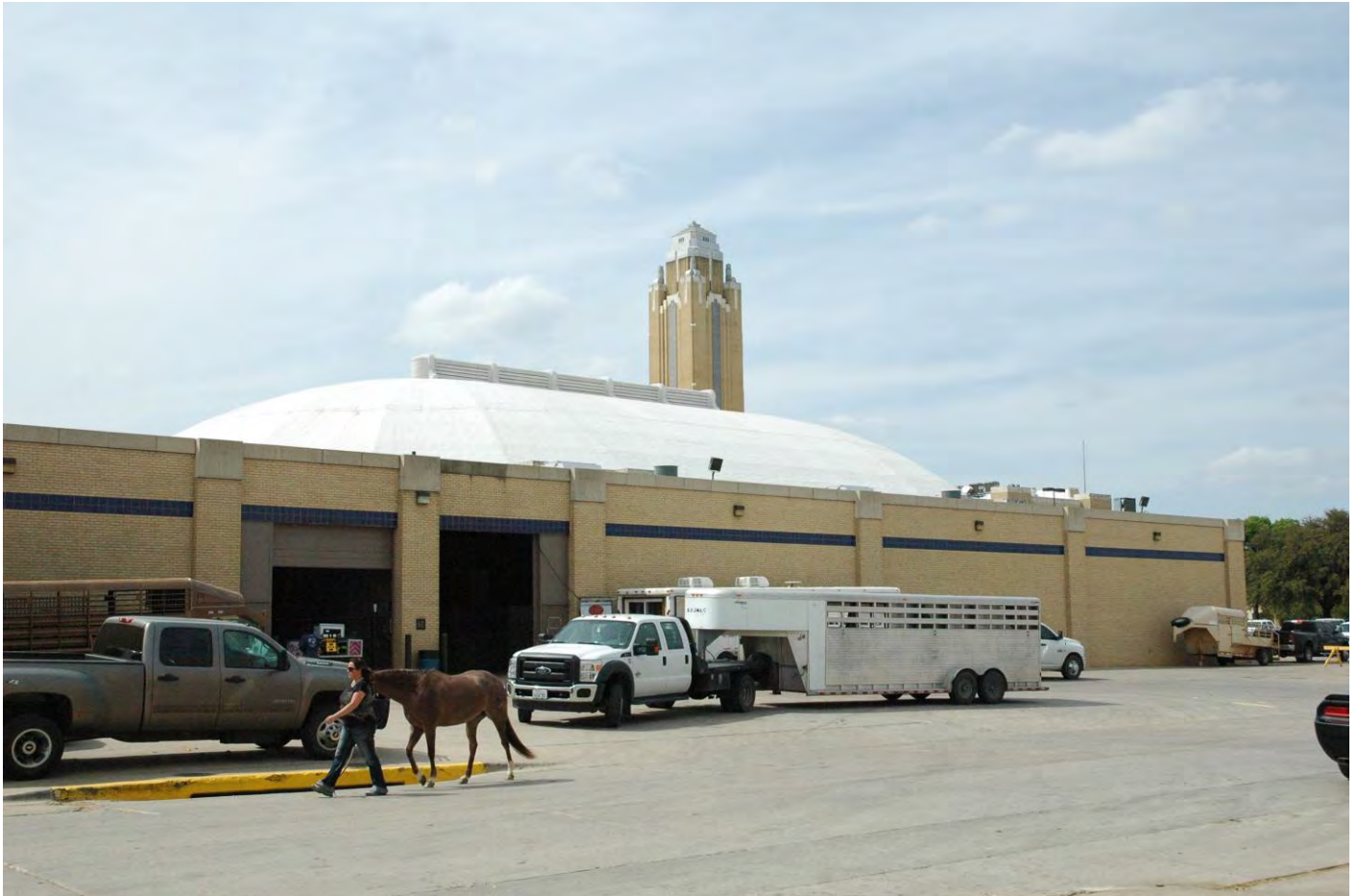
Burnett Building, looking northeast from Burnett-Tandy Drive (formerly Crestline Street)
