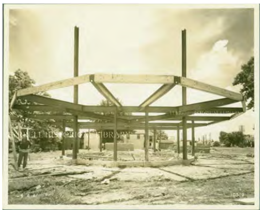
Figure 27. Pig Stand #41 steel framing by Dollinger Steel, Beaumont, Texas, c. 9/4/1941 (Dollinger Steel Company Archives at the Tyrrell Library)
