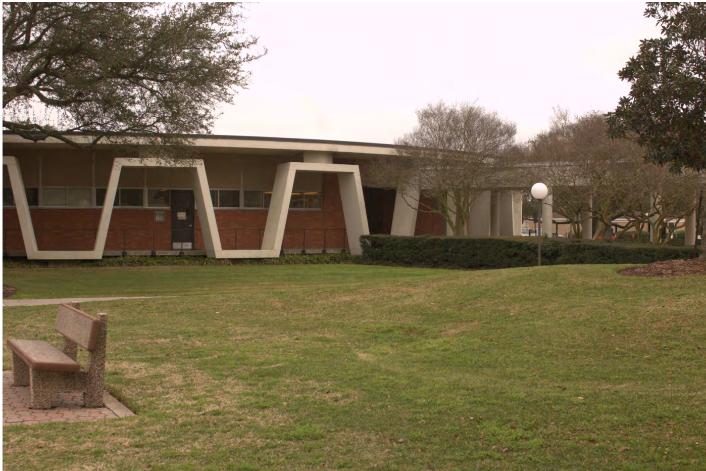
Photo 5 North side. Camera facing South.
