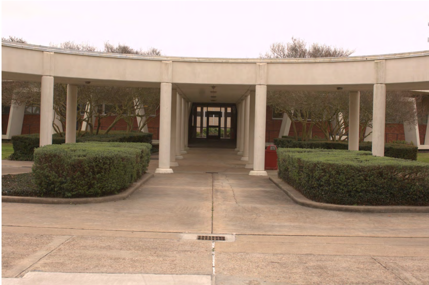
Photo 4 Northwest entrance. Camera facing Southeast.
