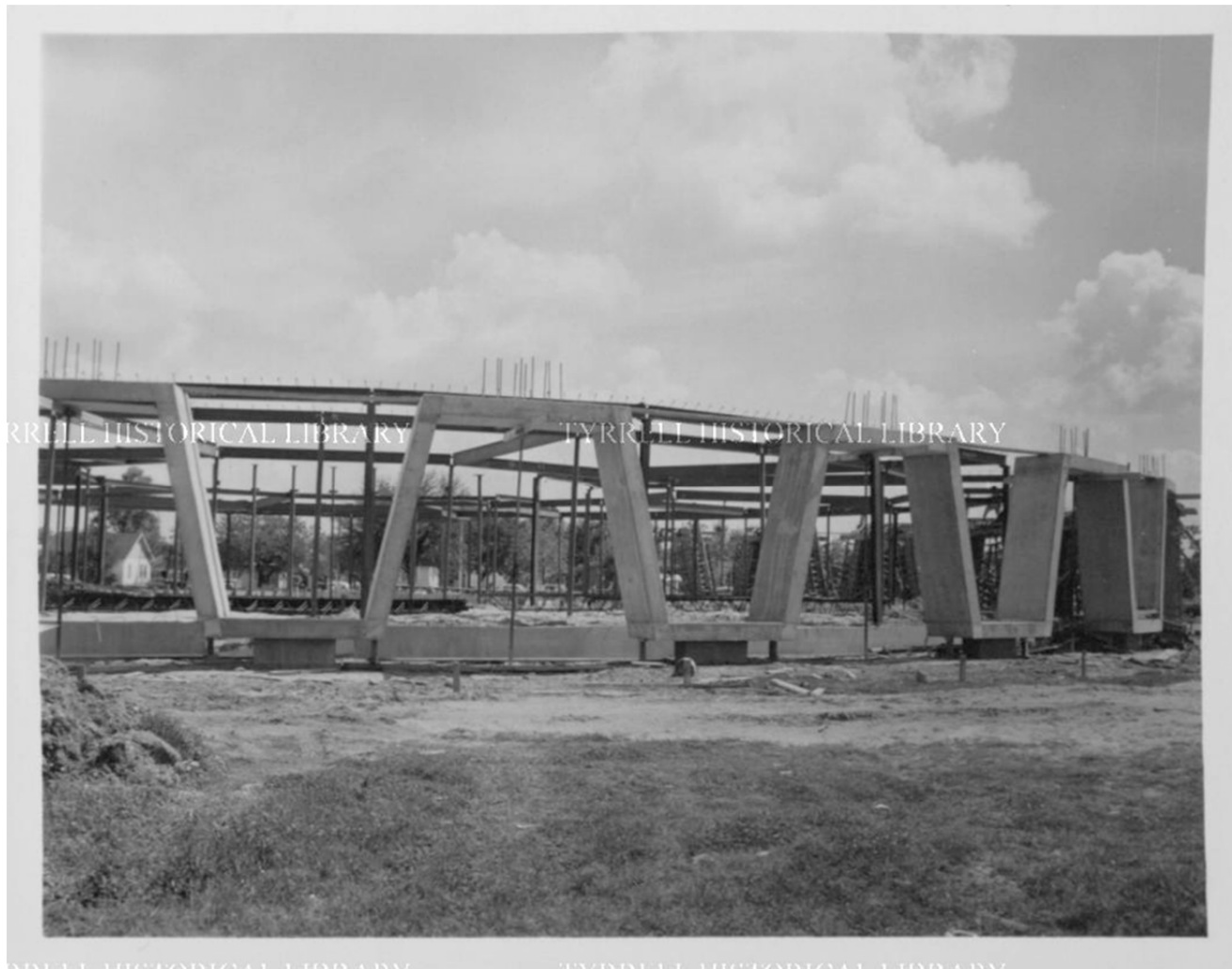
Figure 18. Construction photograph during steel framing, dated May 1959. Note exposed rebar for roof support casting. (Dollinger Steel Company Archives at the Tyrrell Library).
