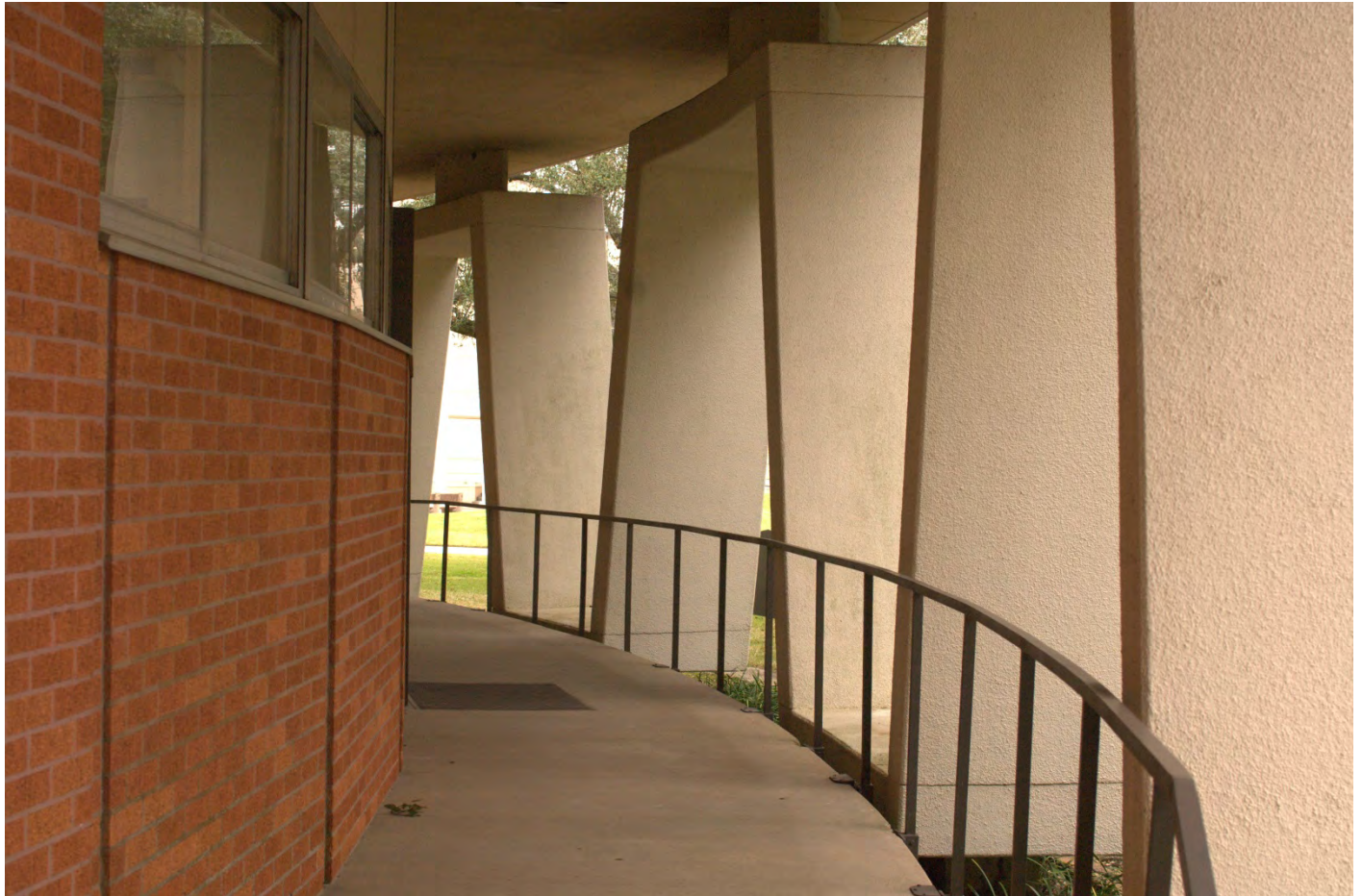
Photo 6 Exterior walkway, Northeast side. Camera facing Northwest.
