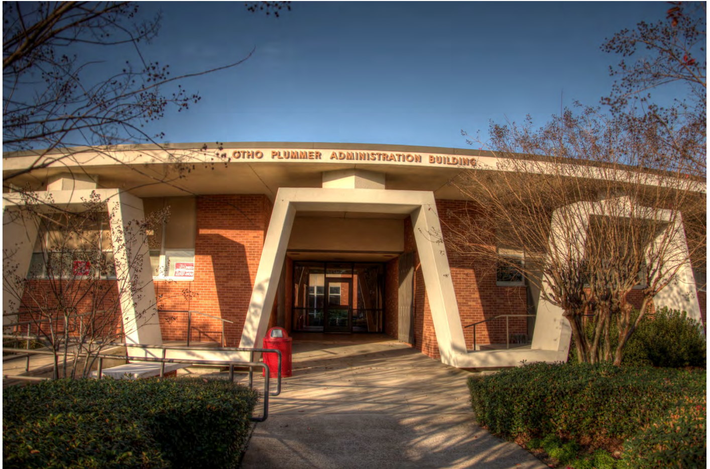
Photo 12 South Entrance. Camera facing North.
