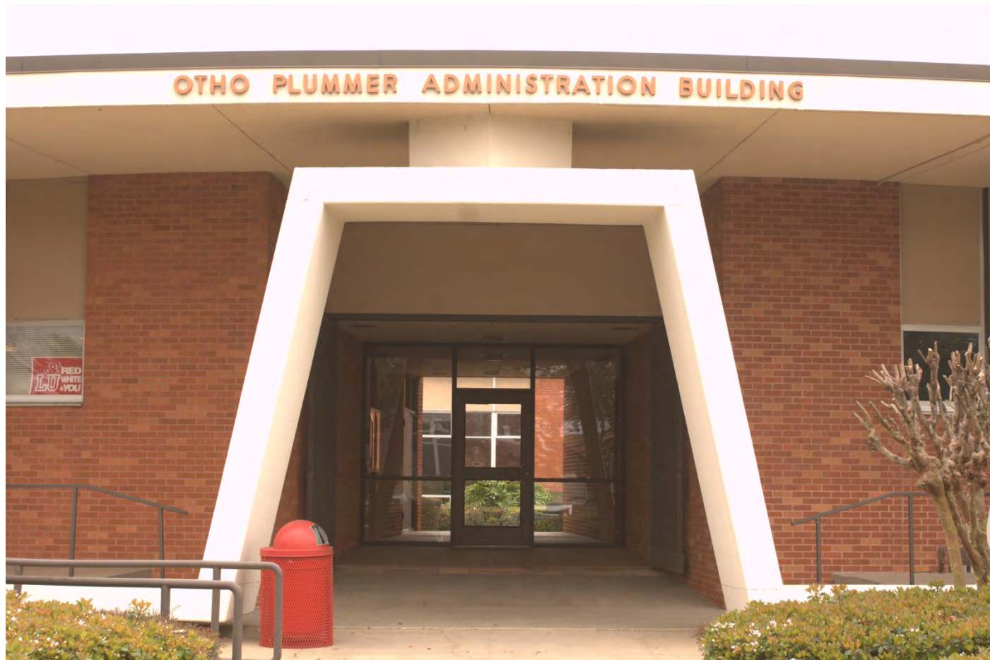
Photo 2 South entrance. Camera facing North.
