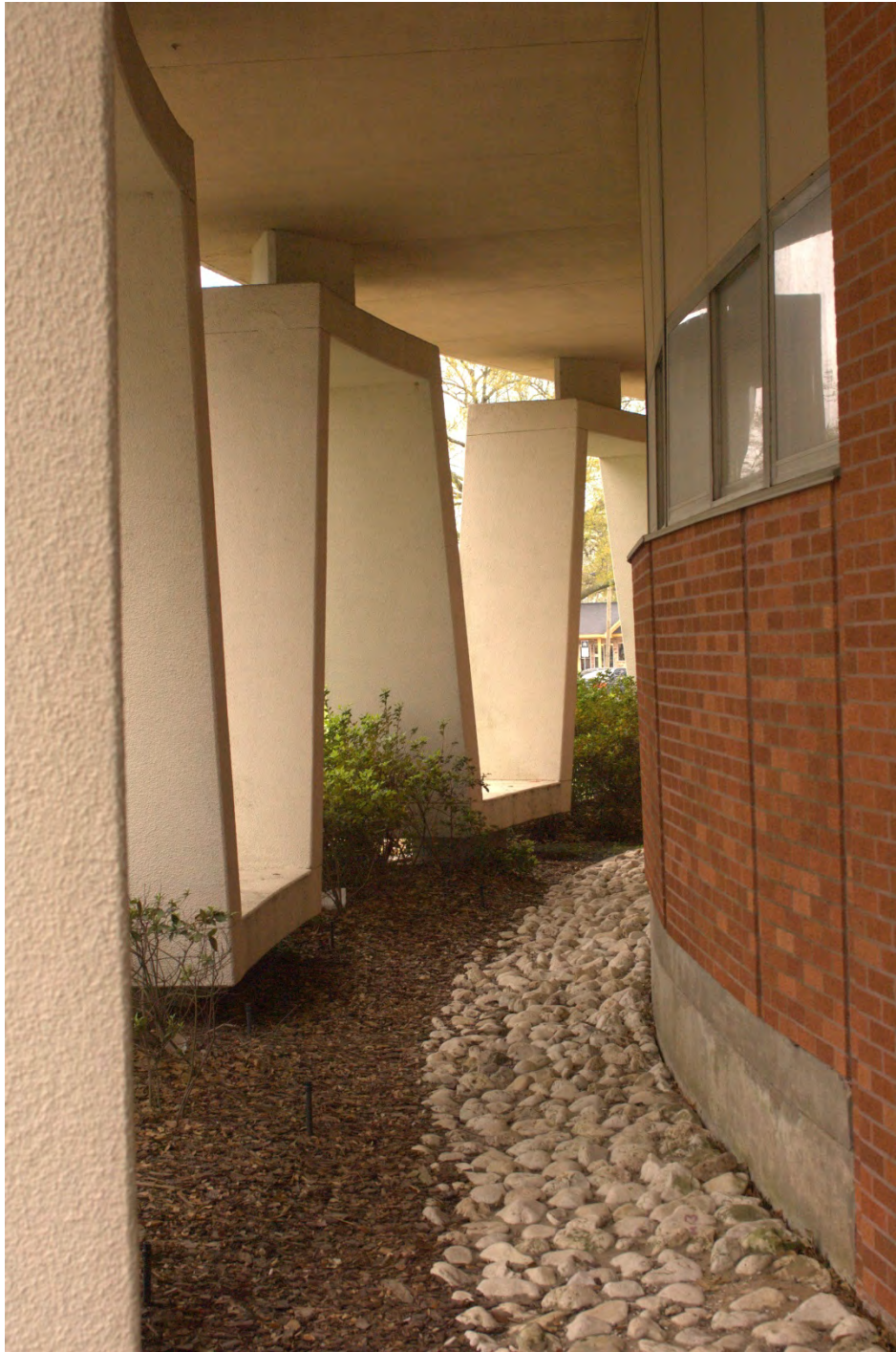
Photo 7 Eastside exterior detail. Camera facing south.
