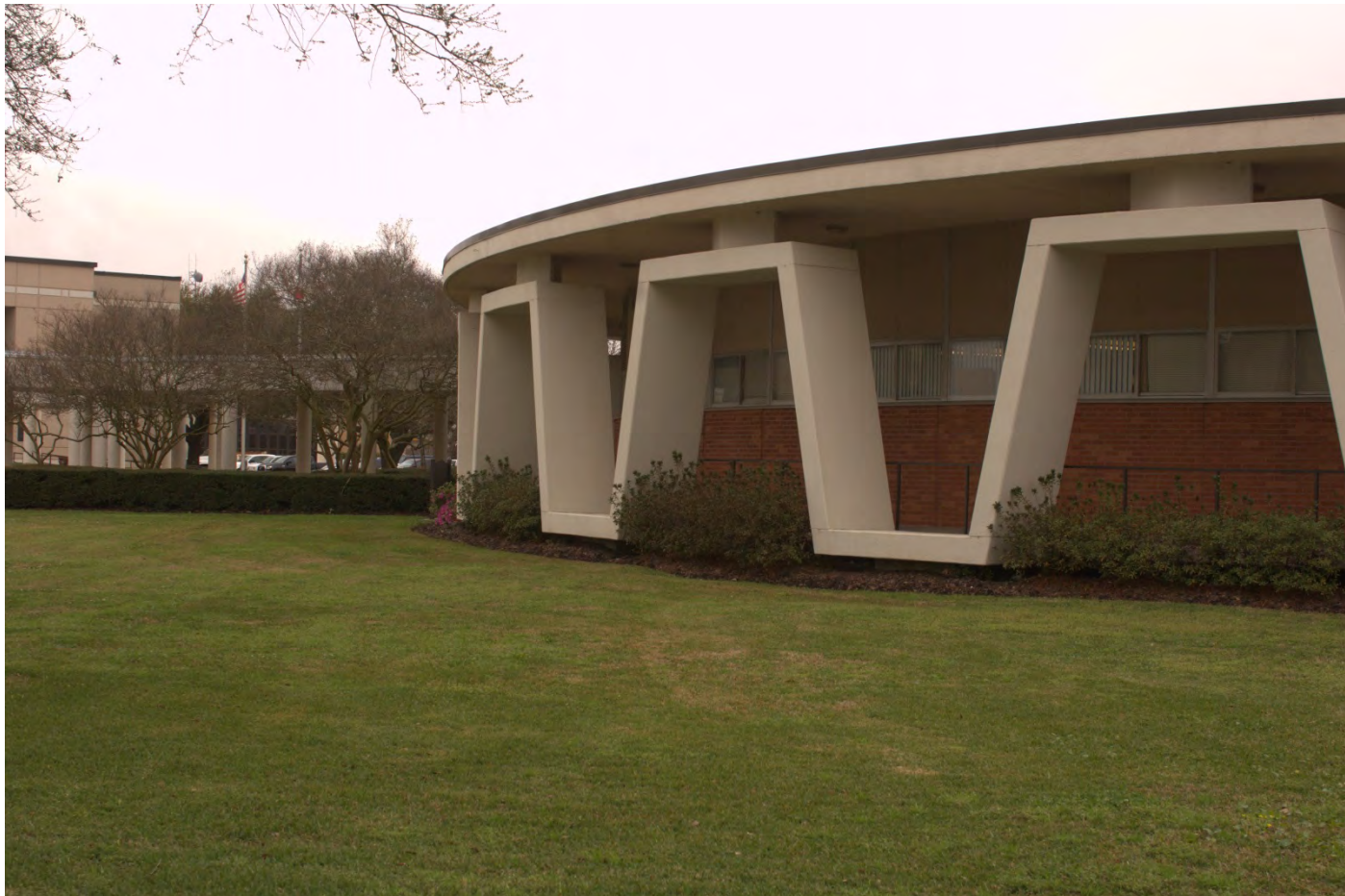
Photo 3 West side. Camera facing North.
