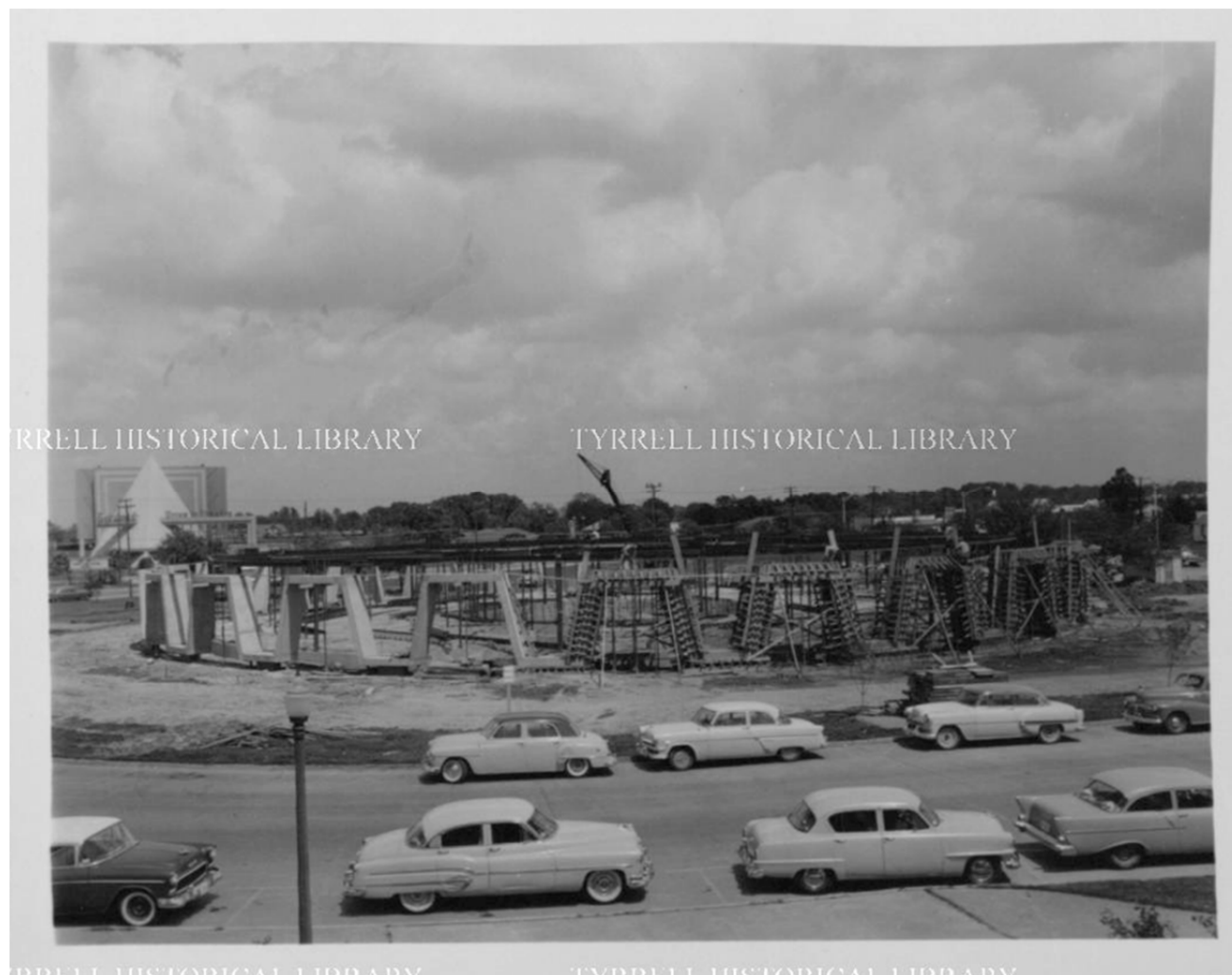
Figure 16. Construction photograph during steel framing, dated May 1959. Note on site concrete casting of perimeter "fret" band. Pyramid drive-in movie theater in background (Dollinger Steel Company Archives at the Tyrrell Library).
