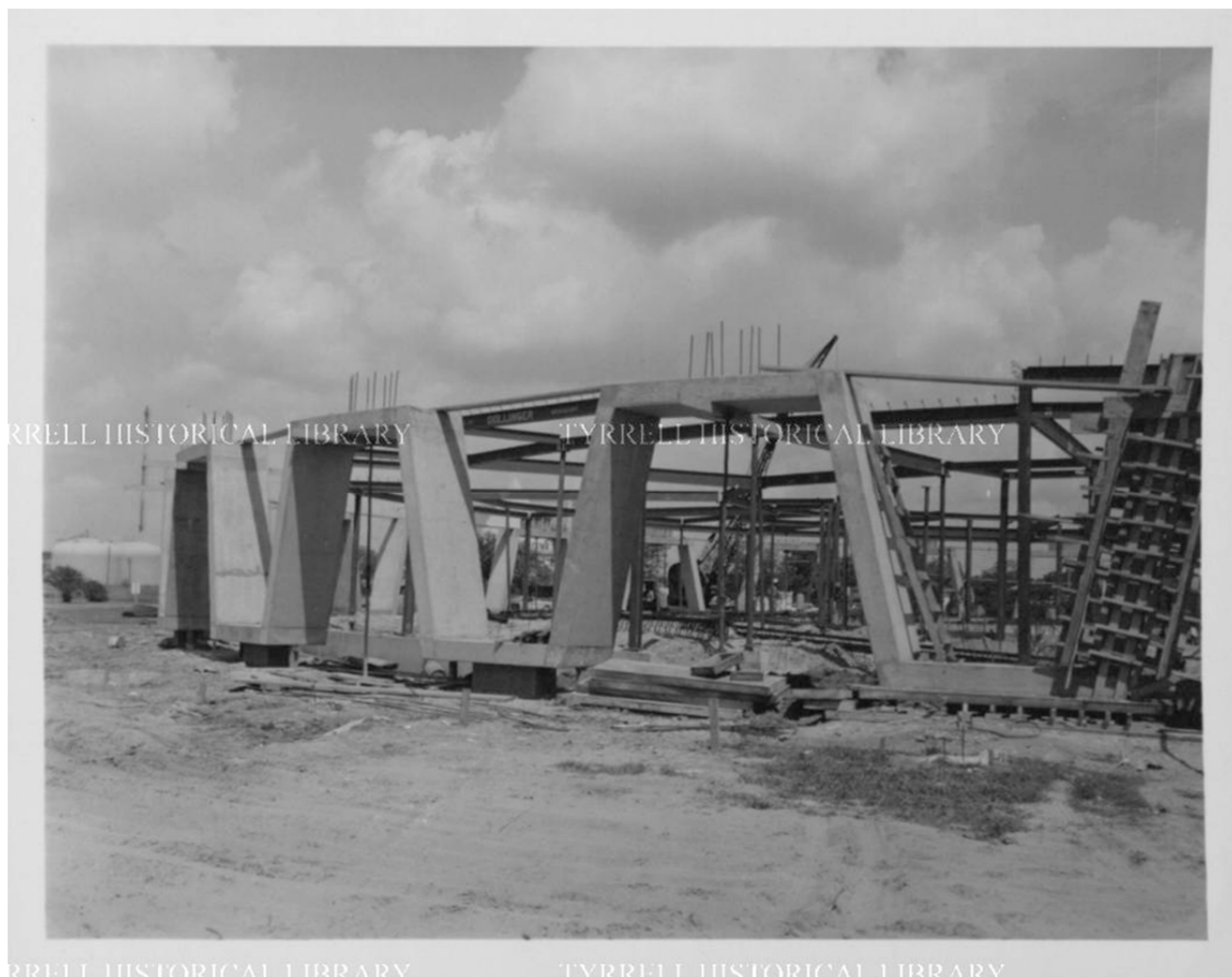
Figure 17. Construction photograph during steel framing, dated May 1959. Note on site concrete casting of perimeter "fret" band. (Dollinger Steel Company Archives at the Tyrrell Library).
