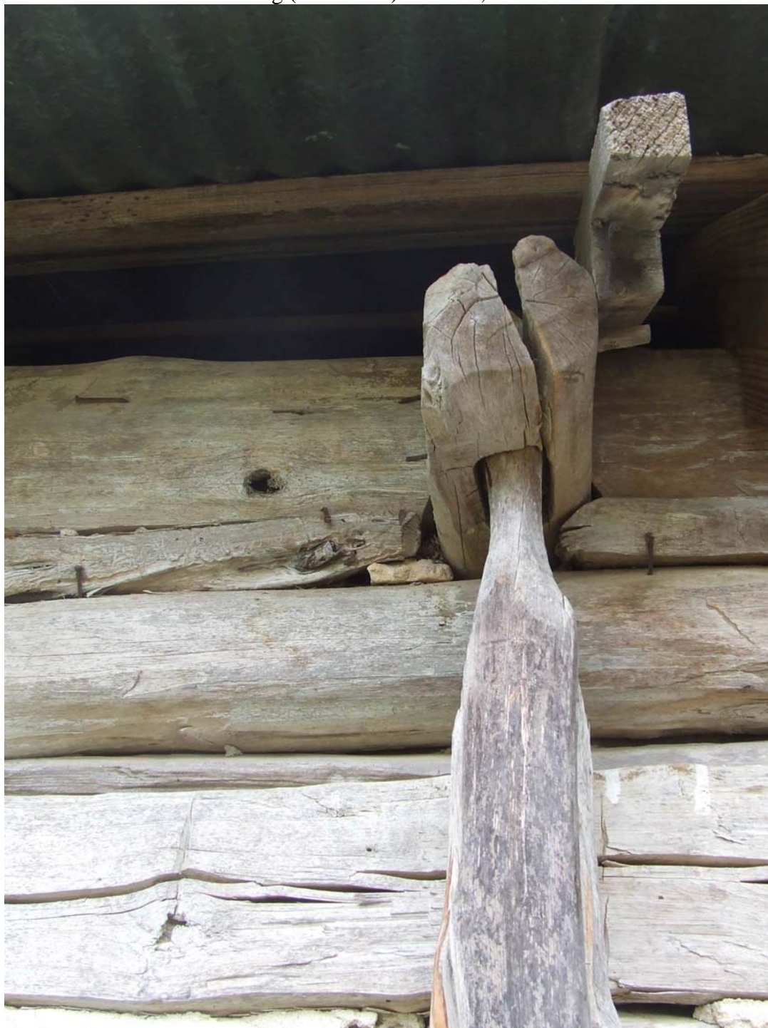
TX_Bosque County_Colwick Homestead_0006.tiff Detail of external wall bracing (south wall). June 26, 2014.
