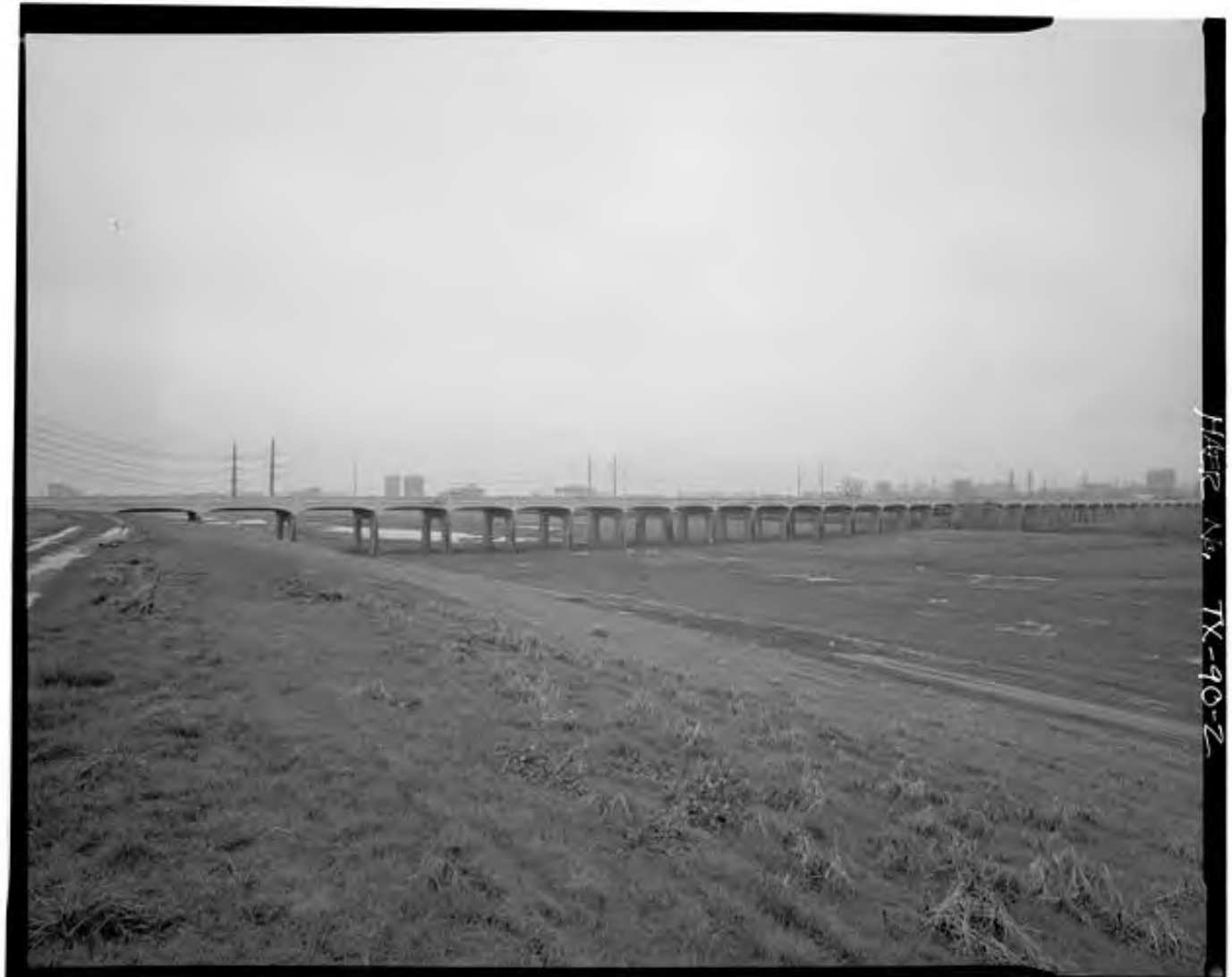
2001 HAER Photo 2 South side, looking north
