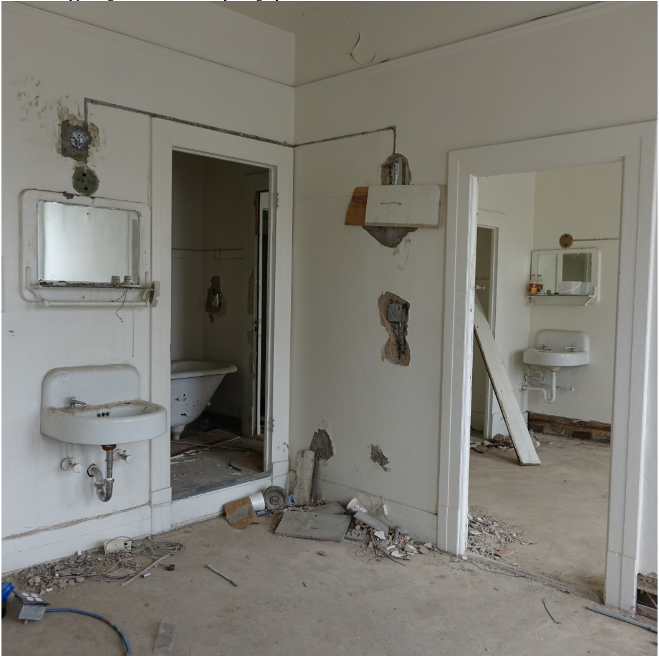
Photo 22. Typical guest room. Photo by Gregory Smith.
