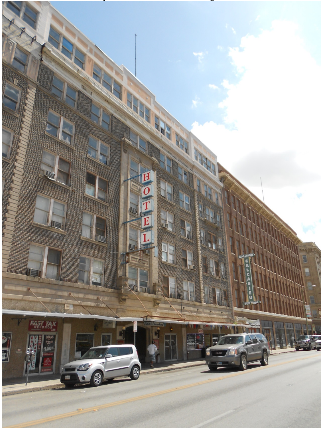
Photo 1. East side of Broadway, Travelers Hotel on left. Facing southeast.
