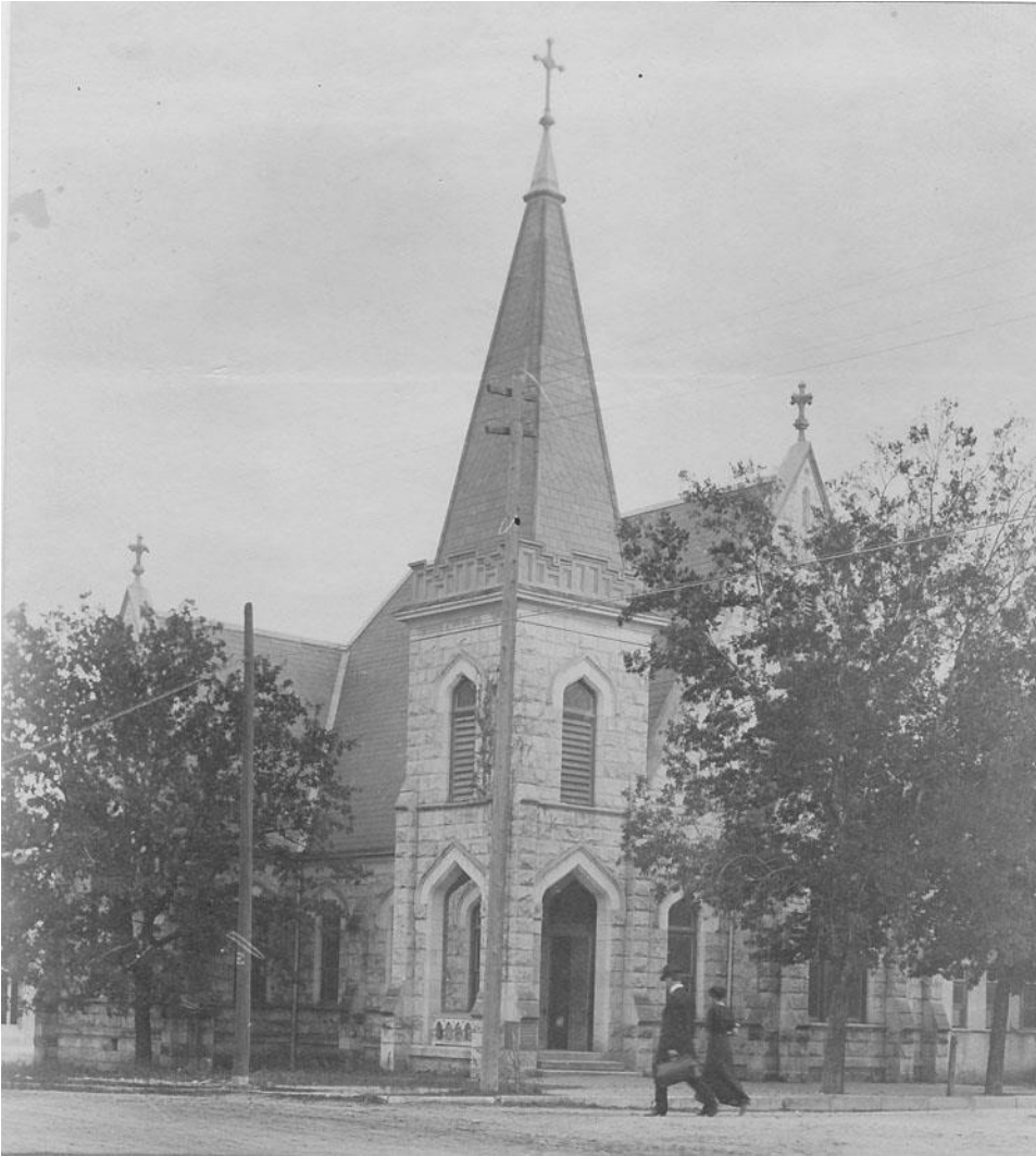
Figure 4: Primary entrance, northwest corner, camera facing southeast c. 1912. Original in All Saints' Episcopal Church archives, 209 W. 27th Street, Austin, Texas.
