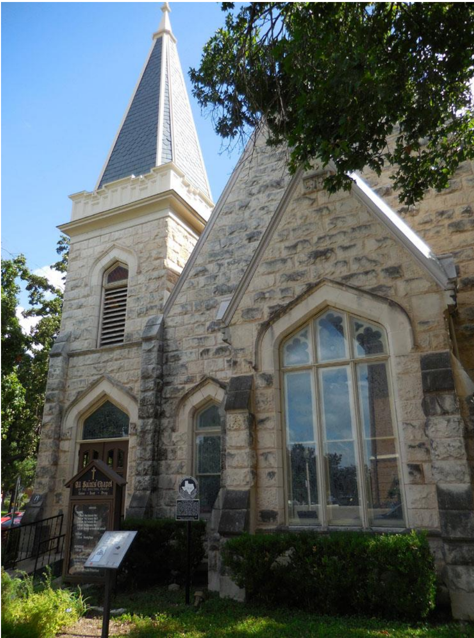
Photo #1: West façade, front entrance camera facing east
