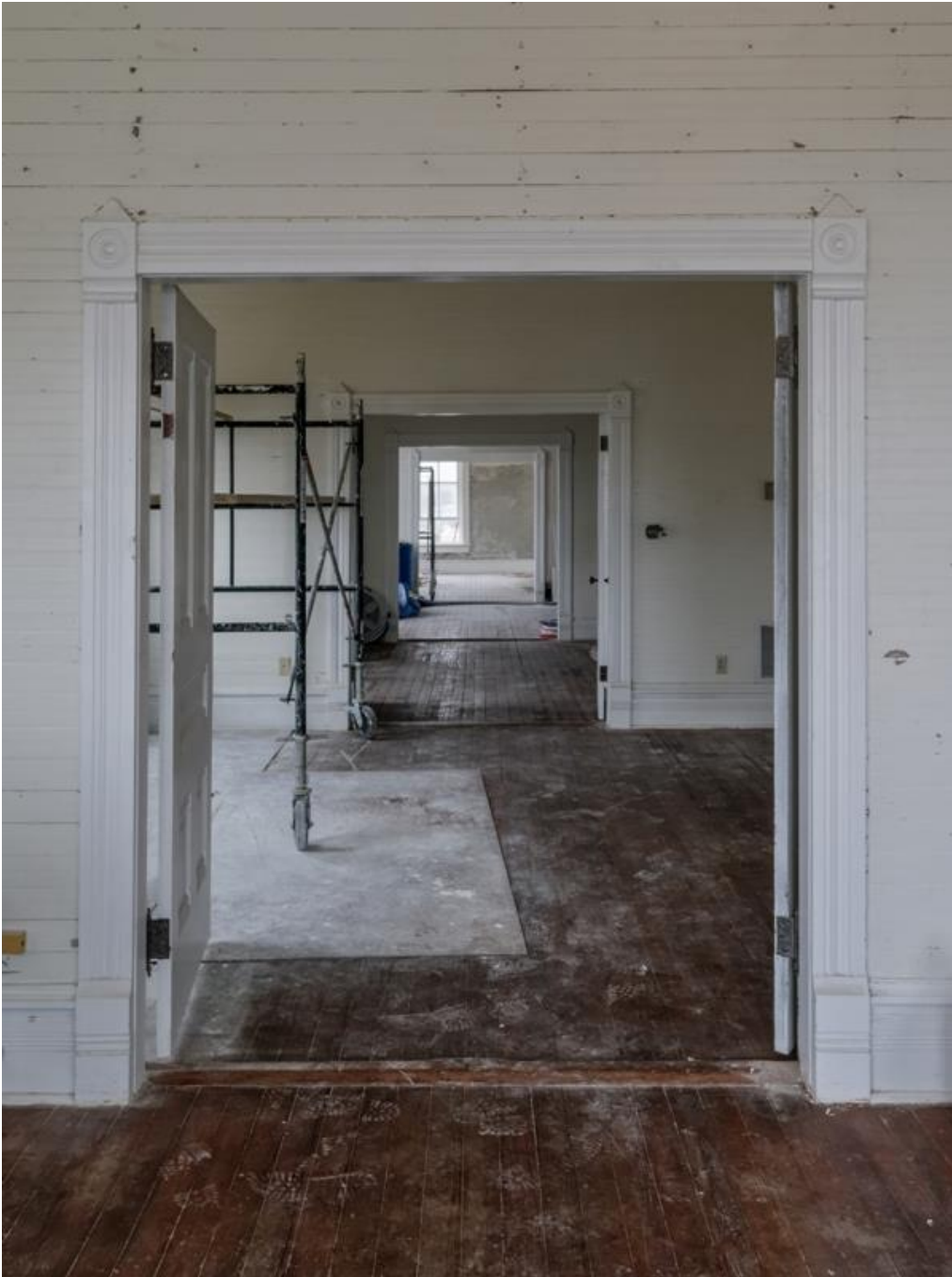
Photo 10 - Interior of Second Floor East Offices. Camera facing: West
