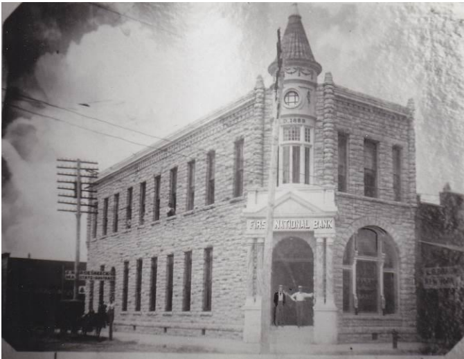
Figure 6 - Exterior view of First National Bank Building. Note telephone pole with multiple lines into Stephenville's telephone exchange which was located at the 2nd floor; ca. 1920s or 1930s. Camera facing northwest
