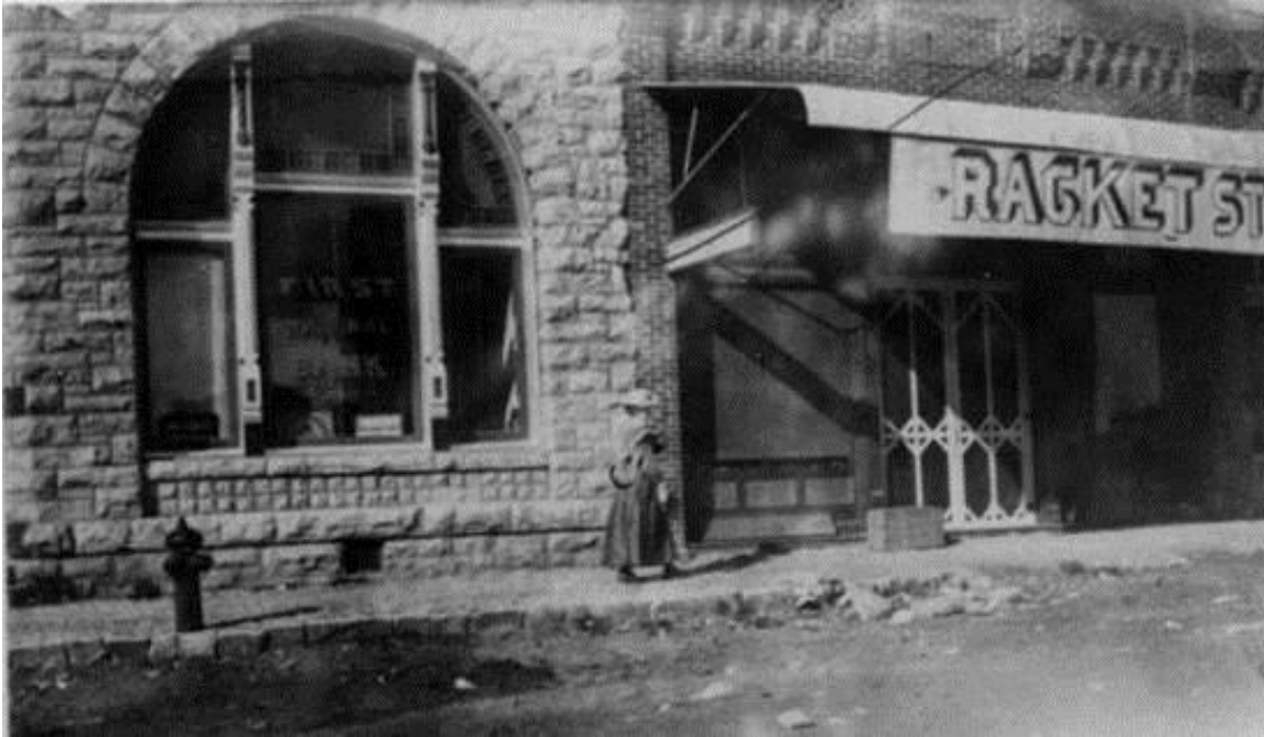
Figure 5 - Exterior view of portion of First National Bank Building and adjacent "Racket" Store. Note large arched window is intact, prior to later modification to accommodate door; ca. early 1900s. Camera facing west
