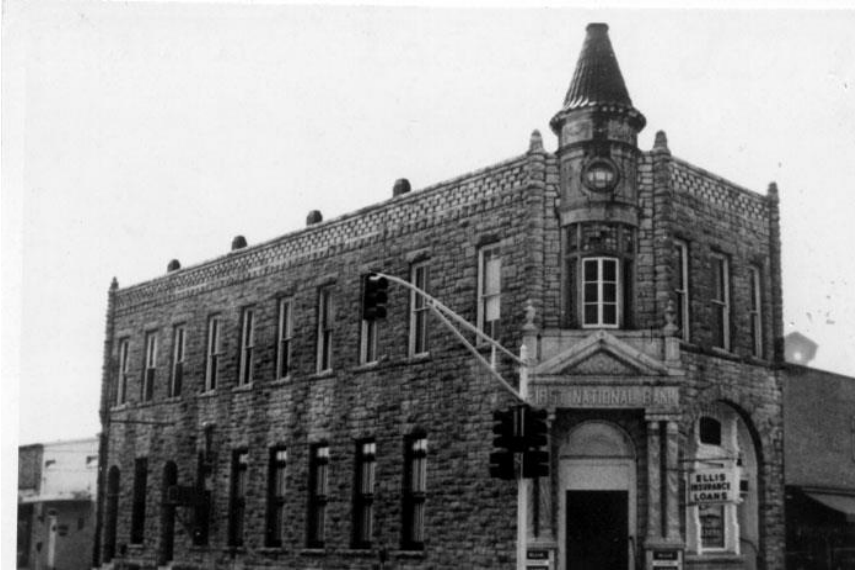
Figure 7 - Exterior view of First National Bank Building. Note replacement of metal cladding at 2nd floor turret is underway and large arched window at the front facade has been modified to accommodate new door; ca. 1930s. Camera facing northwest
