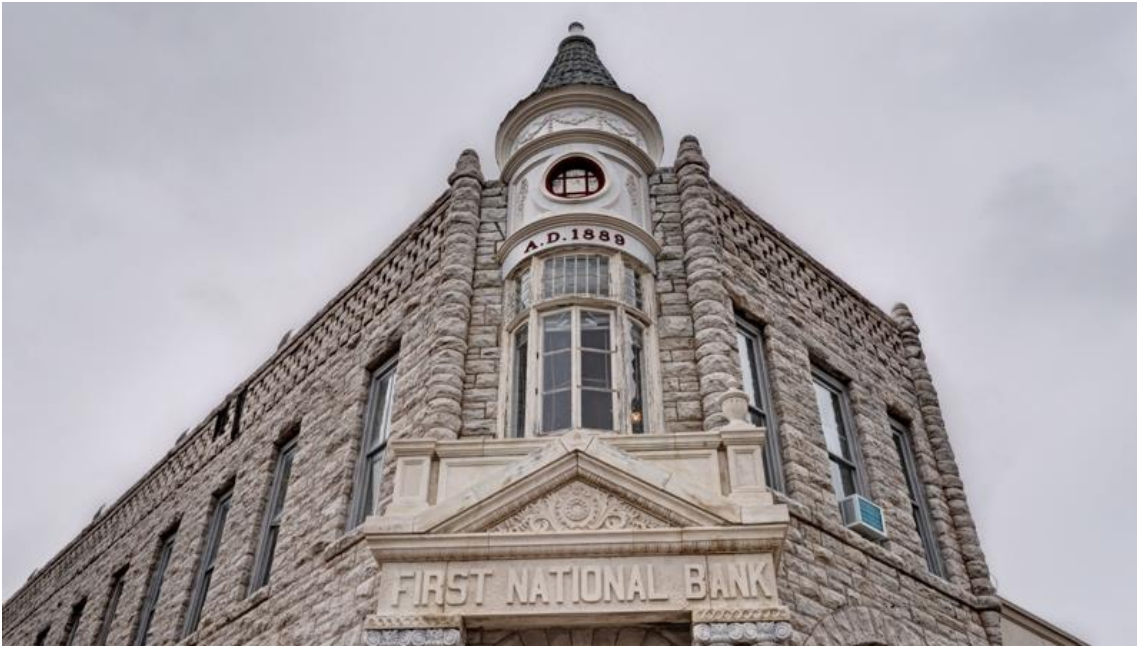
Photo 7 - Close-up of South and East Elevation Oblique with Turret and Second Floor Rounded Window. Camera facing: Northwest
