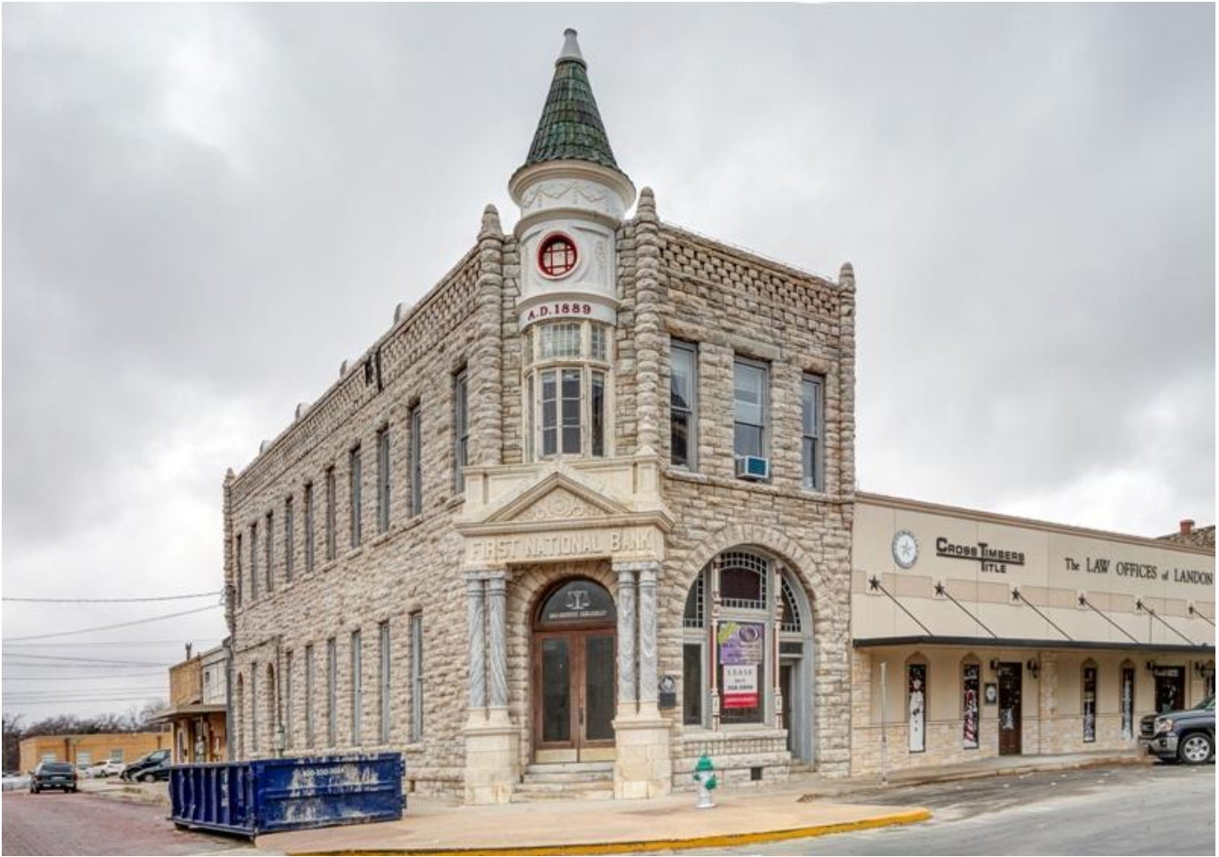
Photo 4 - South and East Elevation Oblique with Corner Entrance. Camera facing: Northwest
