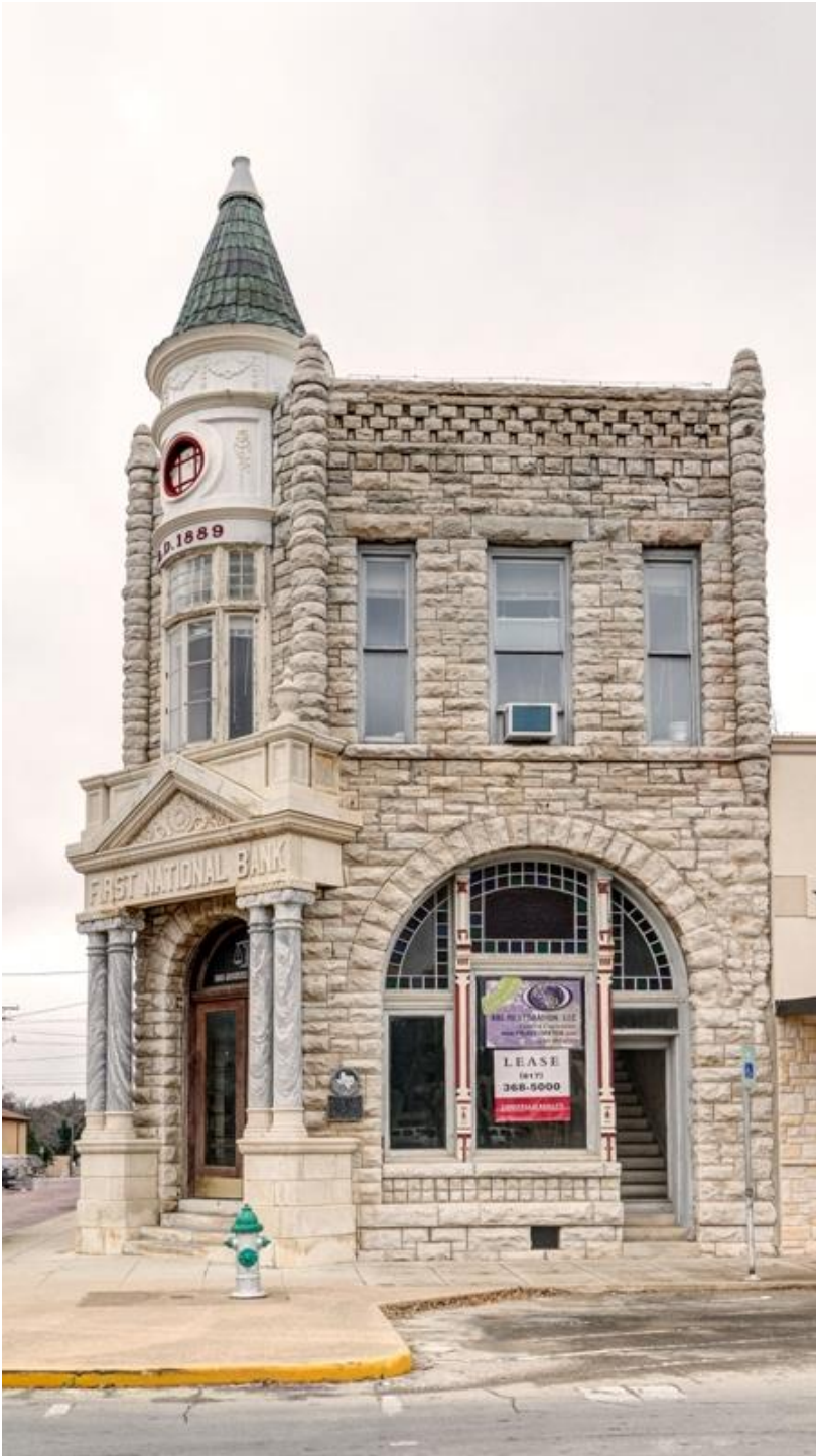
Photo 3 - East Elevation. Camera facing: West
