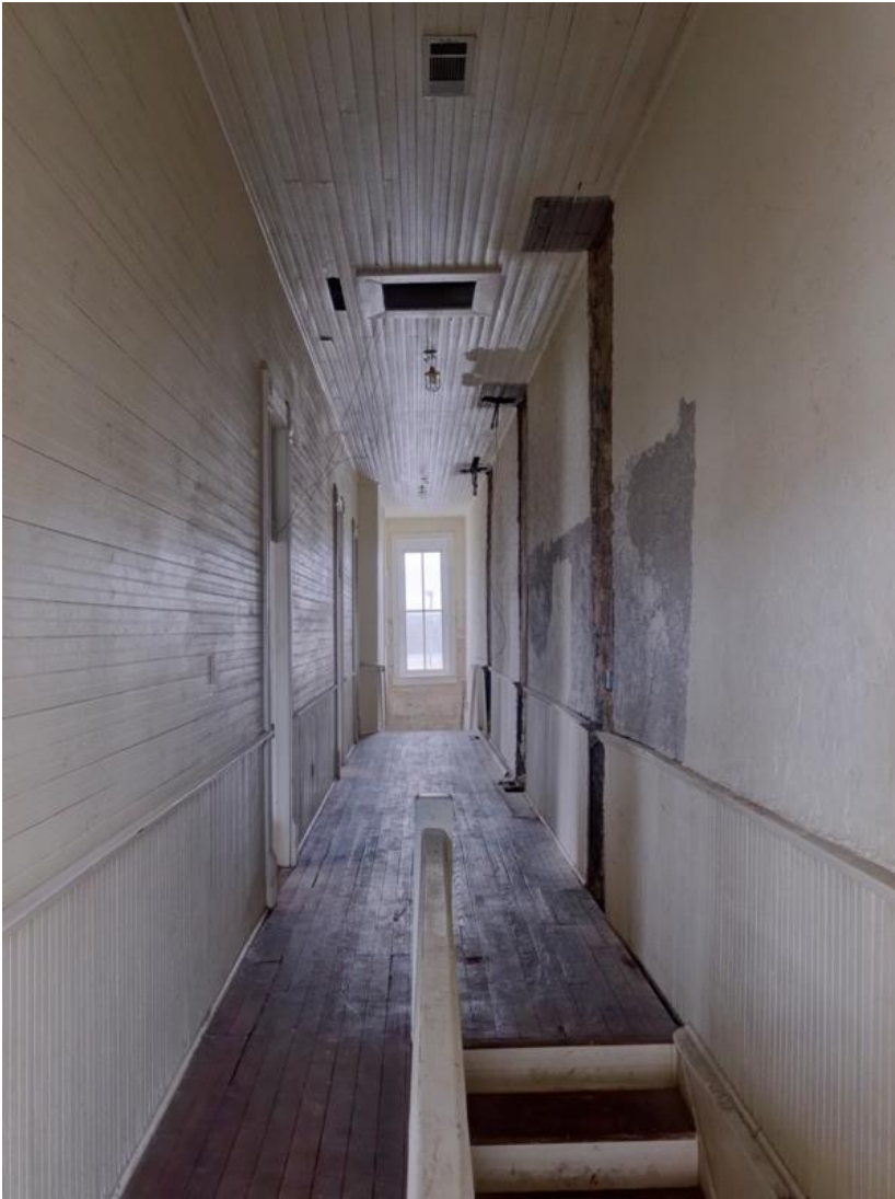
Photo 12 - Interior of Second Floor Corridor. Camera facing: West
