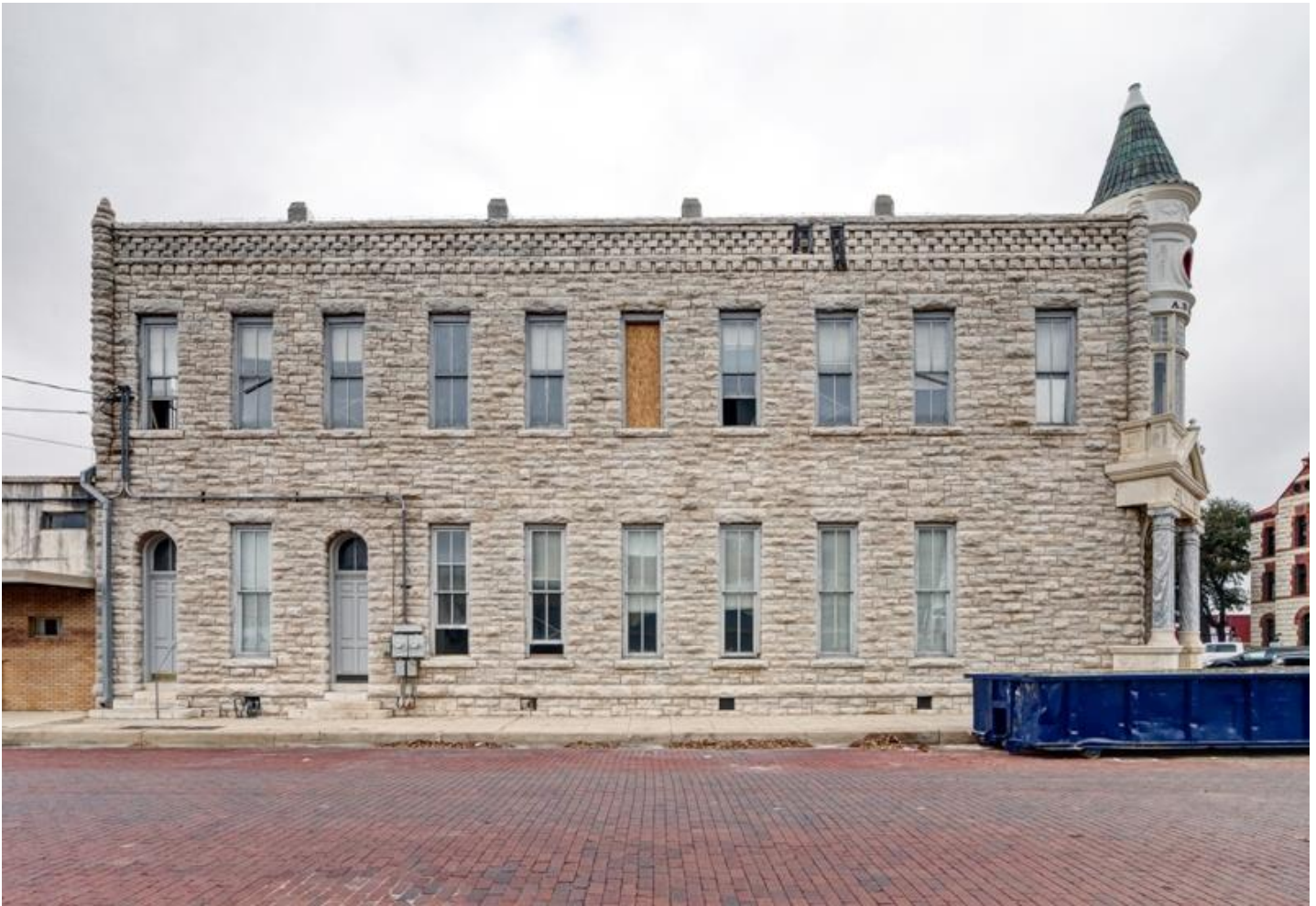
Photo 1 - South Elevation. Camera facing: North
