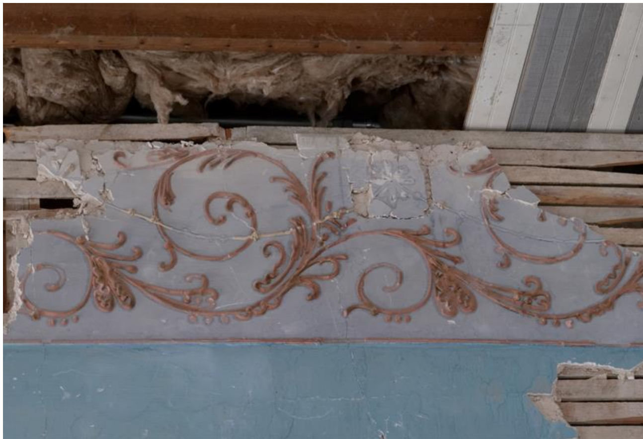
Photo 9 - Detail of Original Decorative Plaster Frieze. Camera facing: West
