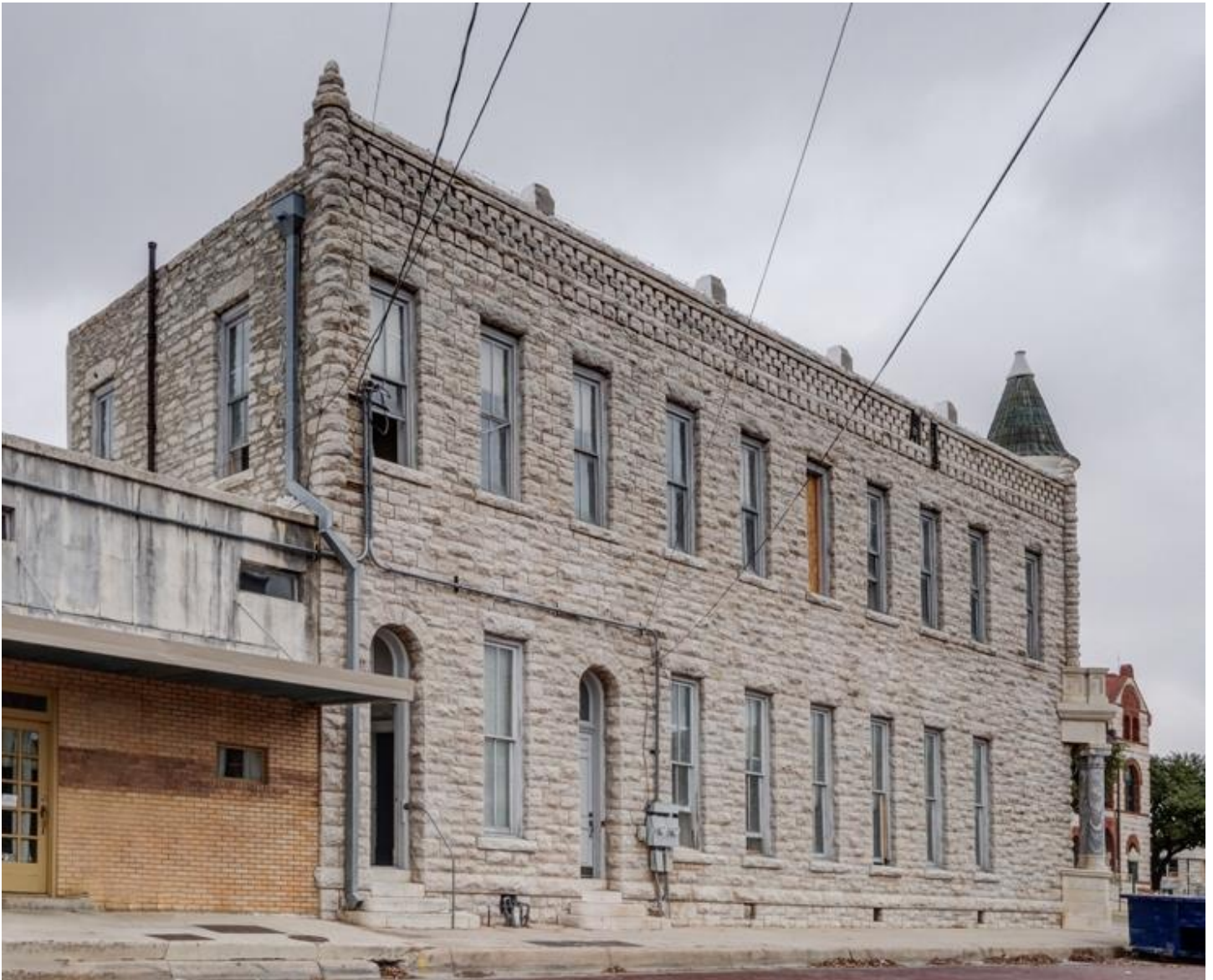
Photo 2 - South and West Elevations Oblique. Camera facing: Northeast
