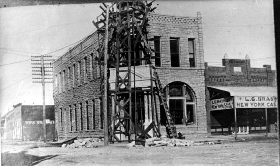
Figure 3 - Exterior view of First National Bank Building during reconstruction of corner, following fire; c. 1902. Camera facing northwest
