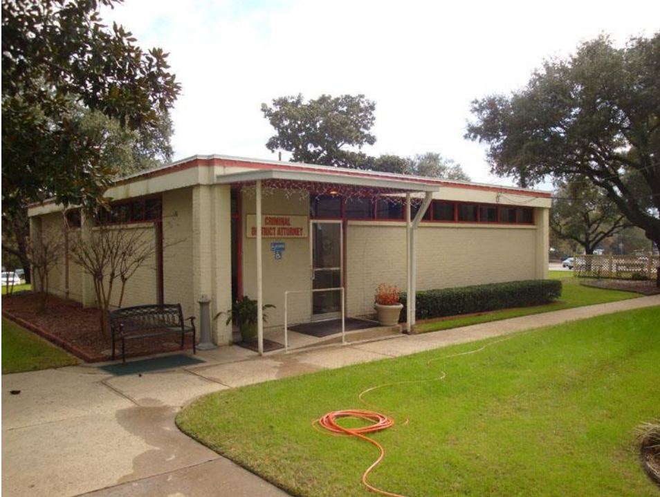
TX_Tyler County_Tyler County Courthouse_0011.tif Noncontributing annex. Camera facing southeast.
