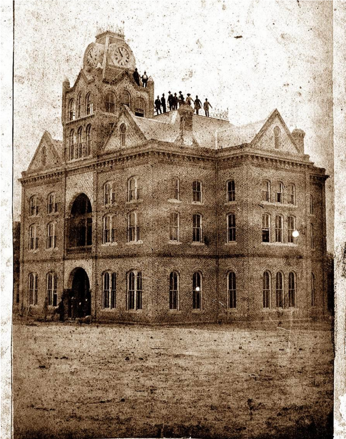
Figure 14: Courthouse soon after completion in 1891.
