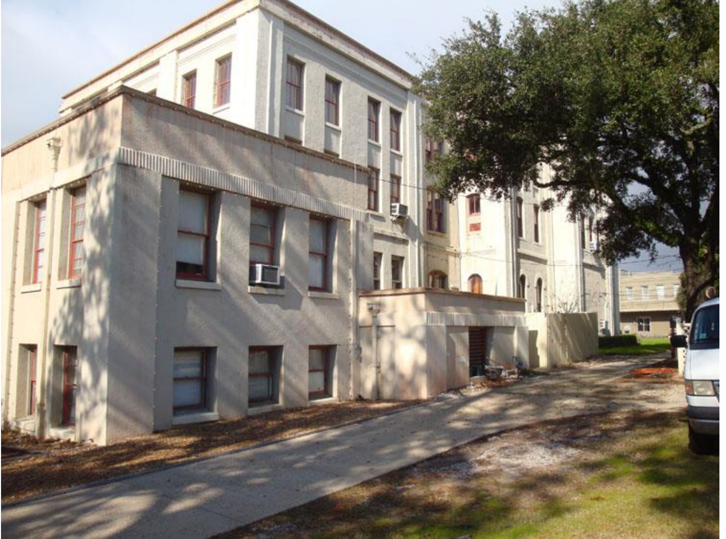
TX_Tyler County_Tyler County Courthouse_0006.tif East façade. Camera facing approximately northwest.
