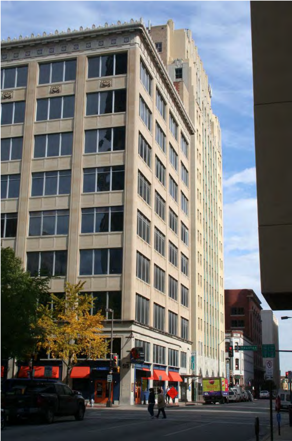
Photo 2: View of west and south elevations, looking east
