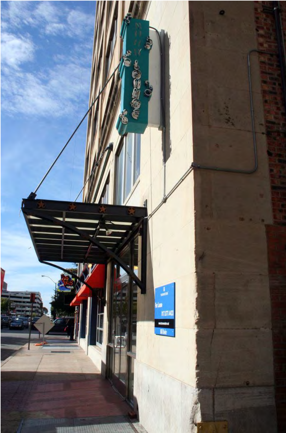
Photo 4: View of south elevation, detail of main entrance, looking west
