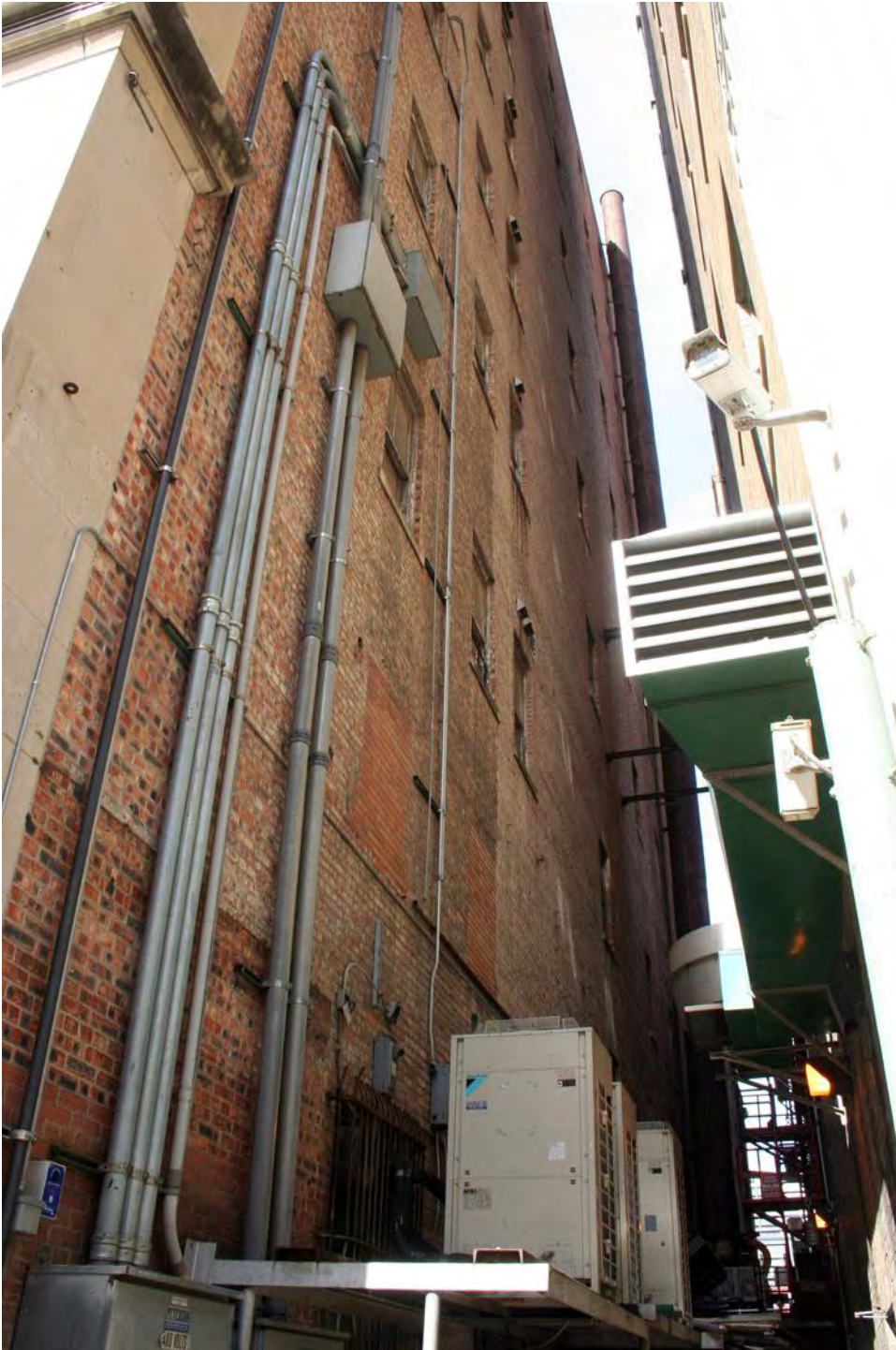
Photo 5: View of east elevation, looking north
