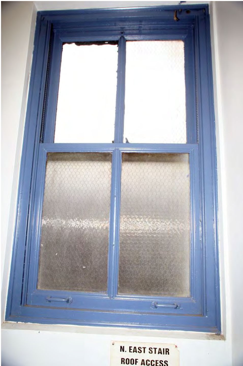
Photo 16: Second floor, detail of window, looking east
