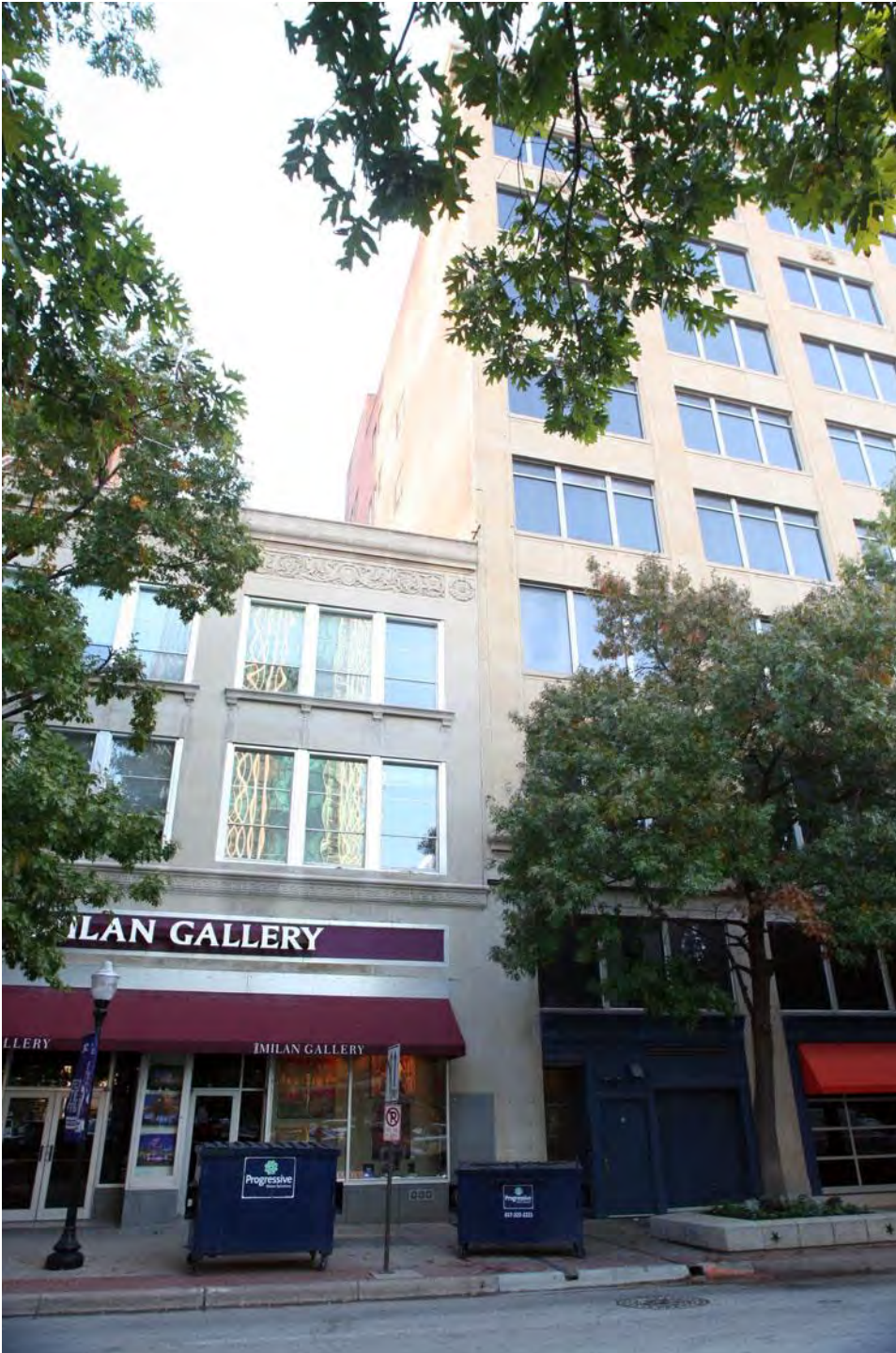
Photo 10: View of west and north elevations, looking east
