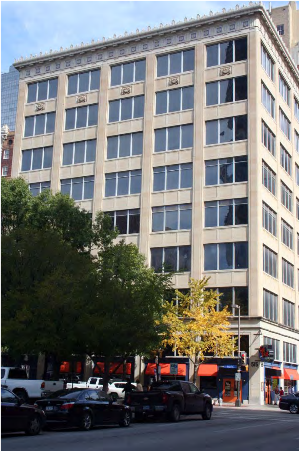
Photo 6: View of west elevation, looking northeast
