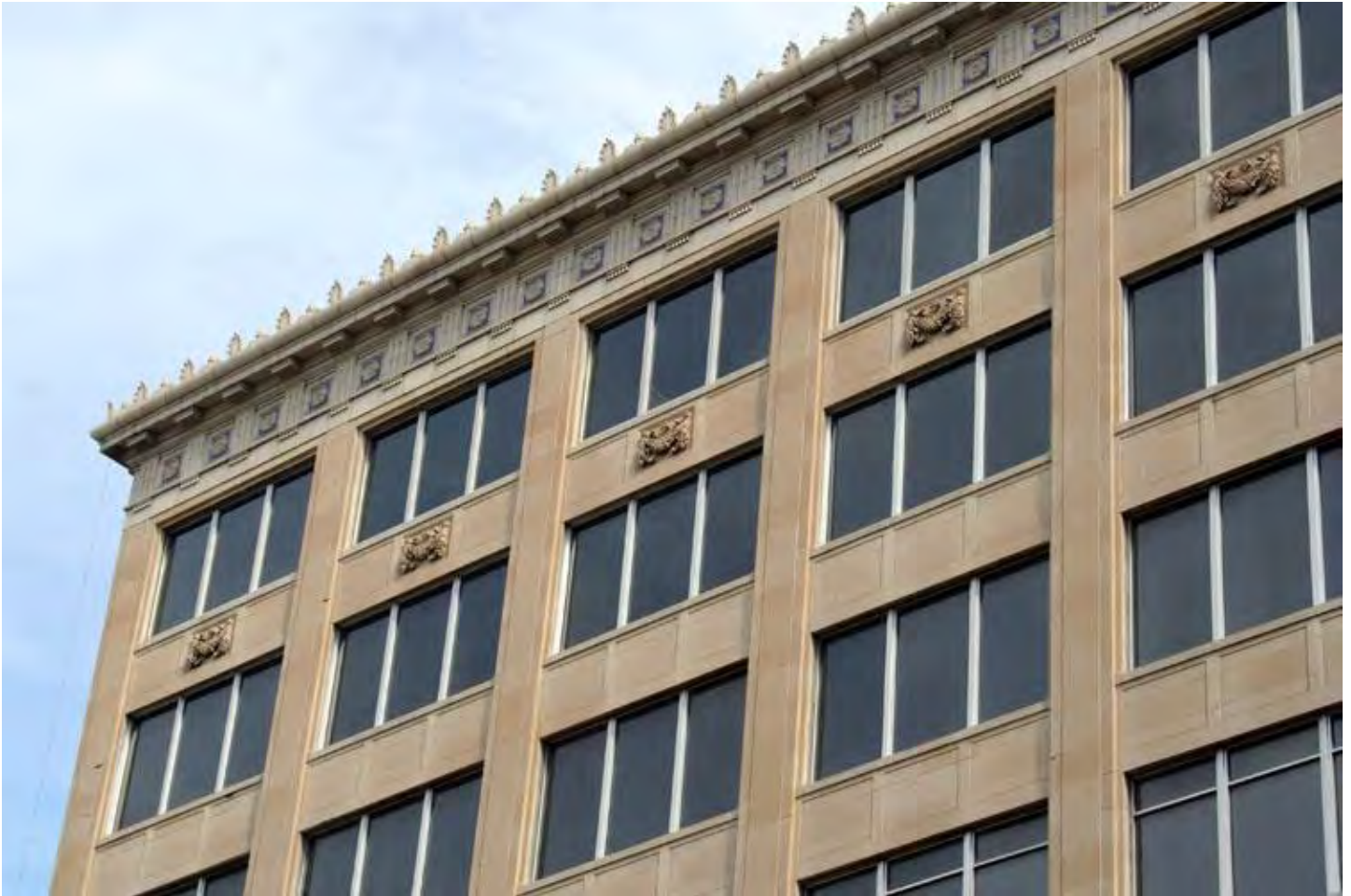
Photo 9: View of west elevation, detail of cornice, looking northeast
