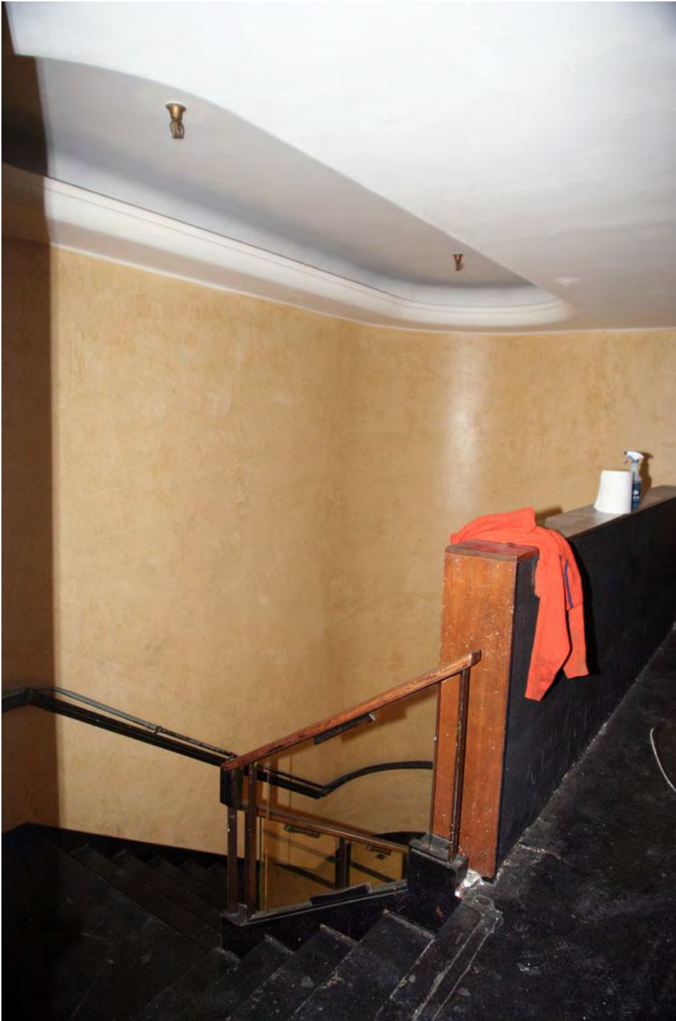
Photo 15: Mezzanine, looking southeast at stair
