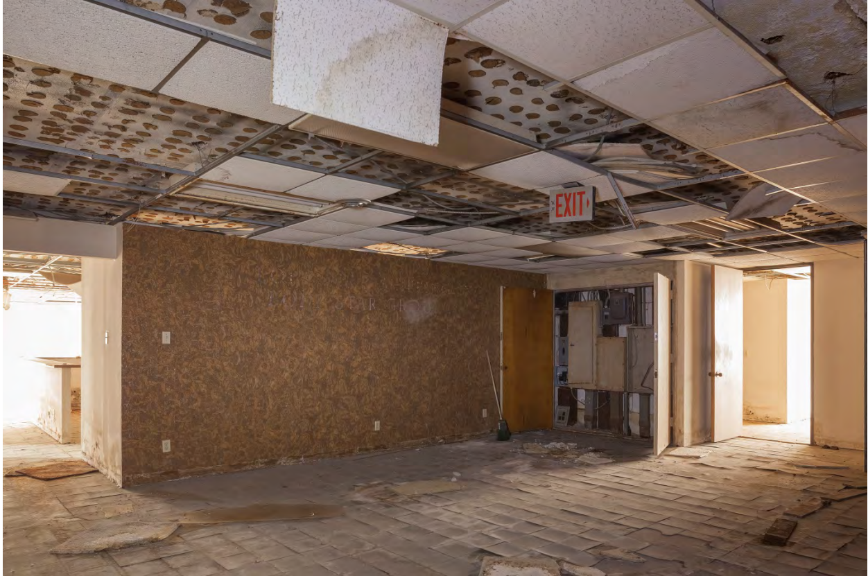
Photo #15 (TX_HarrisCounty_MelroseBuilding_photo_0015) , Typical upper floor tenant space
