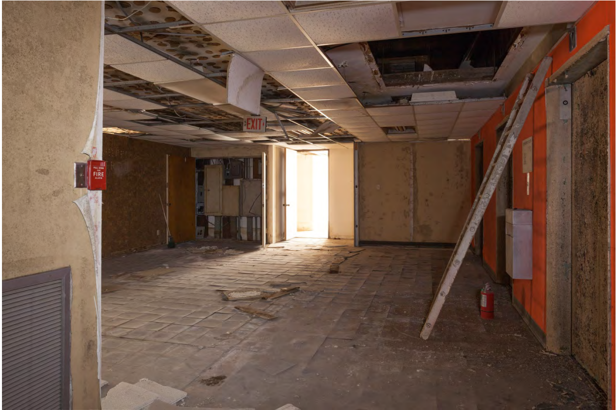
Photo #16 (TX_HarrisCounty_MelroseBuilding_photo_0016) Typical upper floor tenant space
