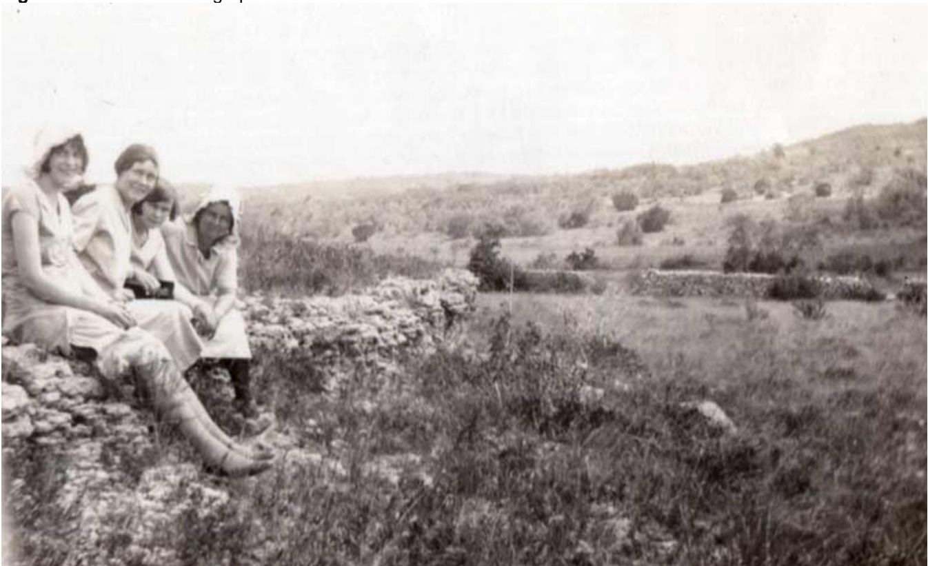
Figure 13. Historic Photograph of Stone Fences
