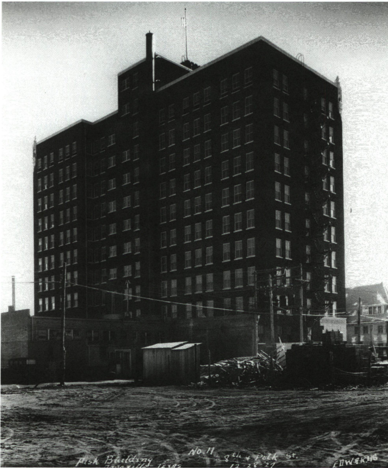
Façade at Northwest Corner, 1928.
