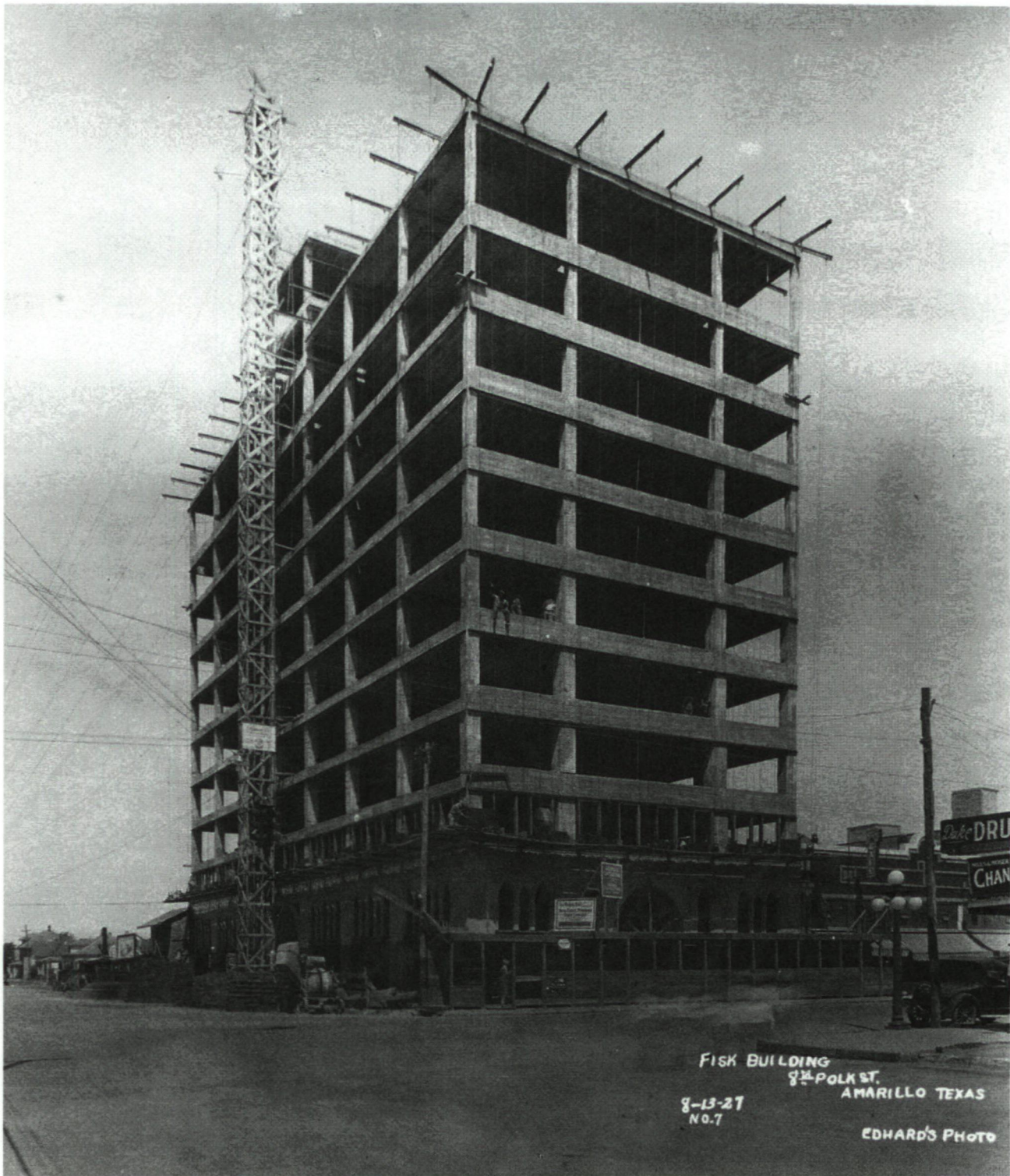
Stone Veneer Construction, 1927.
