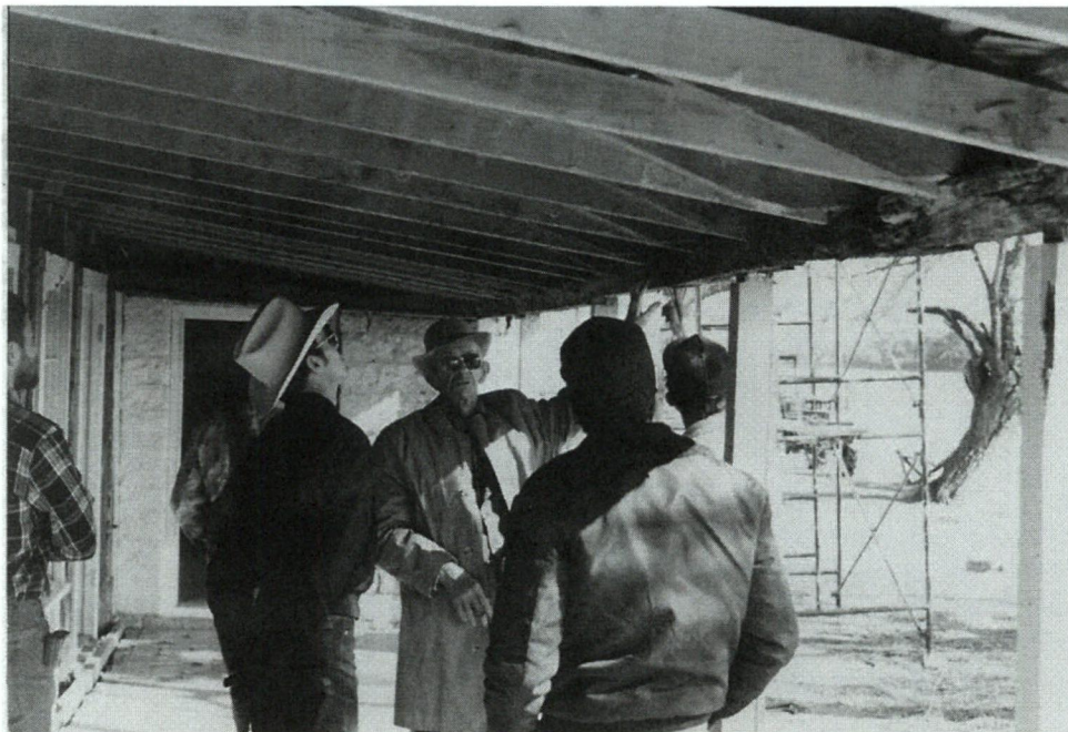
Figure 6: Photo taken during 1986 restoration showing original oak porch beam and new porch rafters. Raiford Stripling facing camera. Courtesy Amy and Randall Walton.
