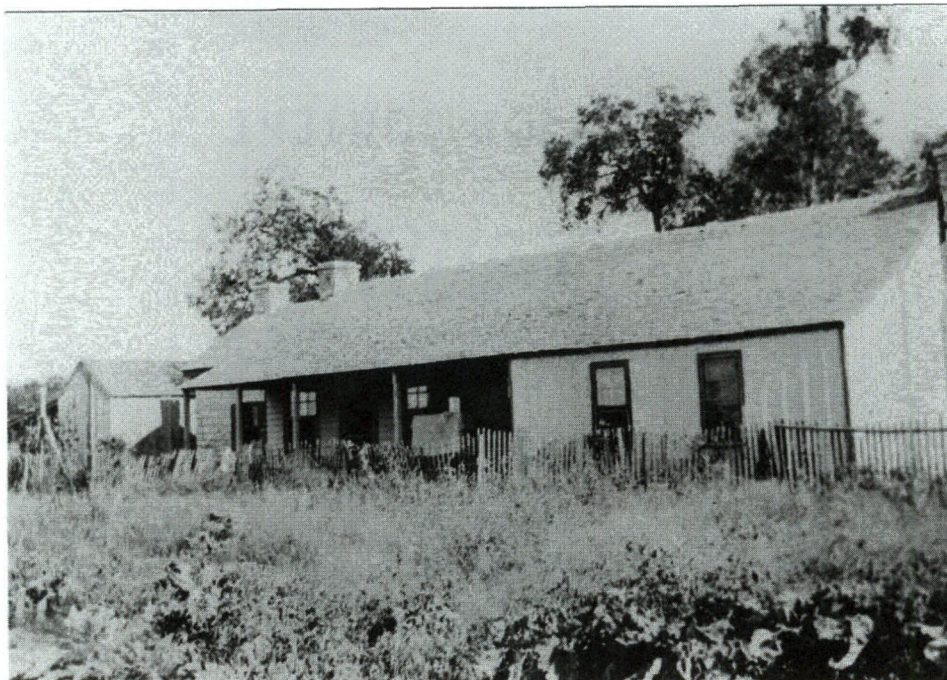
Figure 2: Looking southeast at north elevation, showing a portion of the rear porch enclosed, c. 1910. Courtesy Amy and Randy Walton.
