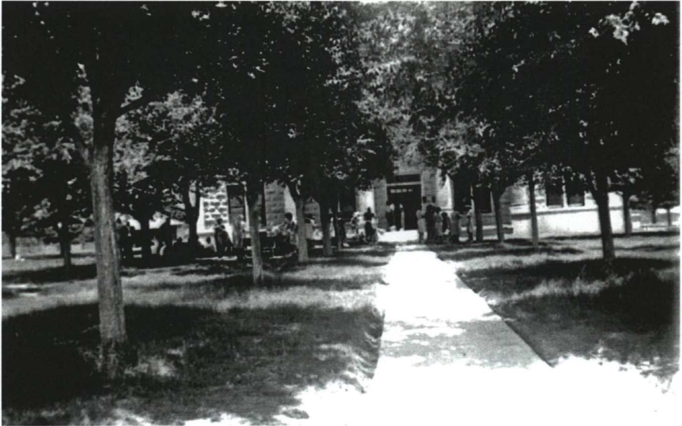
Photo 7. West elevation of the Glasscock County Courthouse with allée of trees, ca. 1940.
