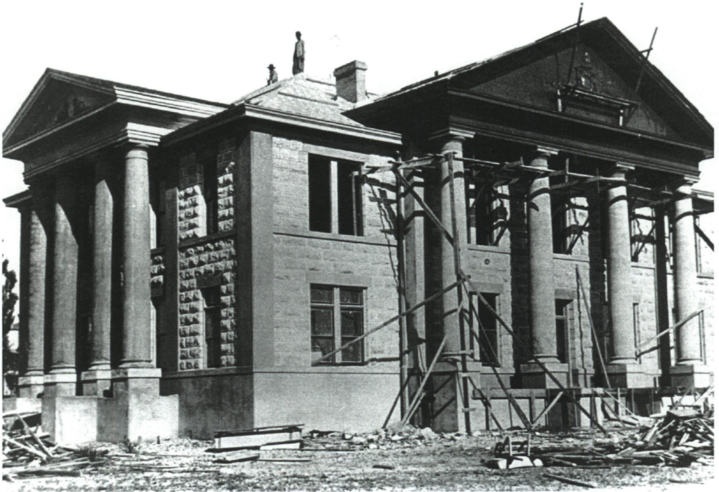
Photo 3. Southeast oblique view of the Glasscock County Courthouse under construction, ca. 1910.
