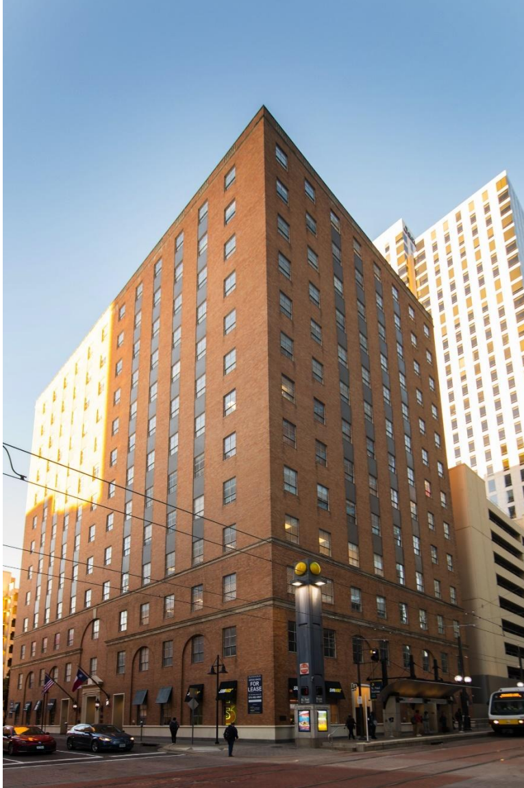
Photo 1. Exterior, southwest and southeast elevations, view north.
