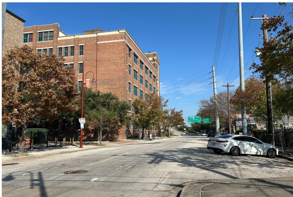
Photo 4. Streetscape, Chenevert Street; view north
