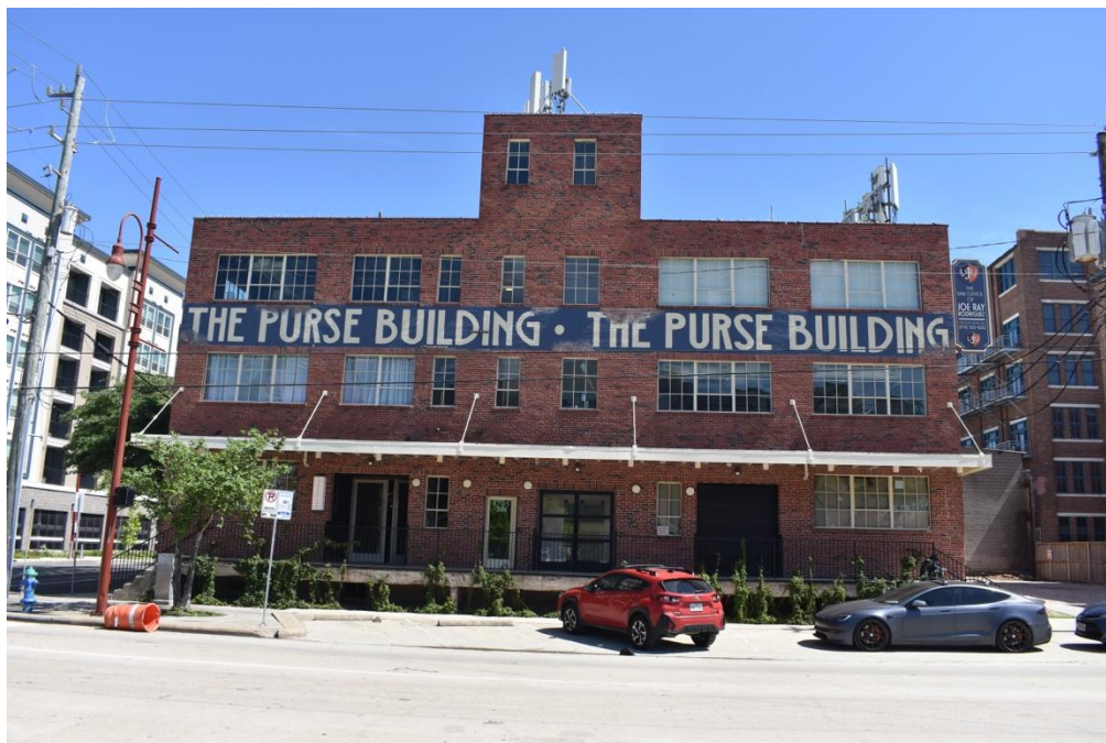
Photo 18. 1701 Commerce, southwest (primary) elevation; view northeast
