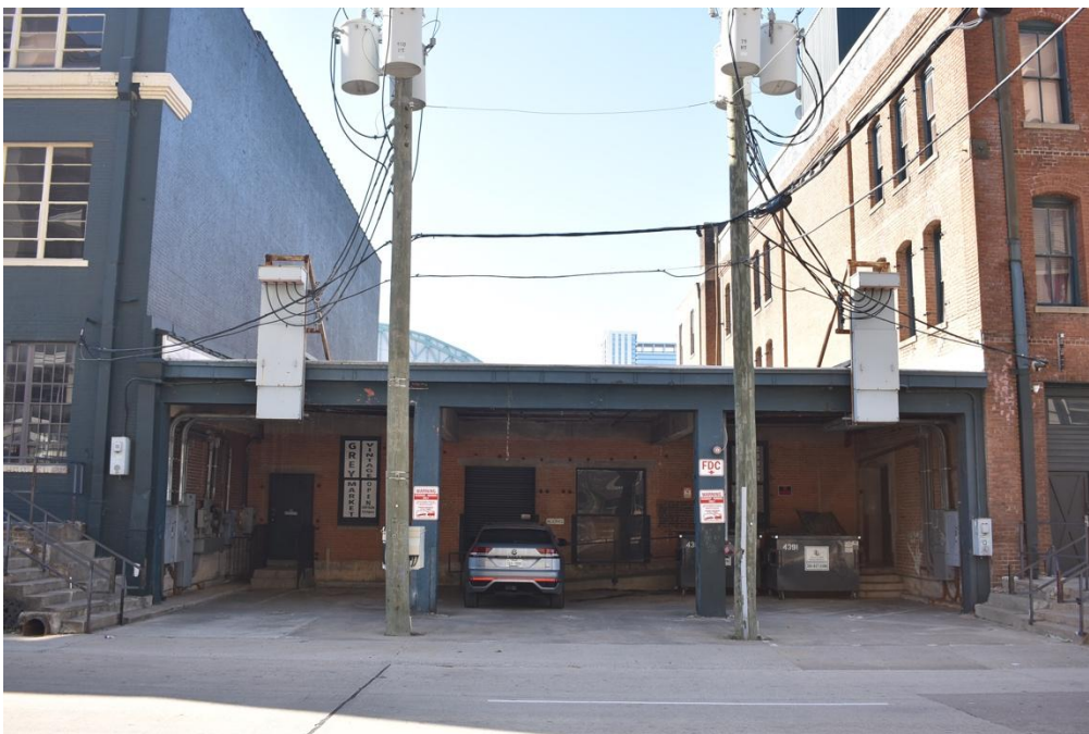
Photo 6. 101 Crawford, northeast elevation and 1929 addition; view southwest
