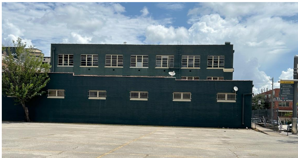
Photo 17. 100 Jackson, southwest (rear) elevation; view northeast
