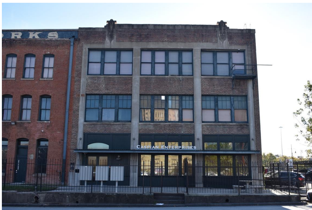
Photo 8. 101 Crawford, northwest elevation of 1920 addition; view southeast
