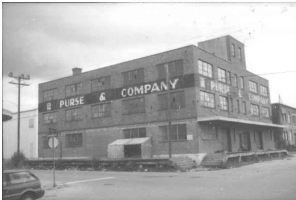
Figure 13. J. L. Jones Warehouse (Resource 3, 1701 Commerce), oblique view of northwest (left) and southwest (right) elevations, as they appeared in 1991 (Barrie Scardino/Texas Historical Commission)
