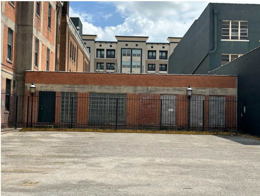
Photo 10. 101 Crawford, southwest (rear) elevation of 1929 addition; view northeast
