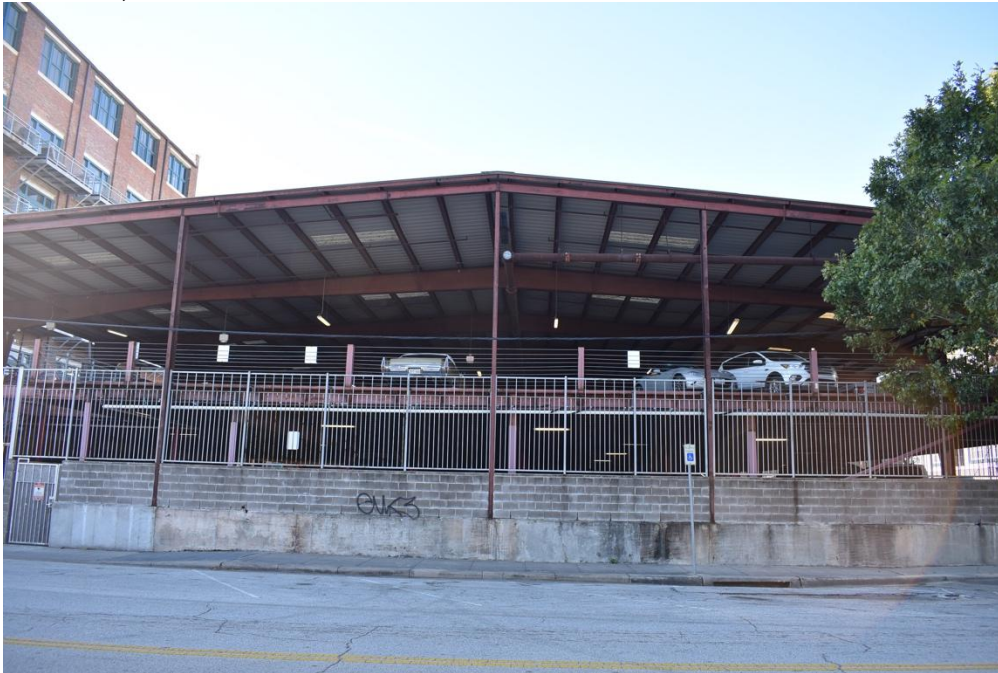
Photo 23. City Lofts Parking Garage (noncontributing structure), 1702 Ruiz, northeast (primary) elevation; view southwest
