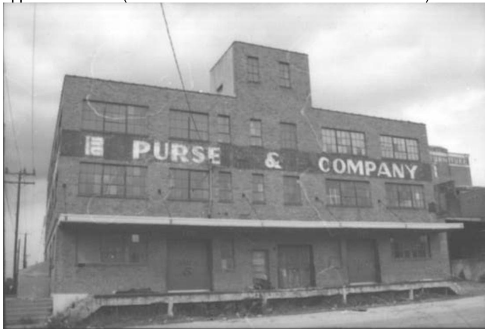
Figure 12. J. L. Jones Warehouse (Resource 3, 1701 Commerce), front/southwest elevation, as it appeared in 1991 (Barrie Scardino/Texas Historical Commission)
