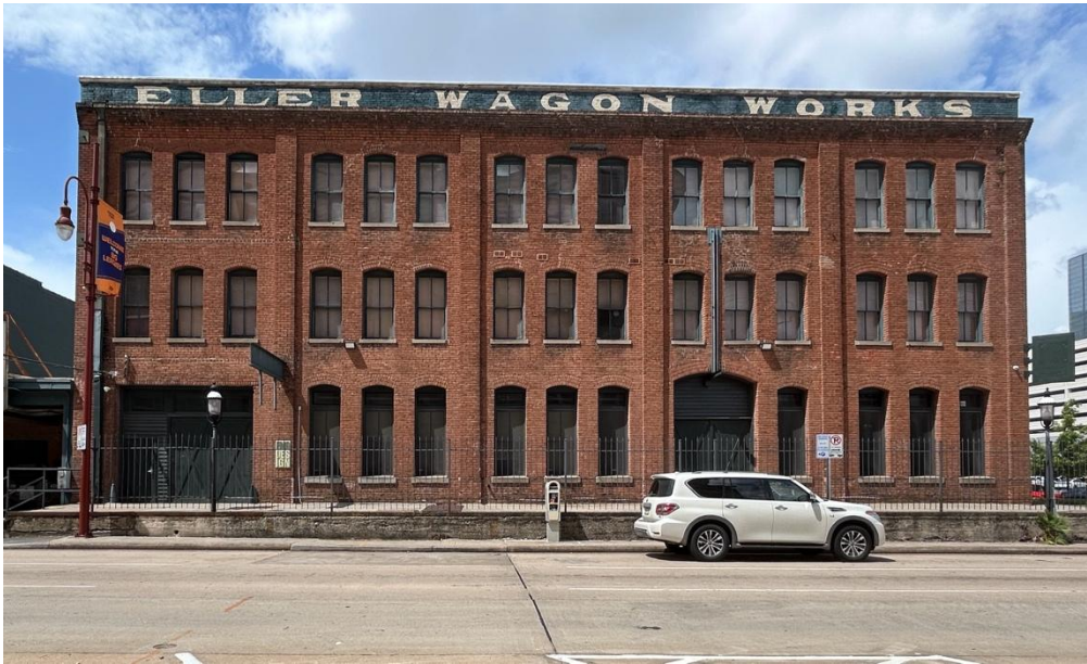
Photo 5. 101 Crawford, northeast (primary) elevation; view southwest
