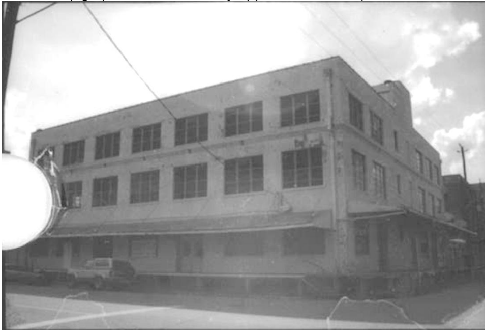
Figure 10. Western Electric Building (Resource 2, 100 Jackson), oblique view of southeast (left) and northeast (right) elevations, as they appeared in 1991 (Barrie Scardino/Texas Historical Commission)
