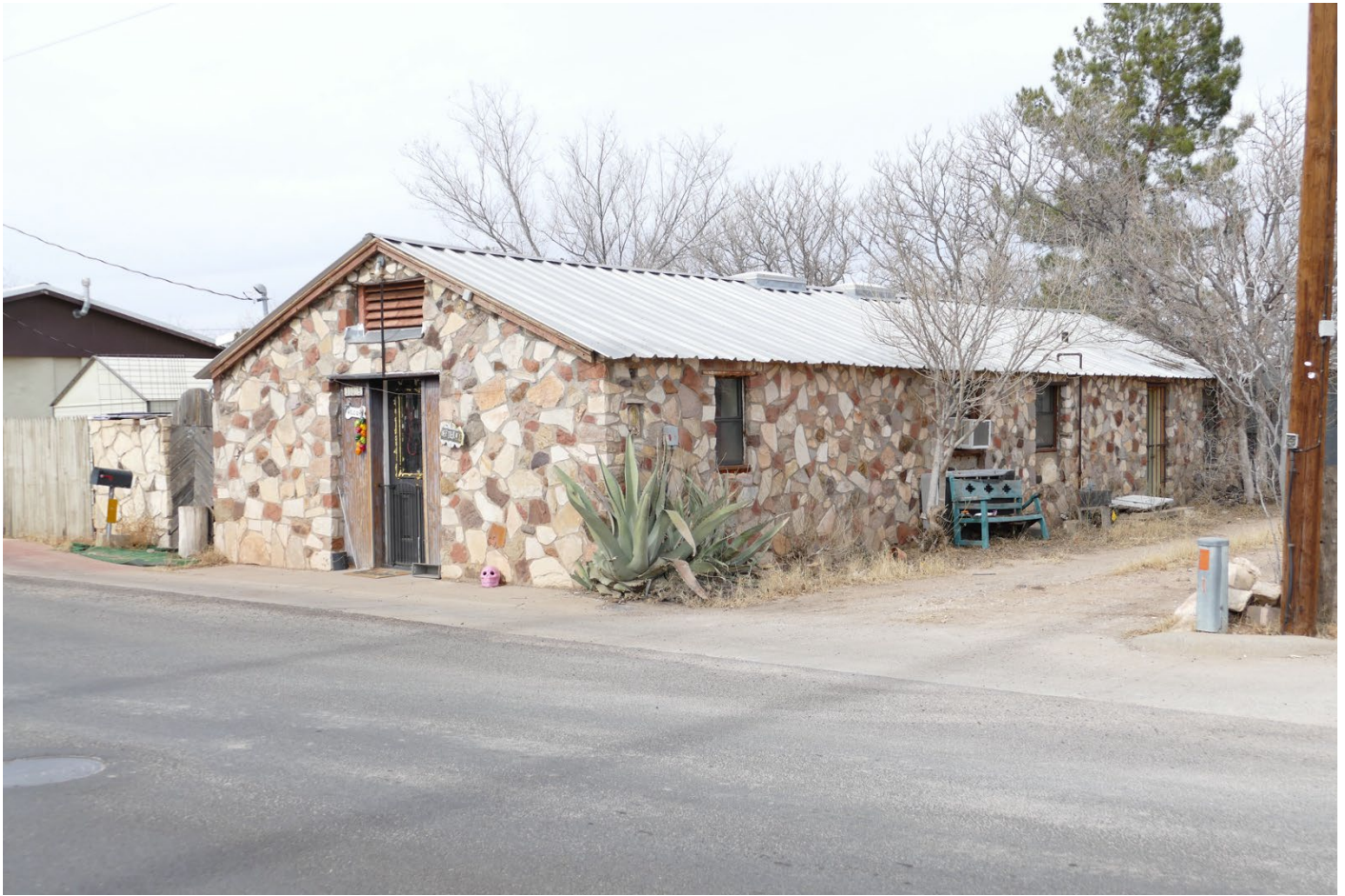
Photo 27. A former WWII temporary building moved to Alpine and clad with native stone (Resource 126).
