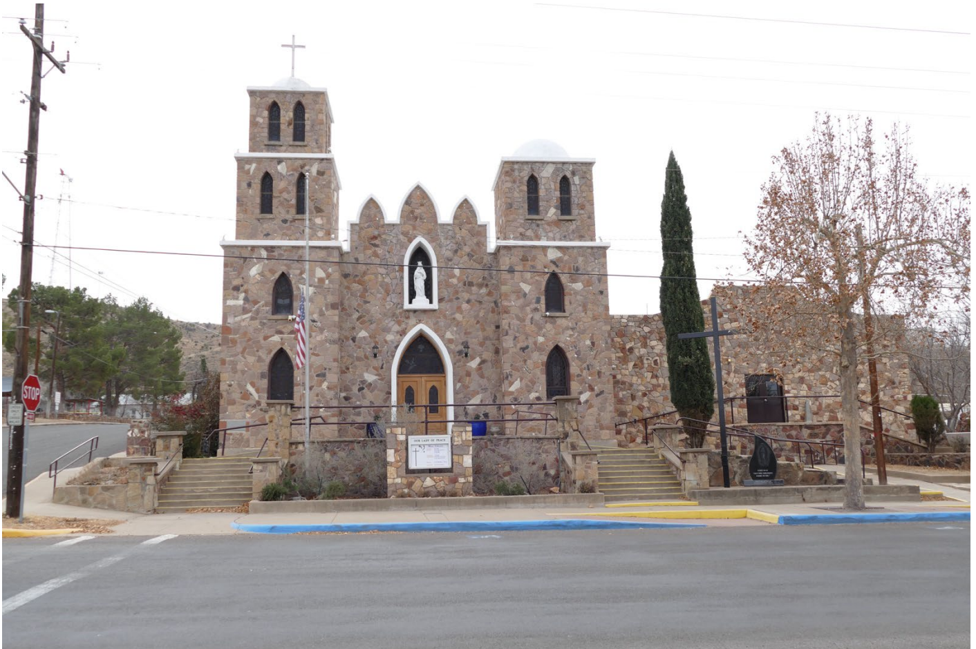
Photo 17. Our Lady of Peace Catholic Church (Resource 32, at left) and adjacent Parish Hall (Resource 33, at right). View south.
