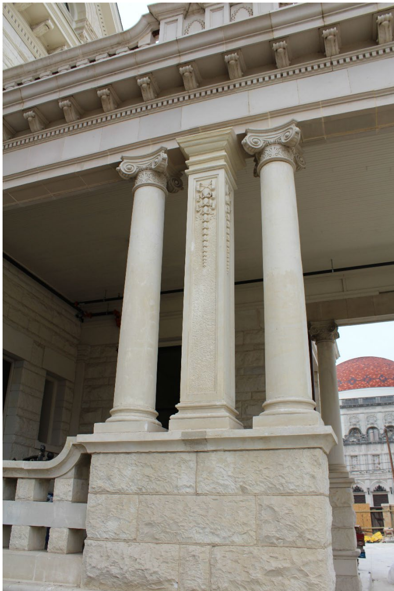
Photo 7. Koehler House – Porte-cochère columns, camera facing northwest. January 30, 2026
