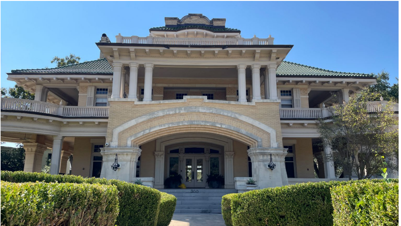
Figure 36: Roy and Madge Hearne House, 2025, north elevation
