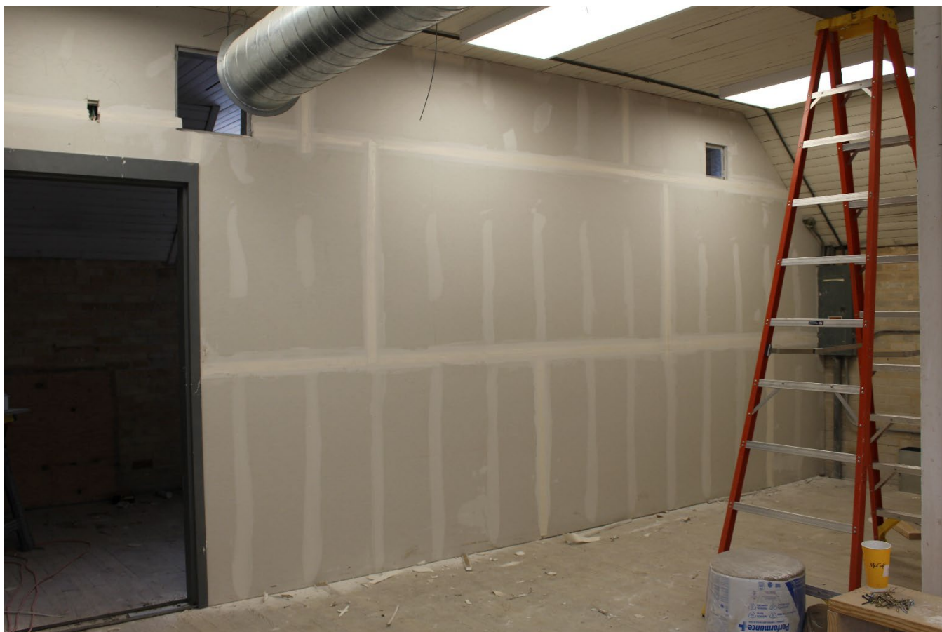
Photo 26. Carriage House – Second floor interior space, camera facing southwest. January 30, 2026
