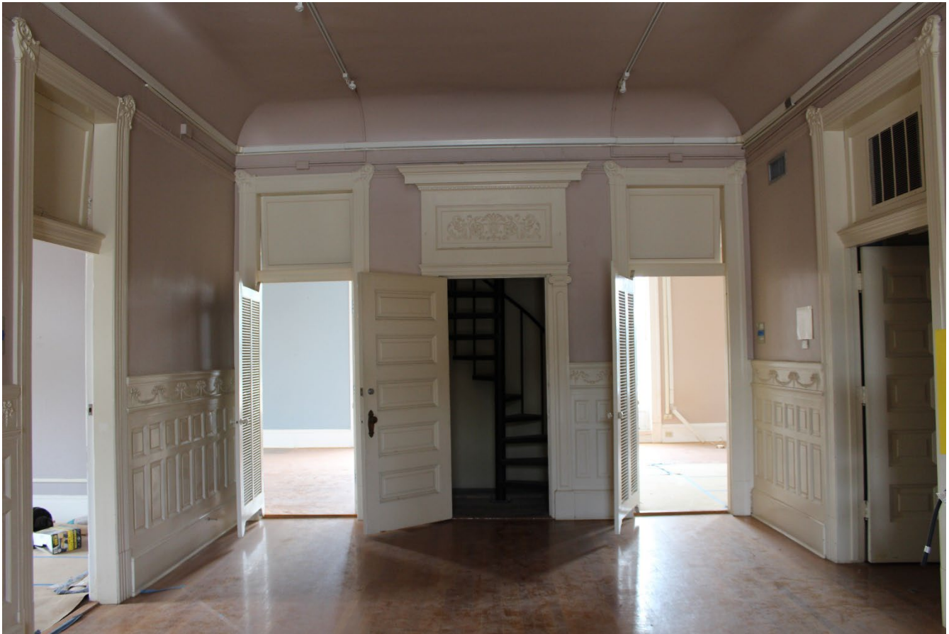
Photo 14. Koehler House – Second floor central hallway, camera facing south. June 11, 2025
