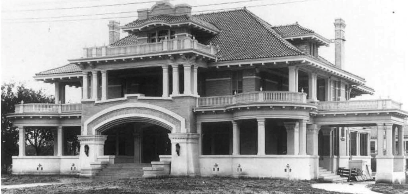
Figure 35: Roy and Madge Hearne House, 1910, north and east elevations, Courtesy of Robert Coote
