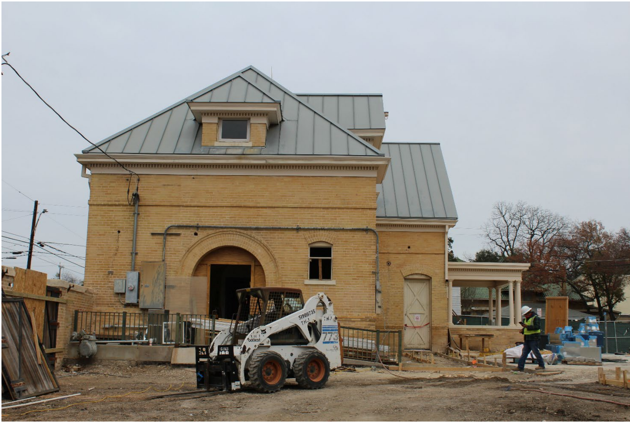
Photo 22. Carriage House – South elevation, camera facing north. January 30, 2026
