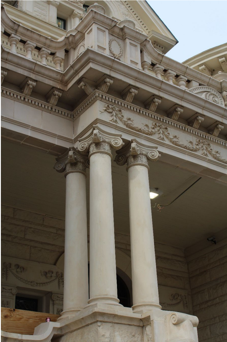
Photo 6. Koehler House – Porch columns, camera facing northwest. January 30, 2026
