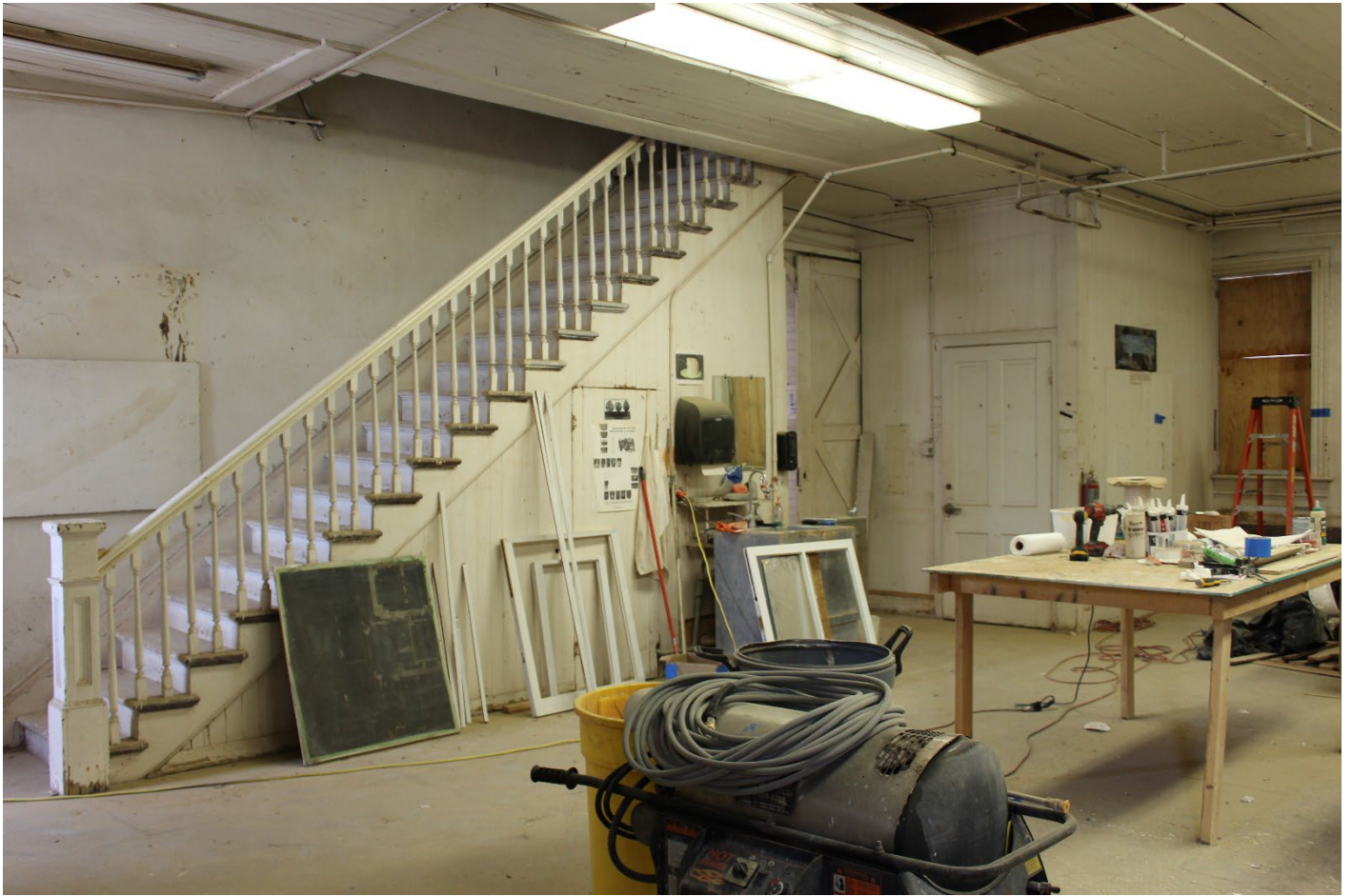
Photo 23. Carriage House – First floor interior space, camera facing southwest. June 11, 2025
