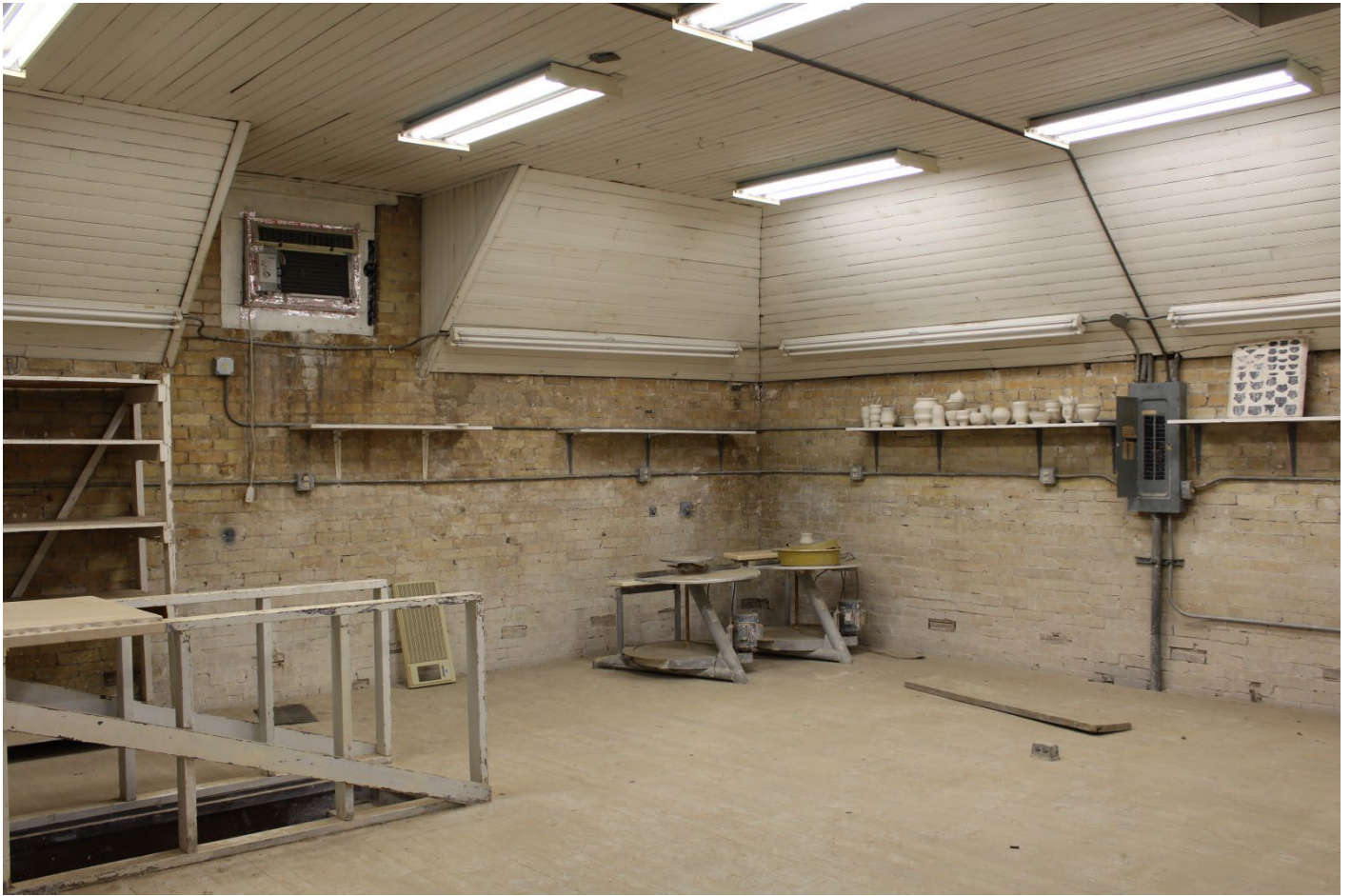
Photo 25. Carriage House – Second floor interior space, camera facing southwest. June 11, 2025
