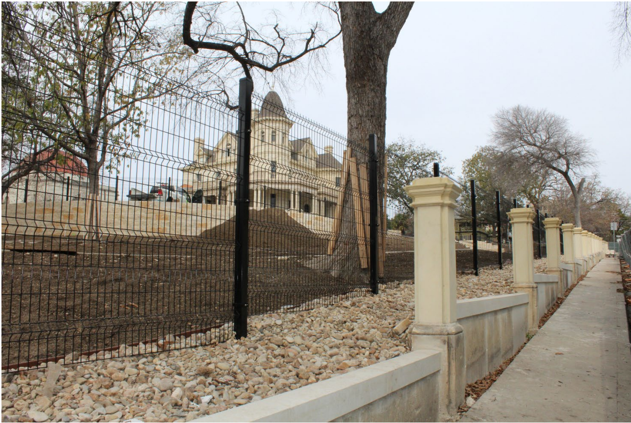
Photo 29. Ornamental limestone and metal perimeter fence - camera facing northwest. January 30, 2026
