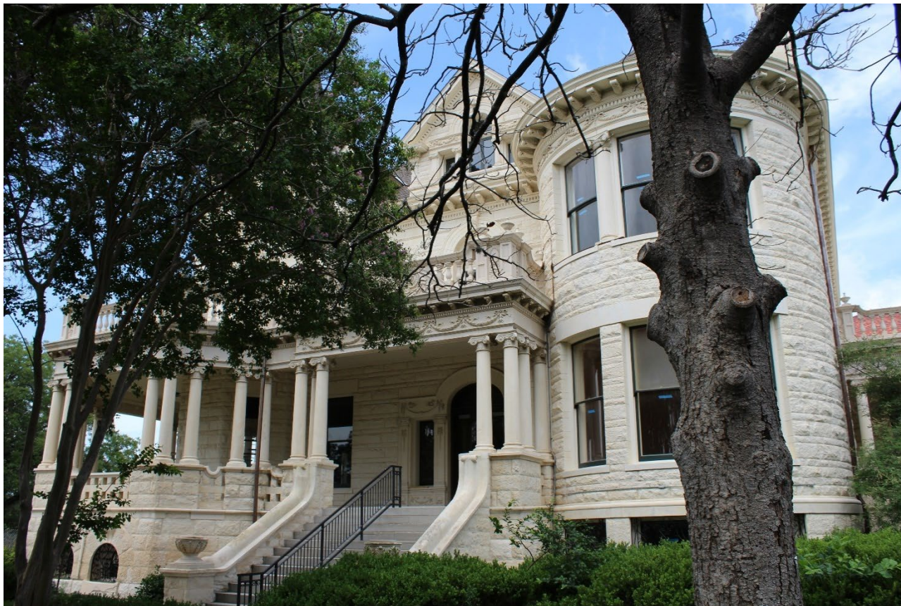
Photo 2. Koehler House - East elevation, camera facing west. June 11, 2025
