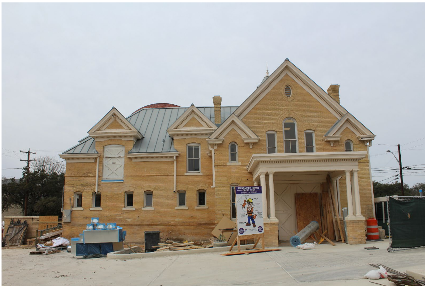
Photo 19. Carriage House – East elevation, camera facing west. January 30, 2026
