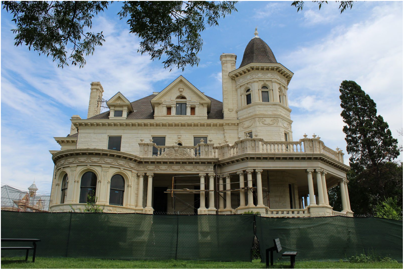
Photo 3. Koehler House - South elevation, camera facing north. June 11, 2025
