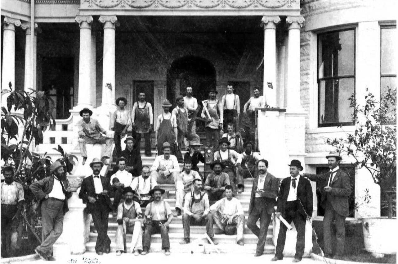
Figure 7. The craftsmen involved in construction work posed on the south porch; The architect, Card Seutter holds the plan. c 1900. Courtesy of San Antonio College Collection
