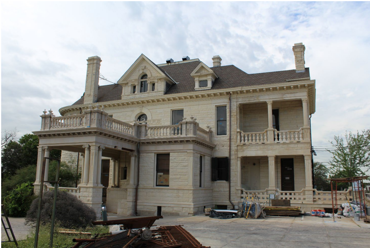
Photo 1. Koehler House - North elevation, camera facing southeast. June 11, 2025
