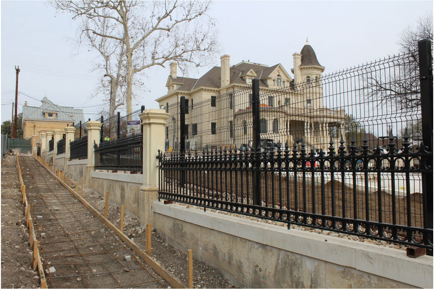
Photo 28. Ornamental limestone and metal perimeter fence - camera facing northeast. January 30, 2026
