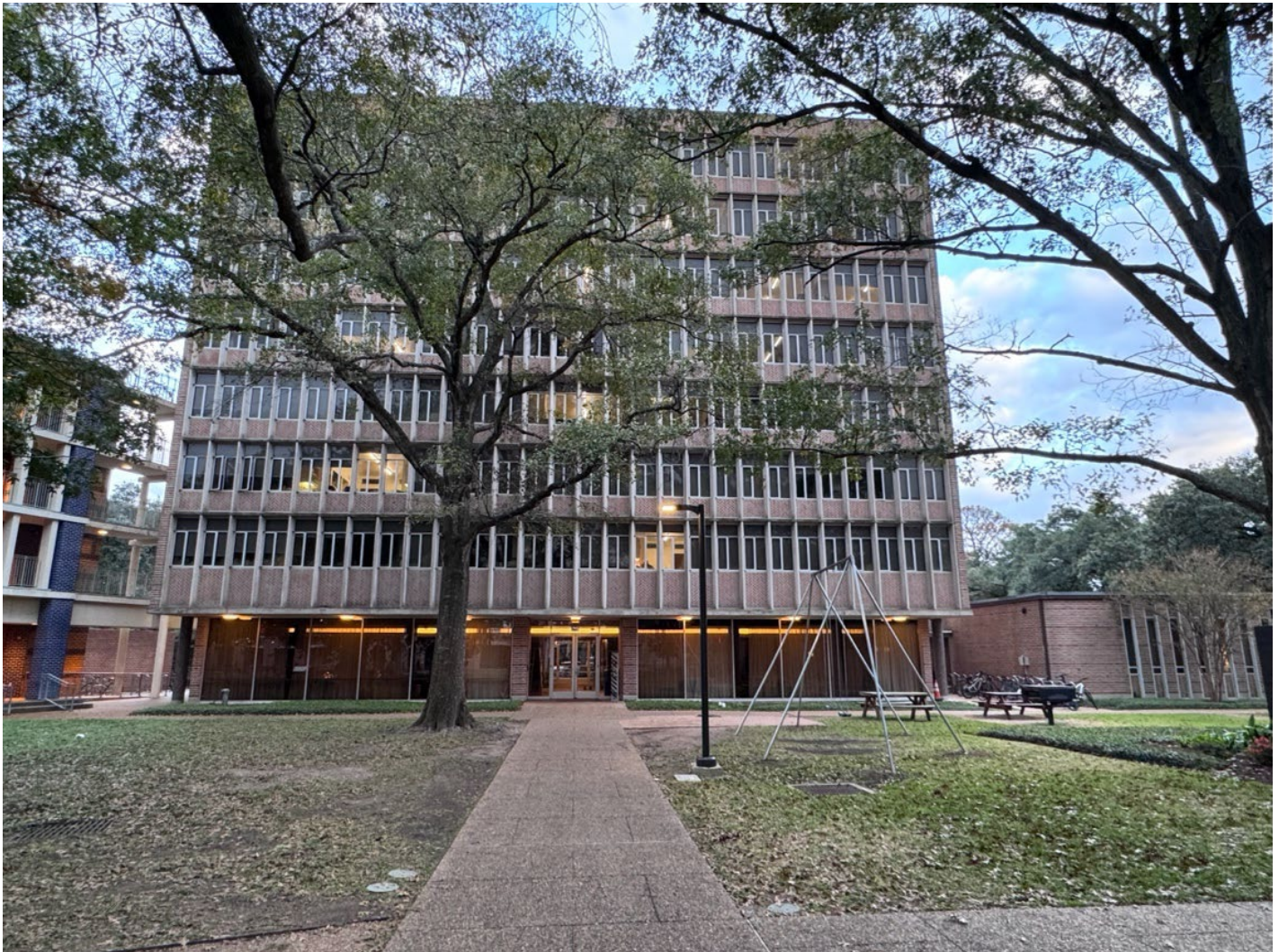
Photo 5. Brown College, west elevation, view east
