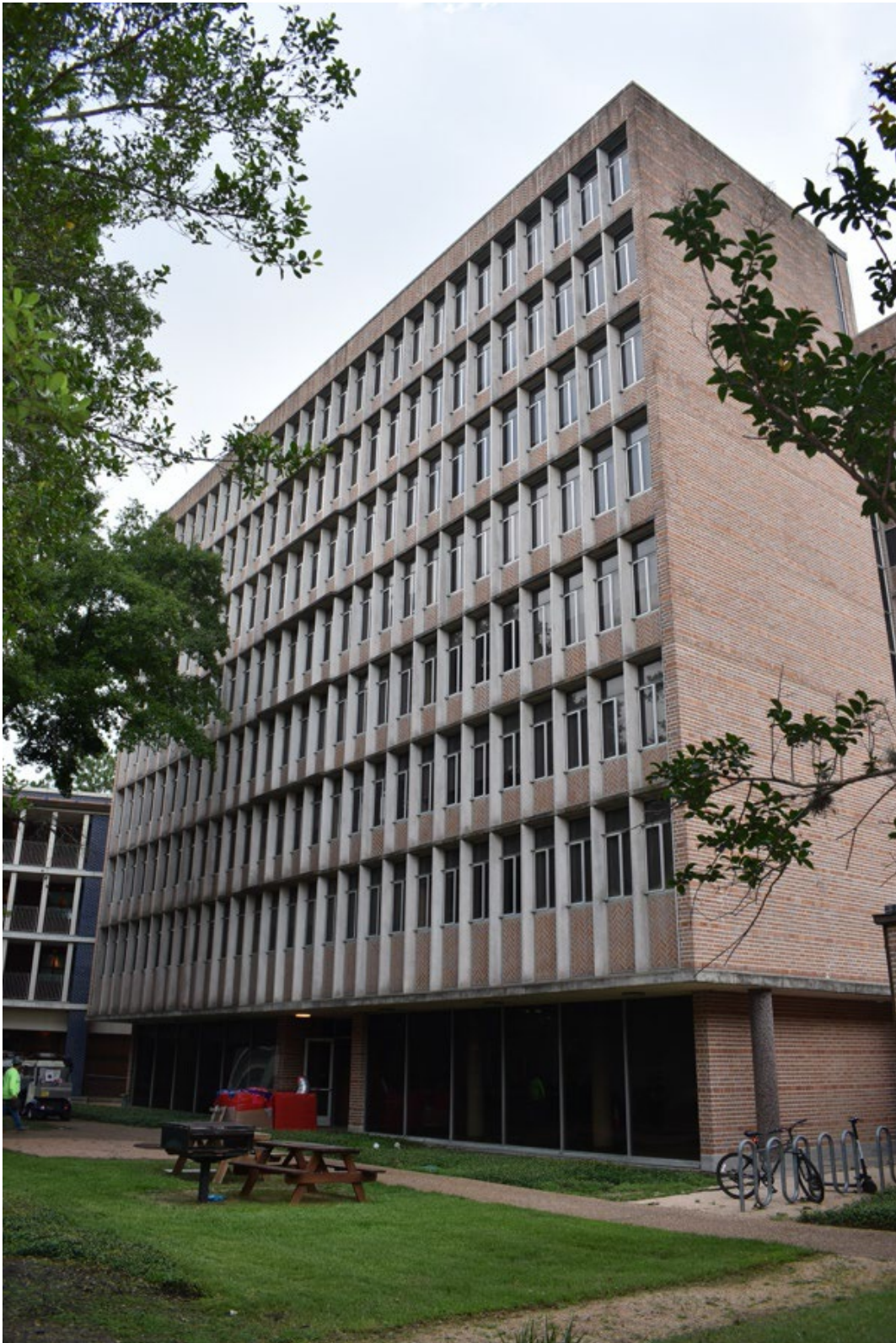
Photo 4. Oblique view: Brown College, west and south elevations, view northeast
