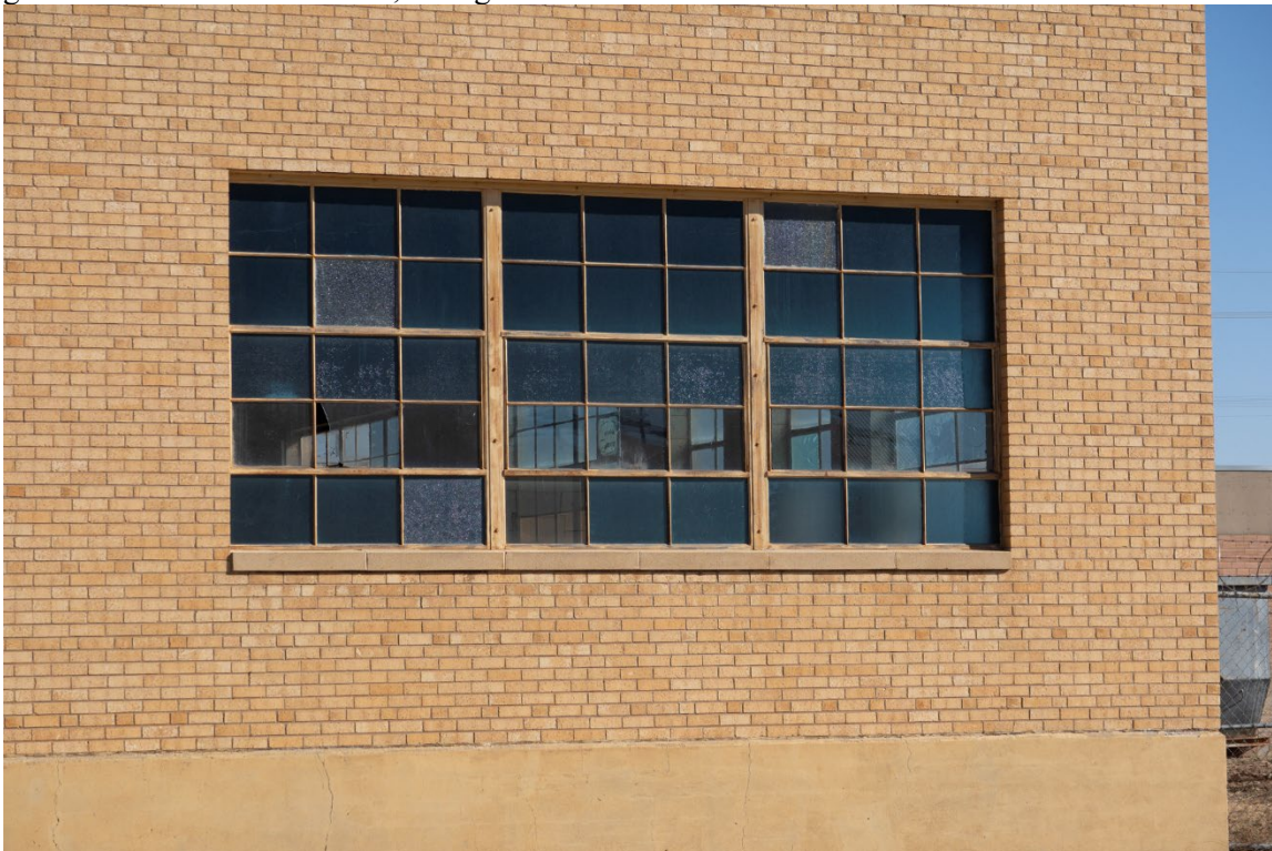
Photo 9. Original industrial windows consisting of textured blue-green glass (possibly Solex product) and band of clear glass in second to bottom row, facing east.
