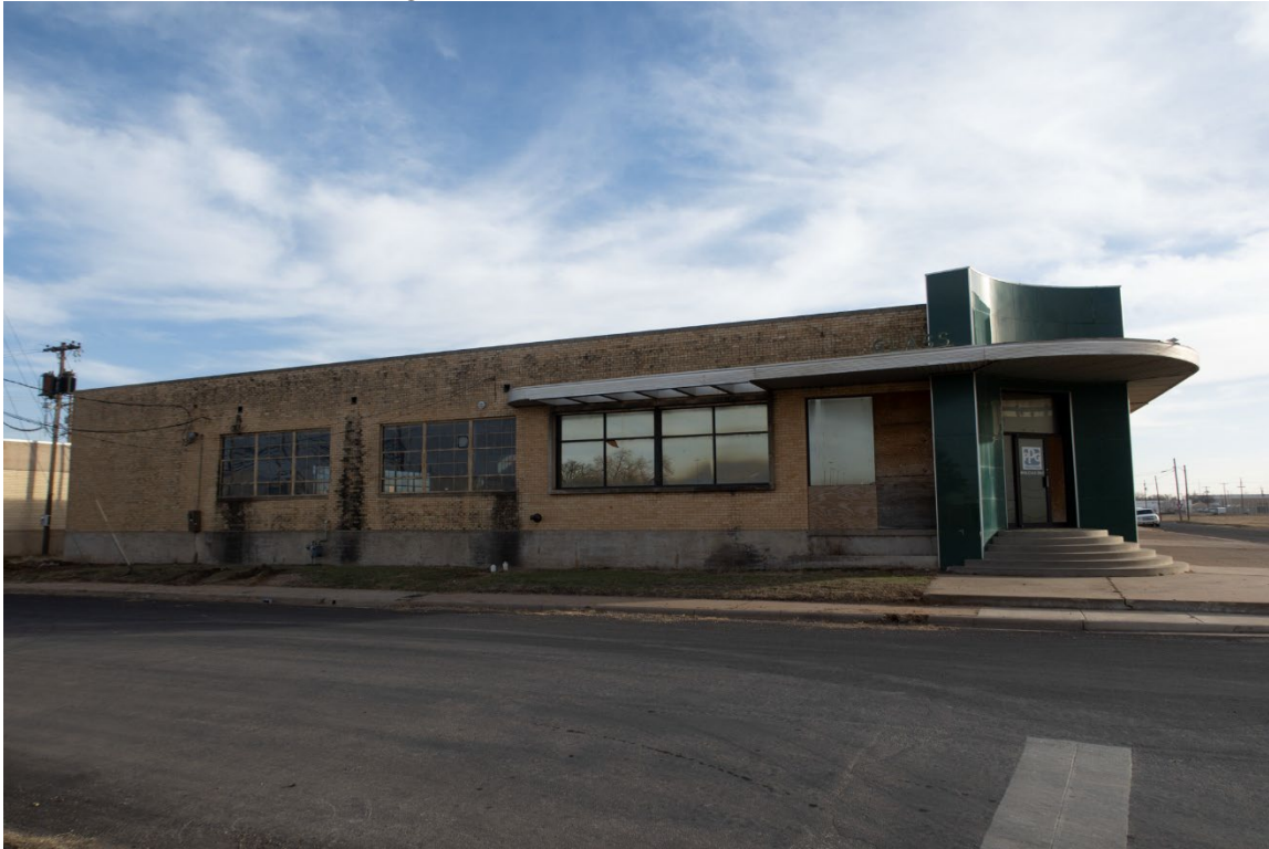
Photo 9. Original industrial windows consisting of textured blue-green glass (possibly Solex product) and band of clear glass in second to bottom row, facing east.
