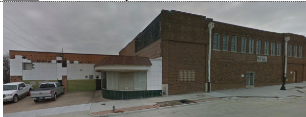
2017 street view—the property was extensively remodeled in 2018 and the Carrara glass (seen on center storefront) removed.
