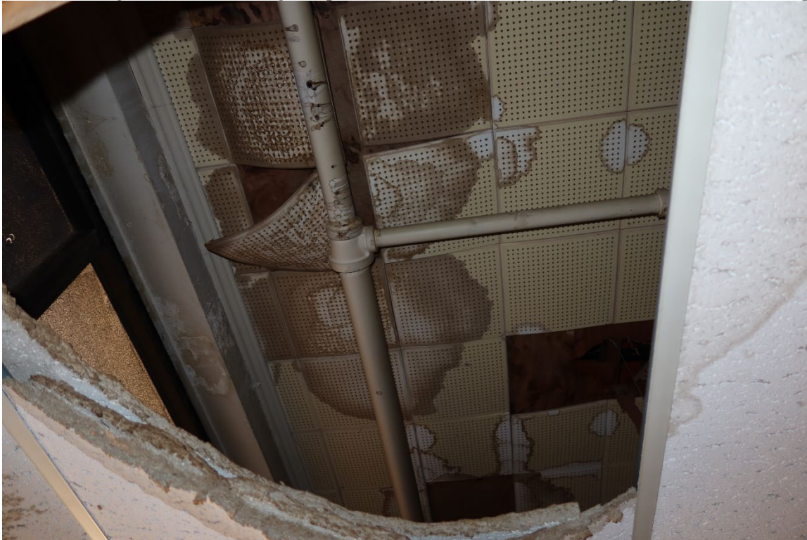
Photo 20: Original crown molding and plaster walls located above the drop ceiling in the office space.
