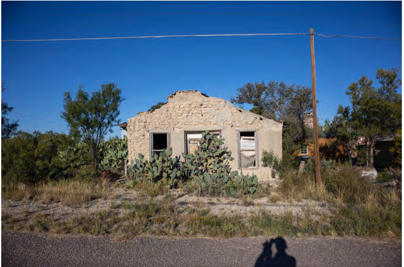
Photo 8. Abandoned adobe house (Site 70), 108 South 4 th Street East, second building on property, 2021 (see Figure 13)
