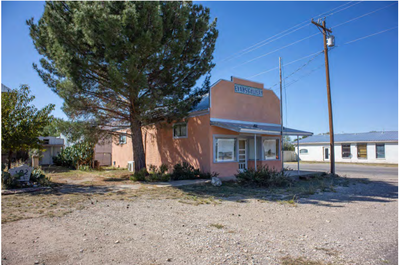
Photo 11. Evans Gallery (Site 5), southeast corner of South 1 st Street East and South Avenue D, 2021 (contributing)
