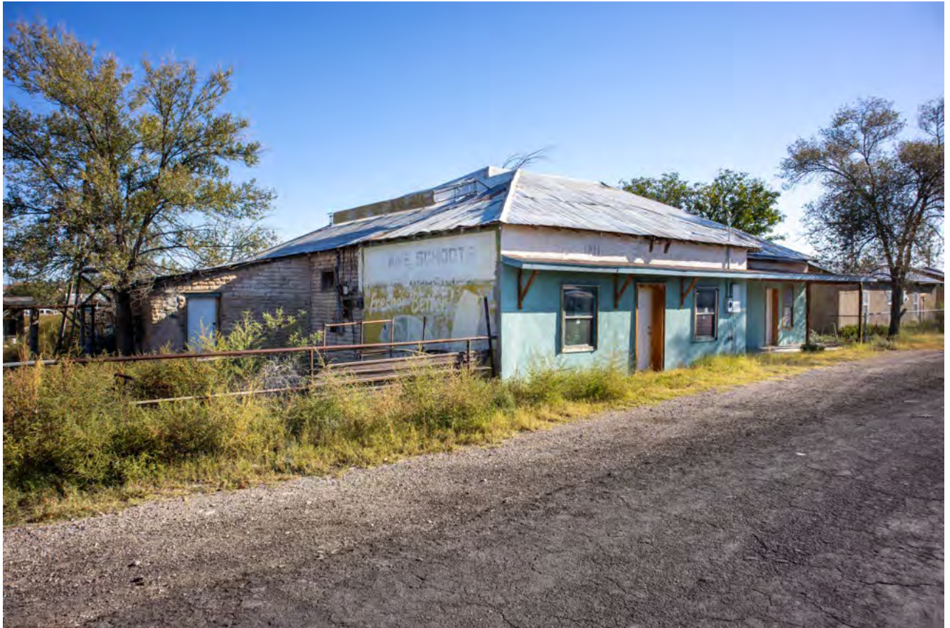
Photo 6. Former Mike Schodt's grocery store (Site 38), now a residence, South 4 th Street East, 2021 (contributing)
