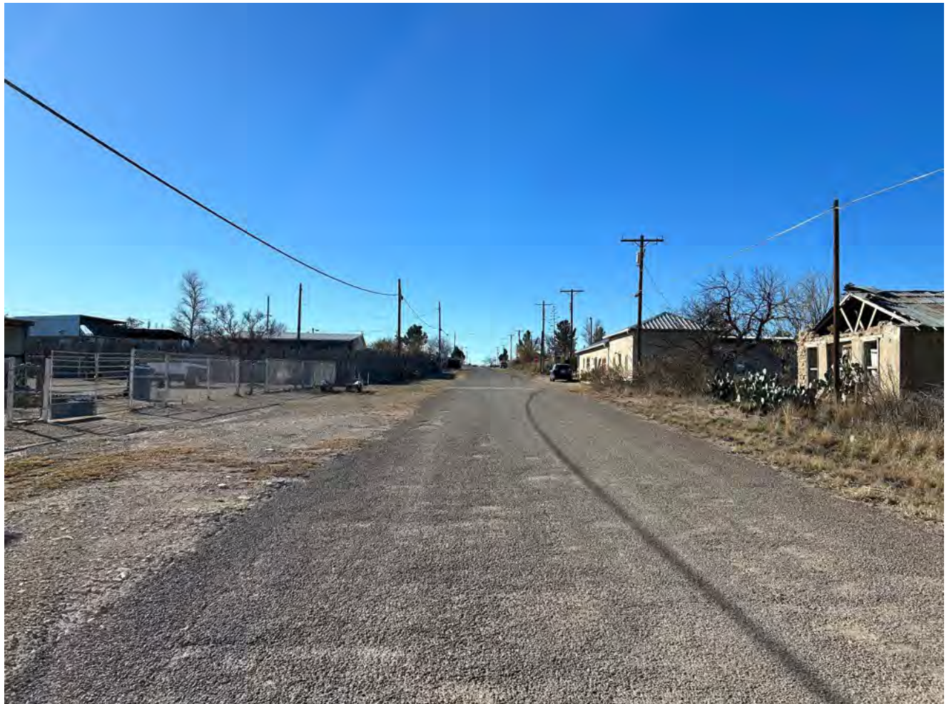
Photo 24. Streetscape, South 4 th Street at Avenue E, camera facing North, January 2023
