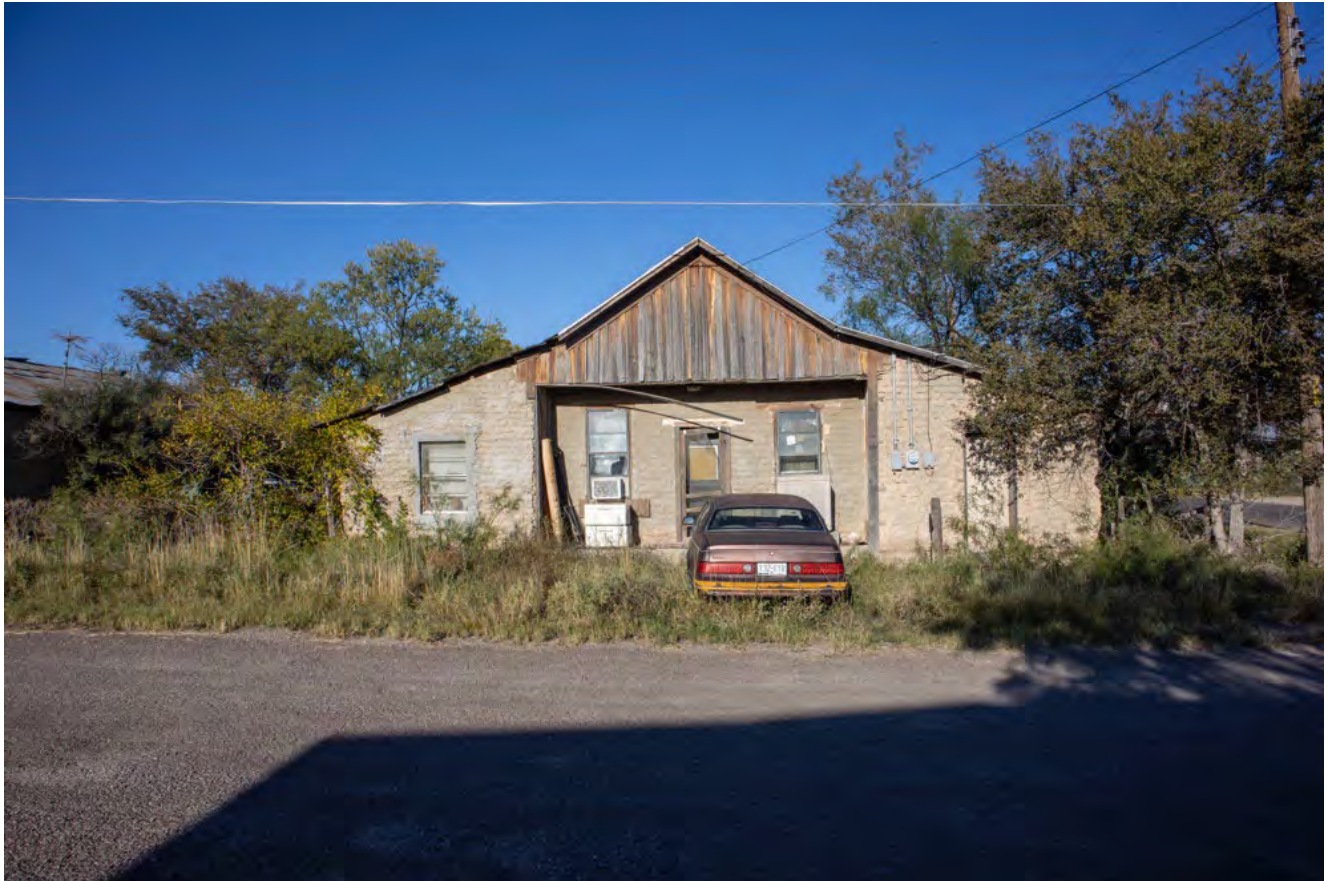
Photo 7. House at 108 South 4 th Street East (Site 70), 2021 (see Figure 12)
