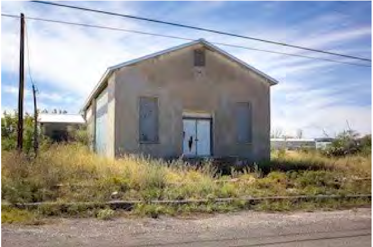
Photo 9. Hidalgo School (Site 128), southeast corner of South Avenue D and South 6 th Street East, 2021 (contributing)
