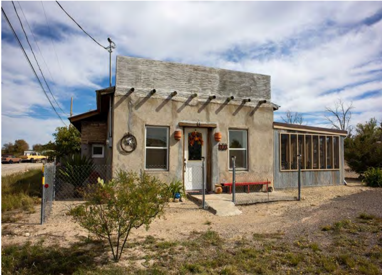
Photo 16. Ca. 1900 historic adobe house (Site 121) severely altered to add faux vigas, new parapet, and screened-in porch, southeast corner of South Avenue F and South 5 th Street East, 2021 (noncontributing)
