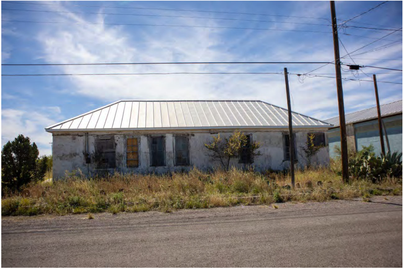
Photo 10. Hidalgo School Recreation Hall (Site 129), southeast corner of South Avenue D and South 6 th Street East, 2021 (contributing)
