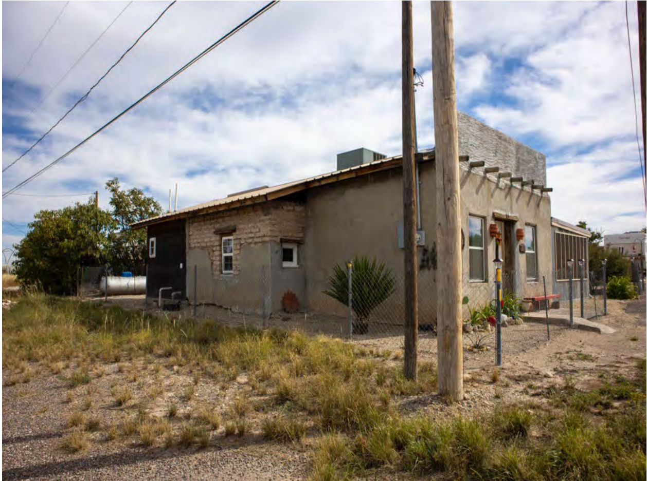
Photo 17. The same house (Site 121), oblique view to show the purposefully exposed adobe and white vinyl windows on the north side of the building.
