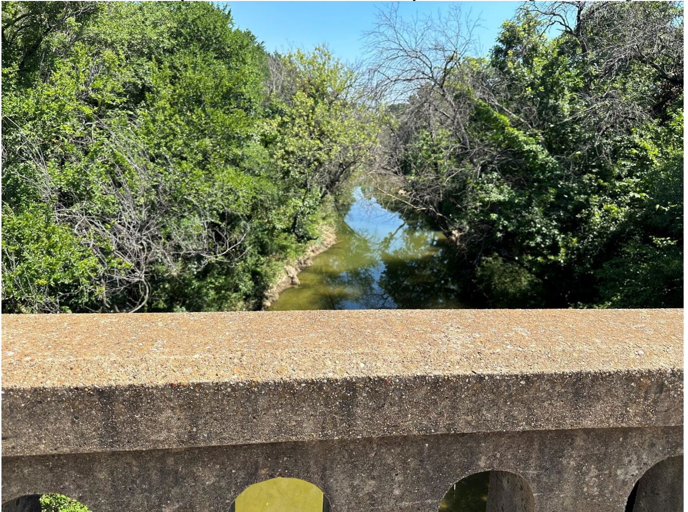
Photo 13. Contextual view of Sycamore Creek from the street level of Sycamore Creek Bridge. Camera facing north.
