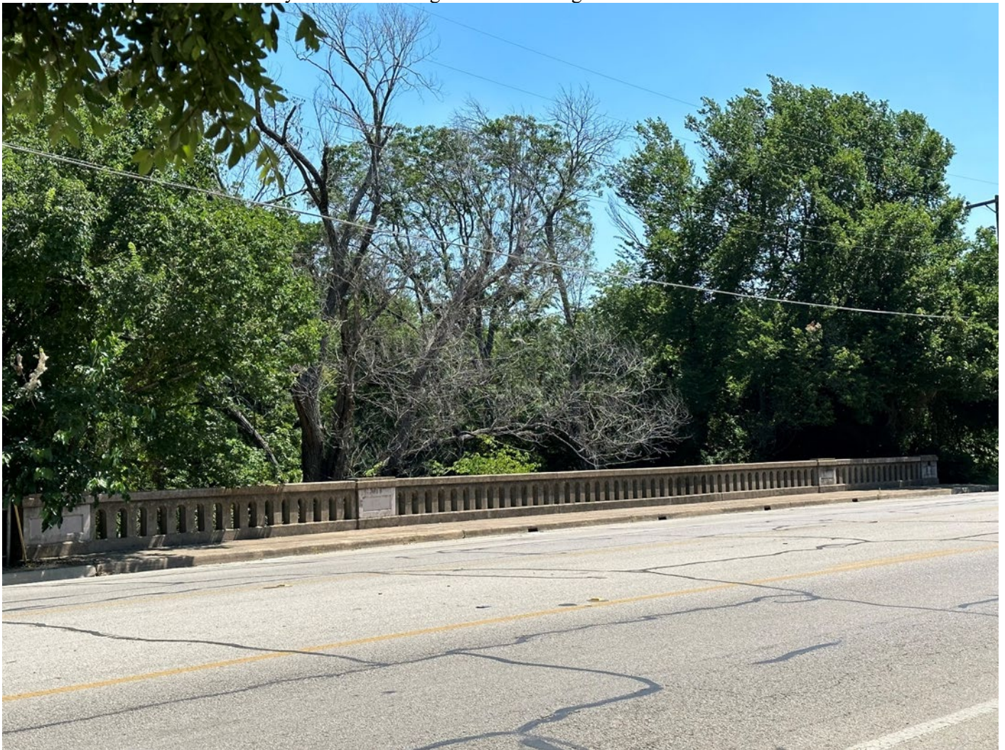
Photo 14. Oblique view of Vickery Boulevard Bridge. Camera facing north.
