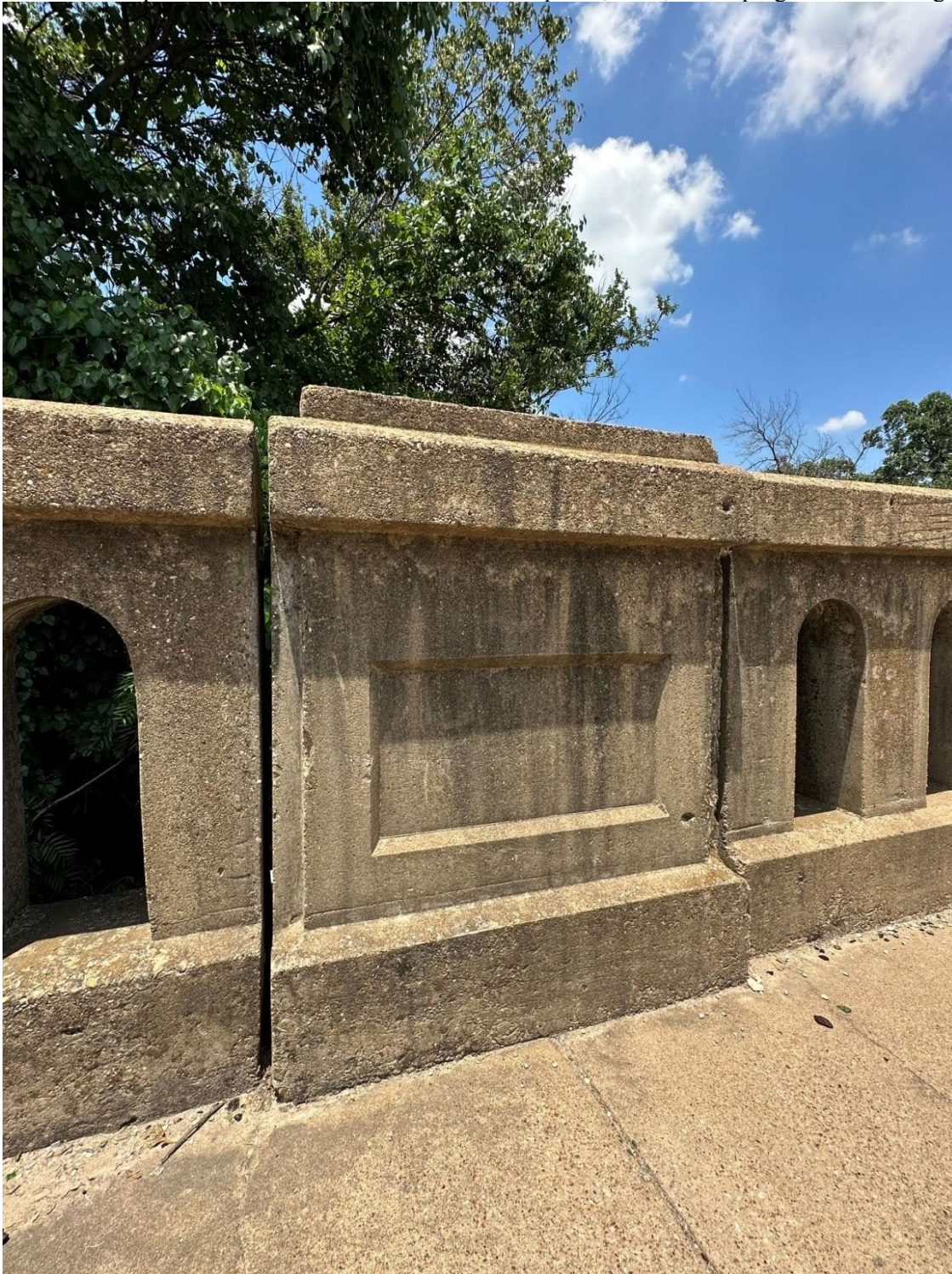
Photo 3. Oblique detail view of column with classical plinth, dado, and coping. Camera facing north.
