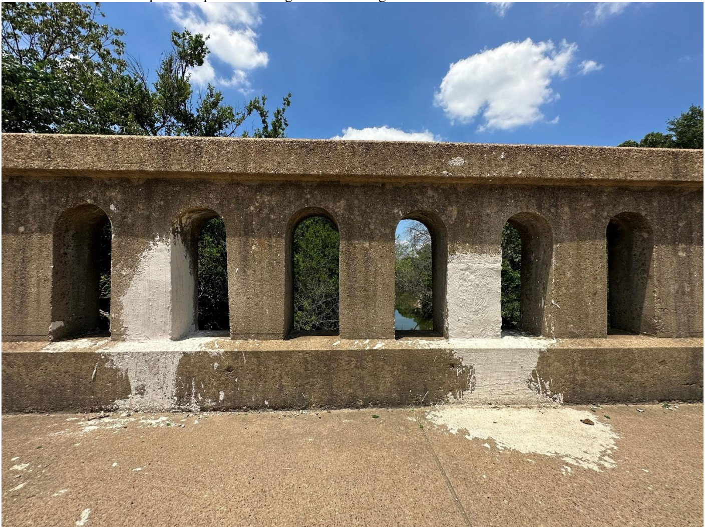
Photo 11. Detail view of plaster repairs on railing. Camera facing north.
