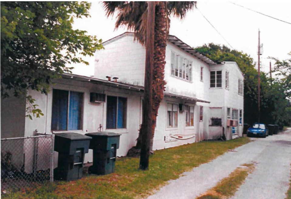
Figure 7. St. Augustine of Hippo Episcopal Church parish hall and rectory, south elevation, as it appeared in 2002
