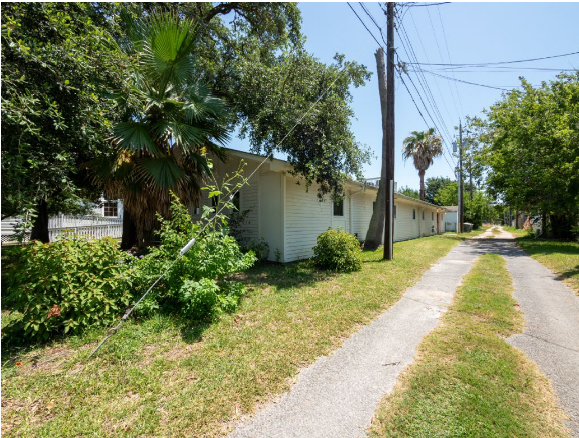
Photo 7. Parish Hall, south elevation, camera facing northeast.
