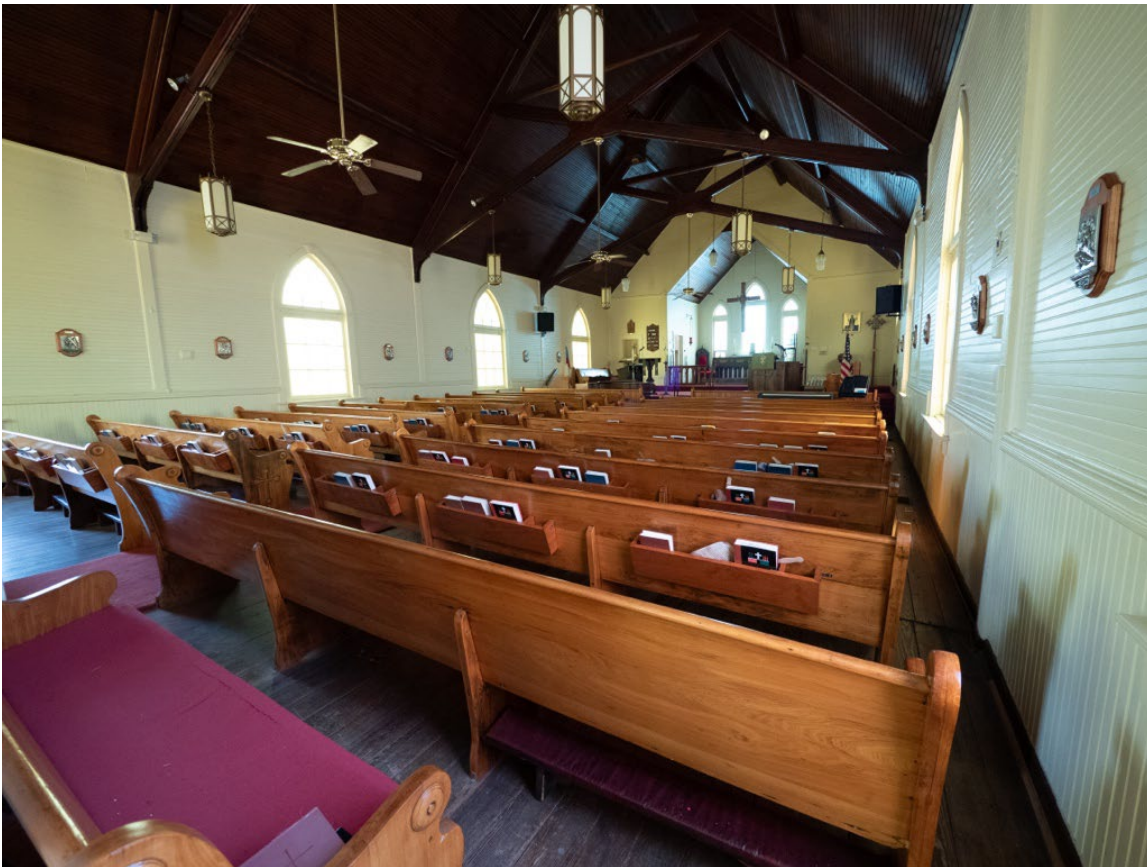
Photo 13. Nave, view from southeast corner, camera facing east.
