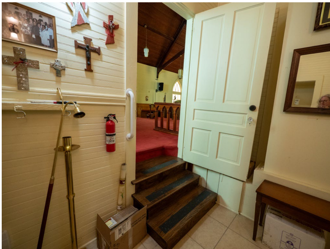
Photo 18. Stairs from Chancel into Sacristy, camera facing southwest.
