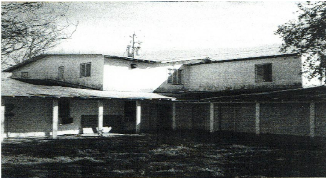
Figure 8. St. Augustine of Hippo Episcopal Church parish hall and rectory, north and west elevations, as it appeared in 2009 after Hurricane Ike and prior to demolition
