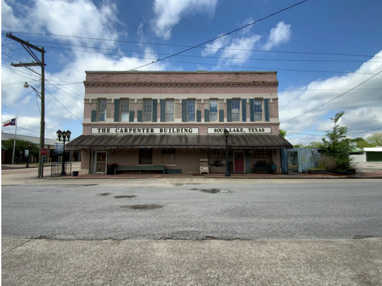
Photo 15. 730 Sixth Street. Carpenter Building (constructed 1903). Camera facing west.
