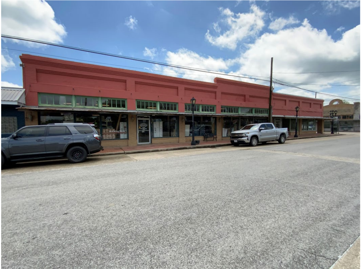
Photo 4. 100 Block of Merchant Street (constructed 1916). Left to right: 135 Merchant Street and 125 Merchant Street. Camera facing southeast.
