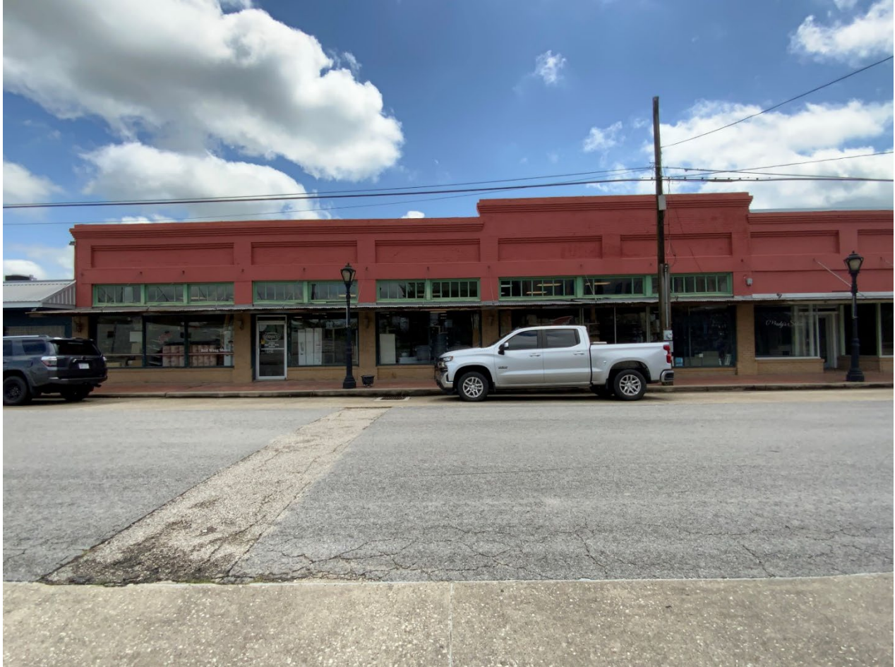
Photo 14. 135 Merchant Street (constructed 1916). Camera facing east.
