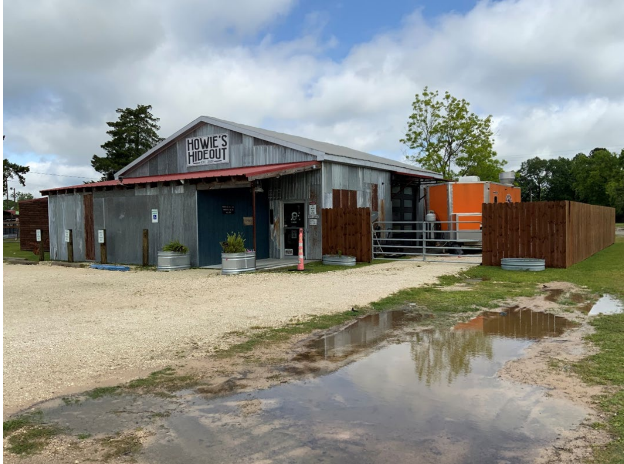
Photo 7. 650 Sixth Street. Workshop Building (constructed 1950). Camera facing northeast.
