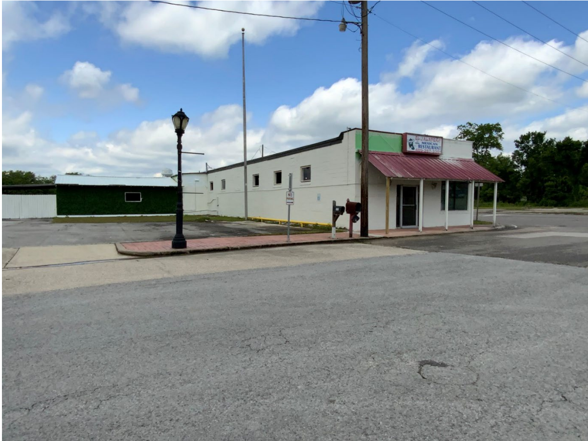
Photo 6. Northwest Merchant Street, showing 104 Merchant Street, a contributing resource.
