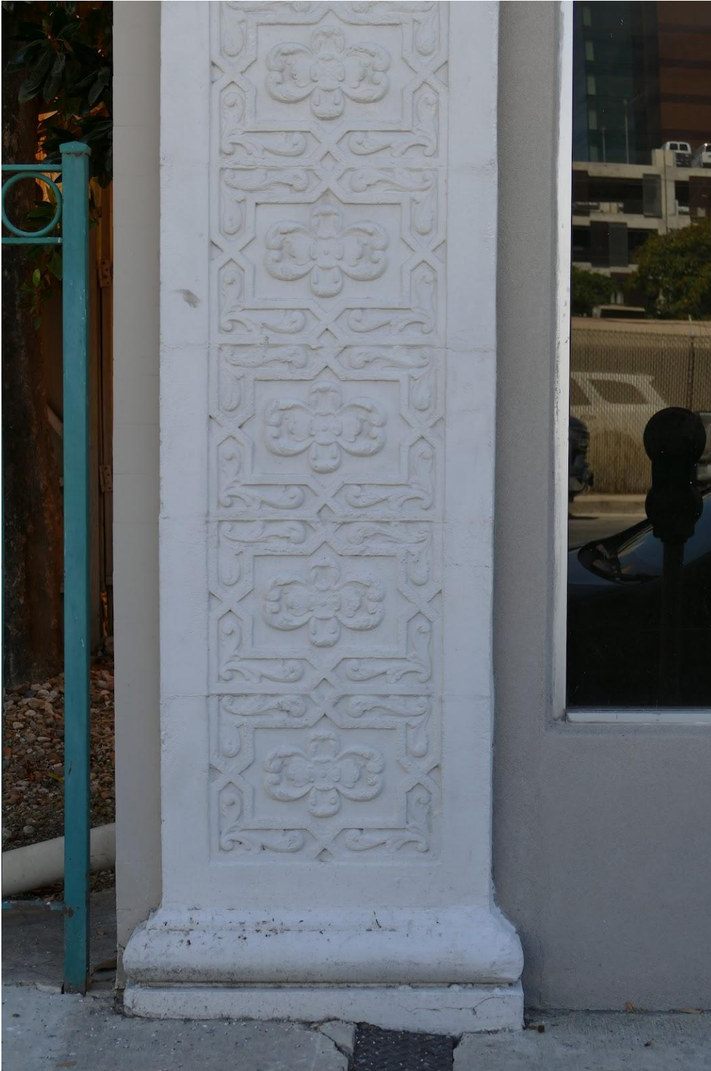
Photo 3: Detail view of cast stone pilasters on San Antonio Tent & Awning Company, view east.
