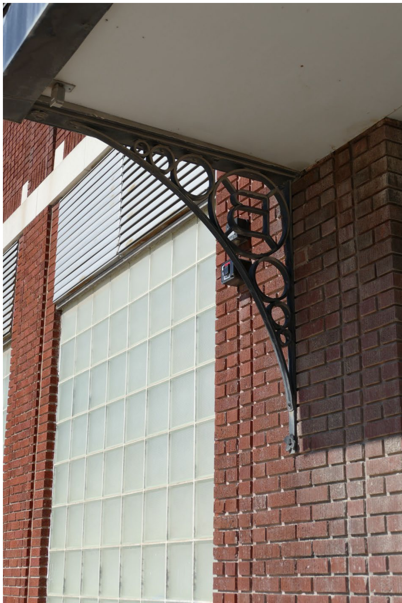
Photo 7: Canopy bracket and tie rod detail with “B” for Buick, view west.
