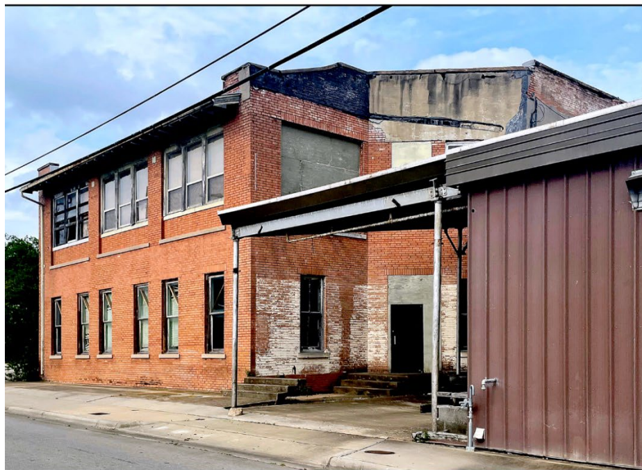
April 26, 2024 Porch infilled with windows and brick.
