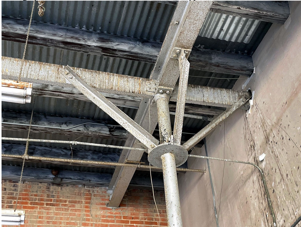
Photograph 25: View of structural brackets for canopy over service dock. Camera Direction: East
