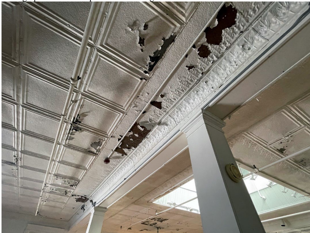
Photograph 36: View of pressed tin ceiling on second floor of office addition. Camera Direction: Northwest
