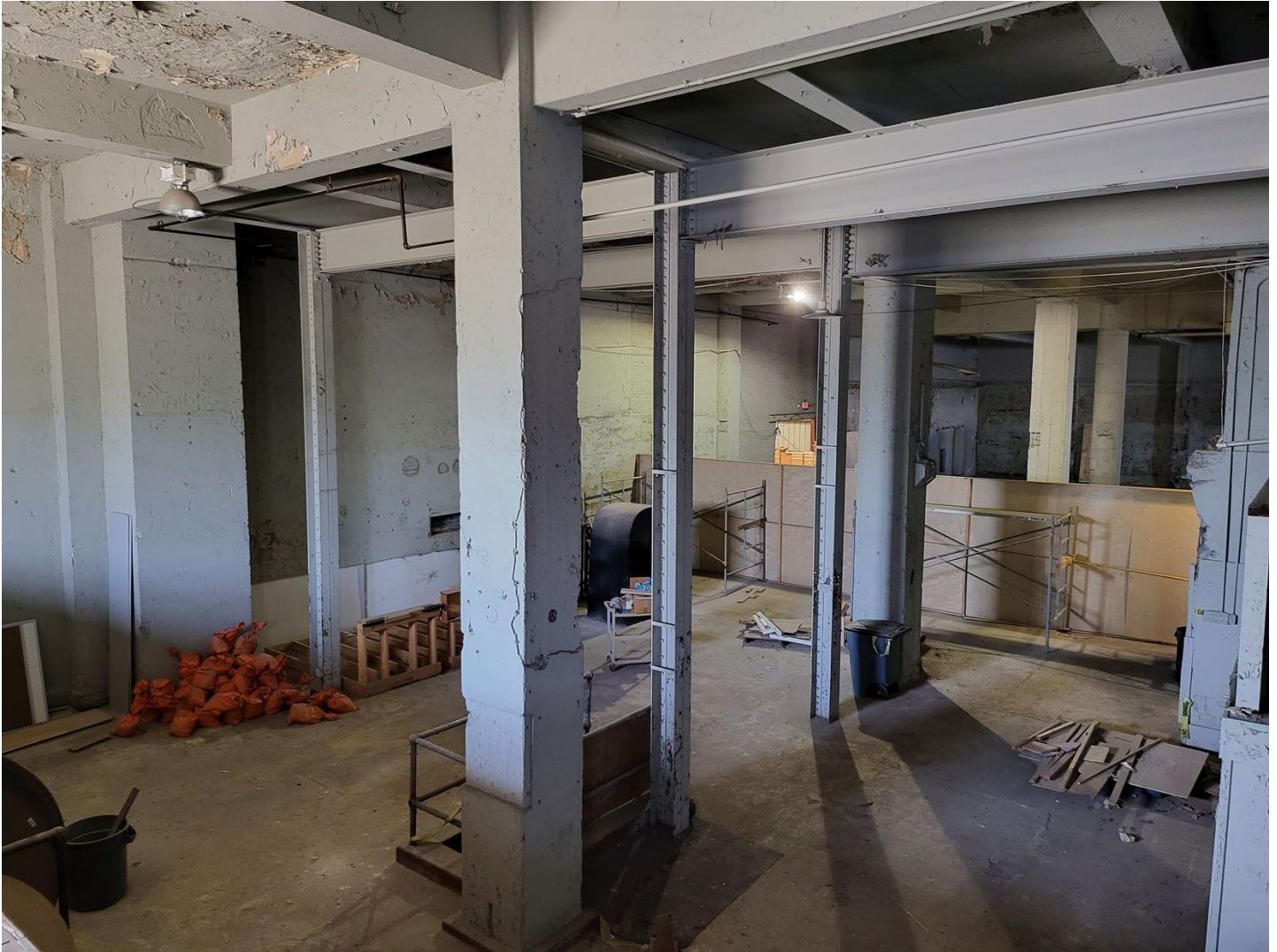
Photo 15: First floor refrigerating room. The original concrete mezzanine catwalk has been removed with metal shoring added to support the floor above which was damaged from extended exposure to ice and salt. Stair to boiler room is at bottom center. Facing southwest.
