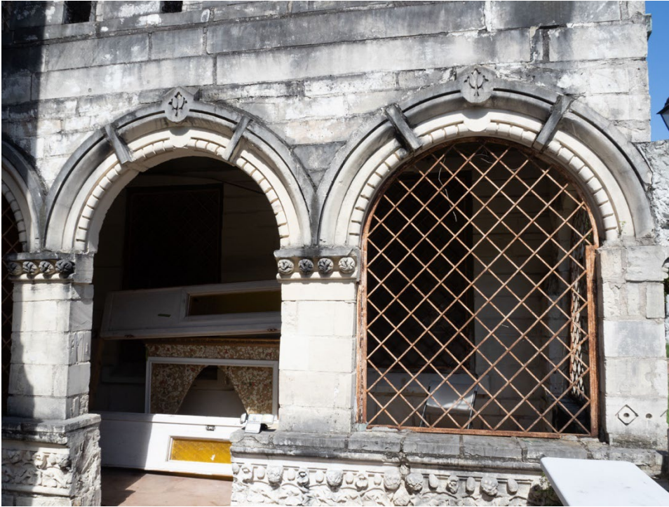
Photo 12. Cast stone frieze detail below front entry arches, camera facing east.
