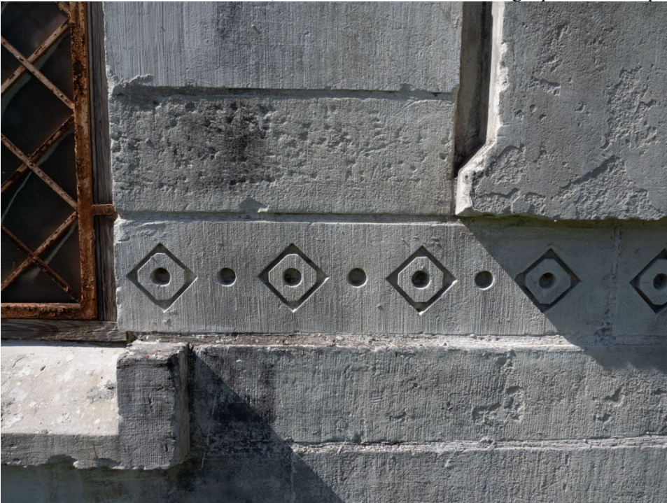
Photo 10. Cast stone block detail, round circles with alternating squares set on point, front elevation, camera facing north.
