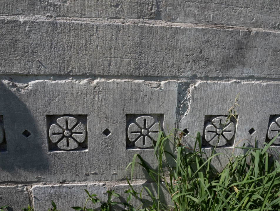
Photo 10. Cast stone block detail, round circles with alternating squares set on point, front elevation, camera facing north.
