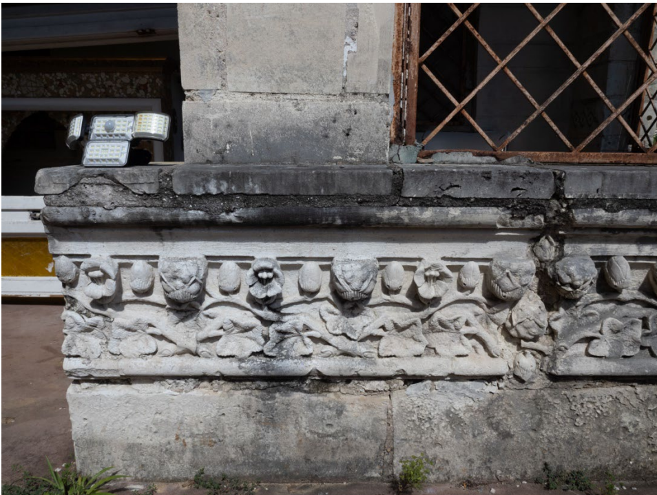
Photo 12. Cast stone frieze detail below front entry arches, camera facing east.
