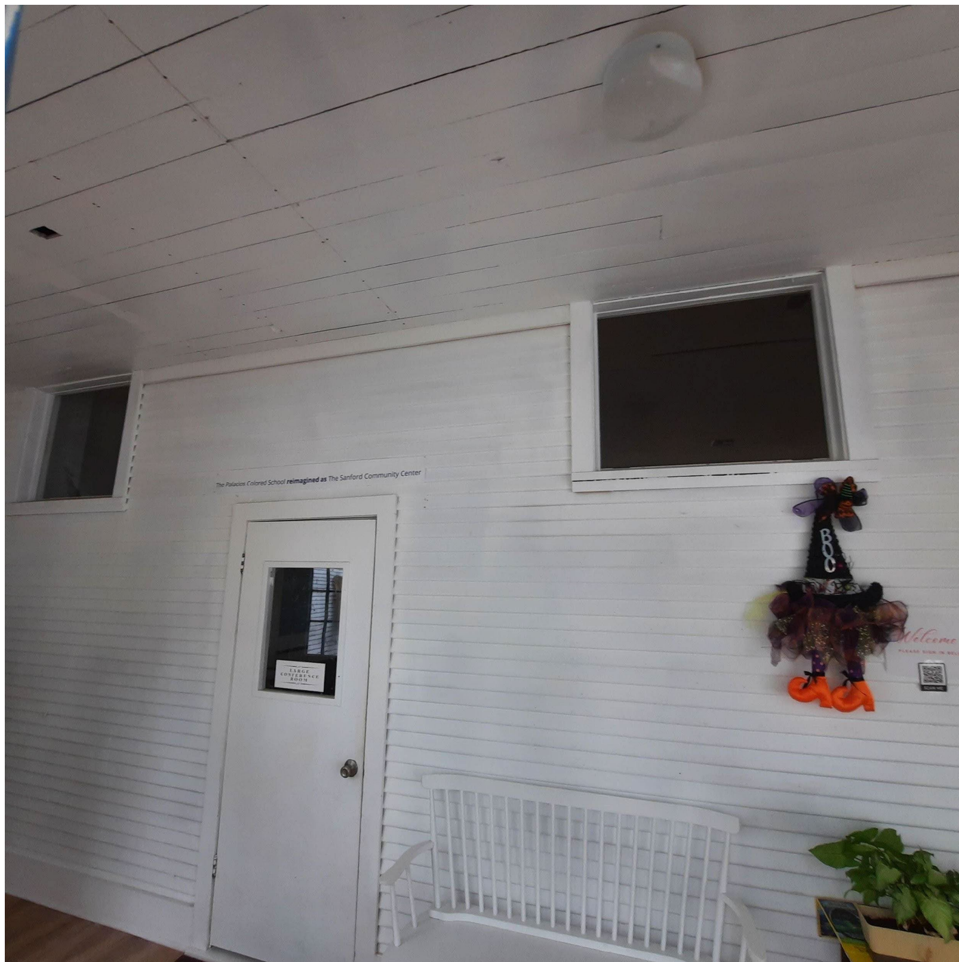
Photo 13 - Original plank ceiling.
