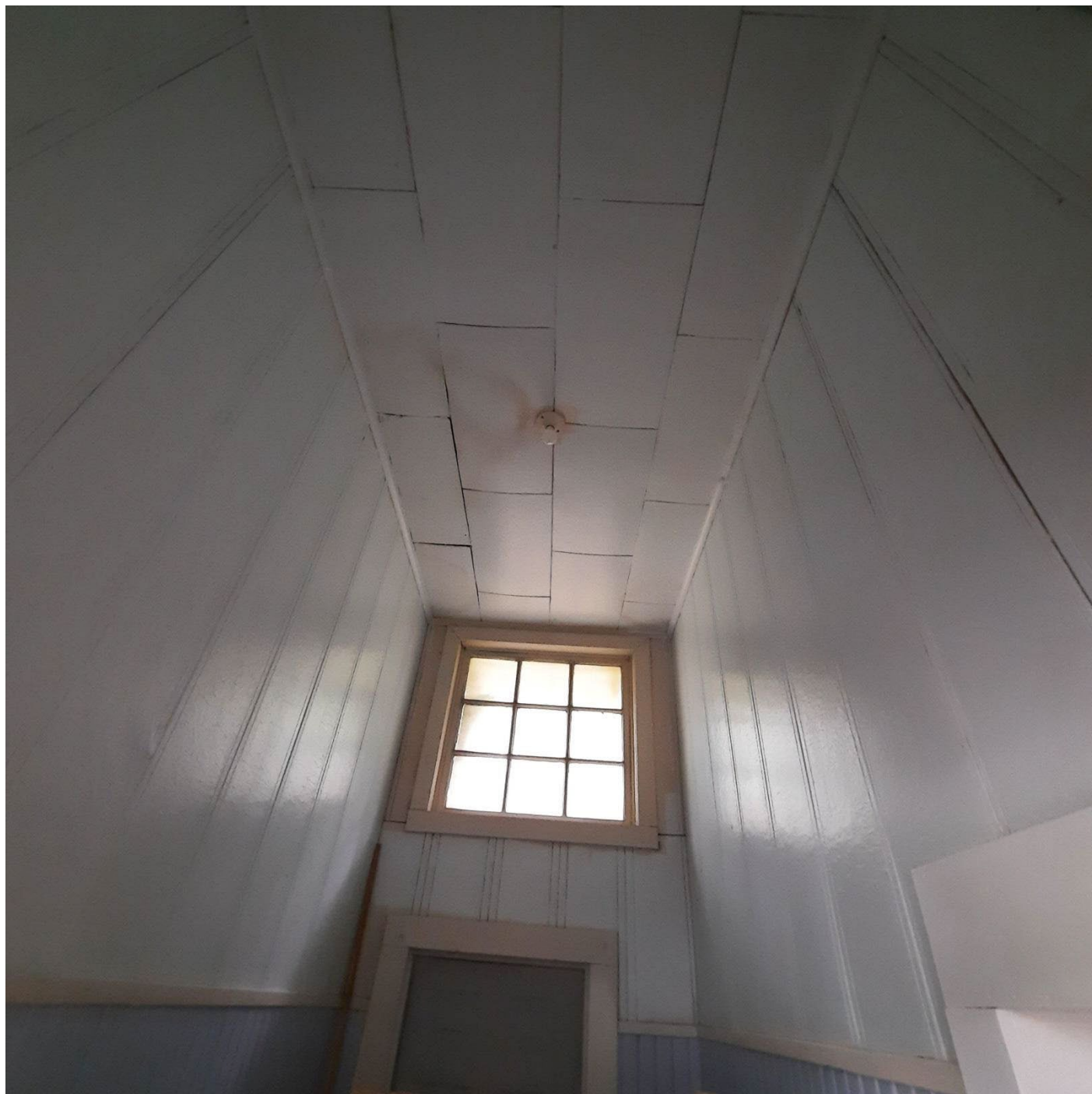
Photo 15 - Fiberboard ceiling and wood walls in storage room.
