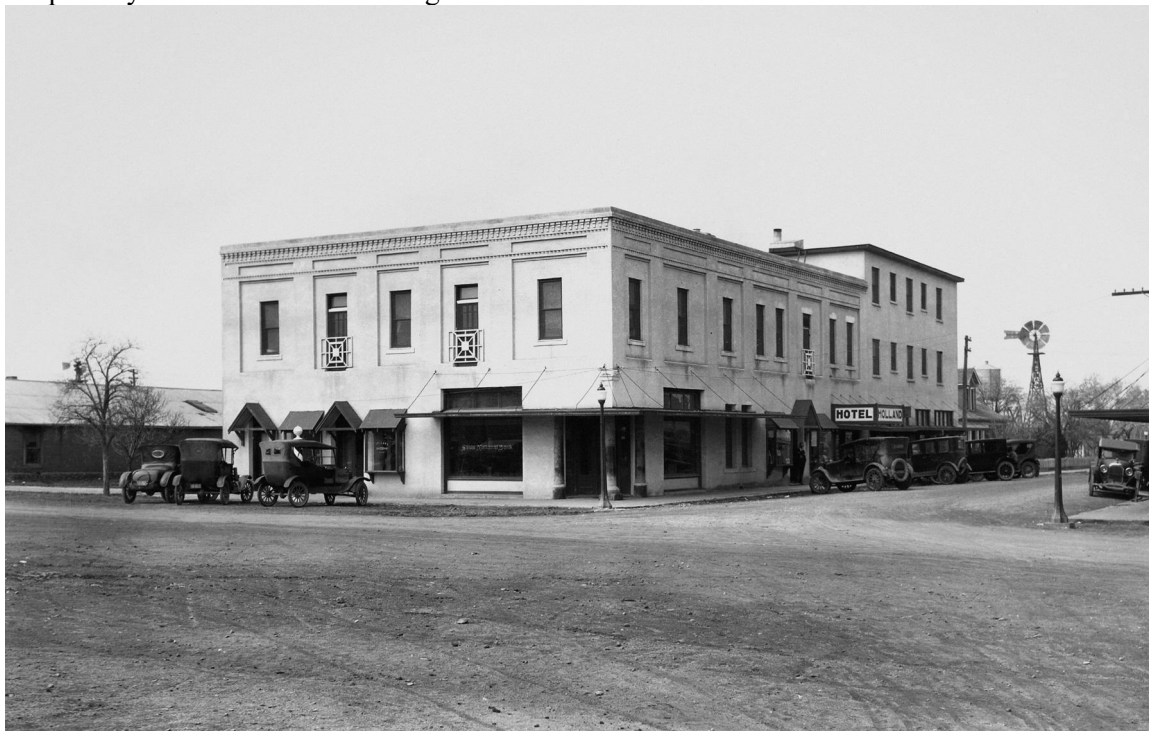
Figure 4. Holland Hotel after completion of 1923 rear addition and renovations. Stucco was applied to the exterior, the second story porch was removed and doors sealed, and new awnings were added above the first-floor windows. Note the primary entrance is located along N. 6th Street.
