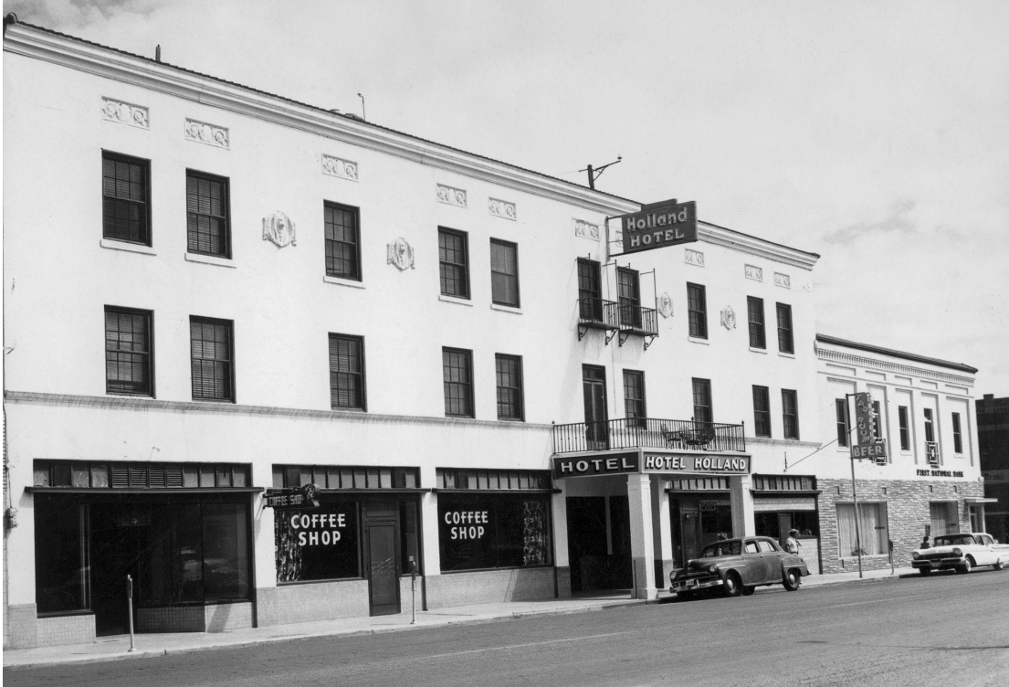
Figure 20. Circa 1960 photo of Holland Hotel. View Northeast. Note addition of faux-stacked stone on the first floor of the 1907 building and the reconfiguration of the formerly clipped corner entrance. Source: Holland Hotel
