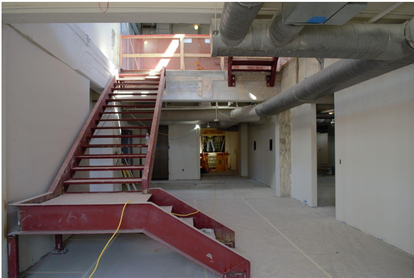
Photo 8: South end of basement showing slab cut for new stairs, looking north.
