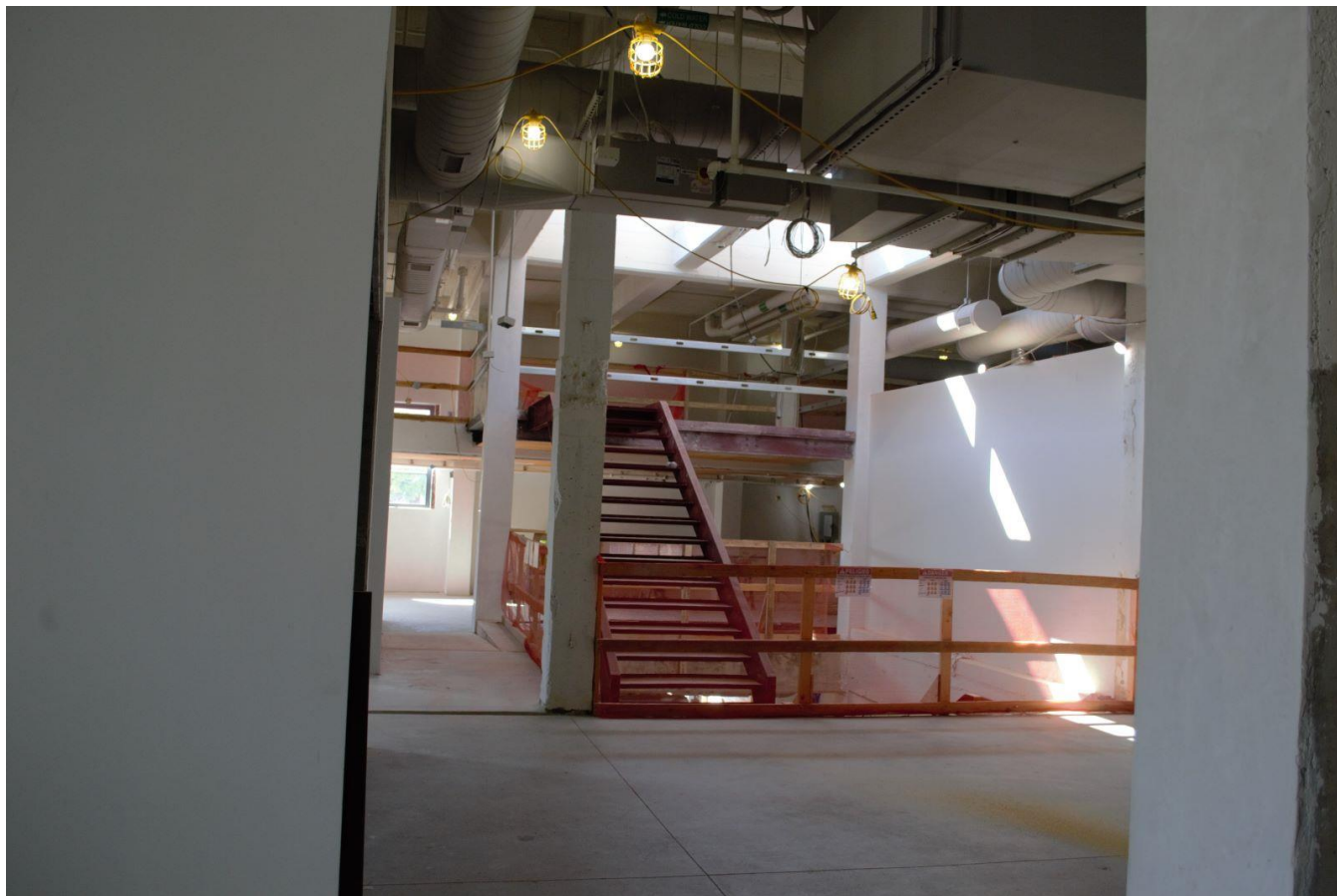
Photo 12: South end of first floor with slab cut for new stairs and mezzanine in the background, looking southwest.
