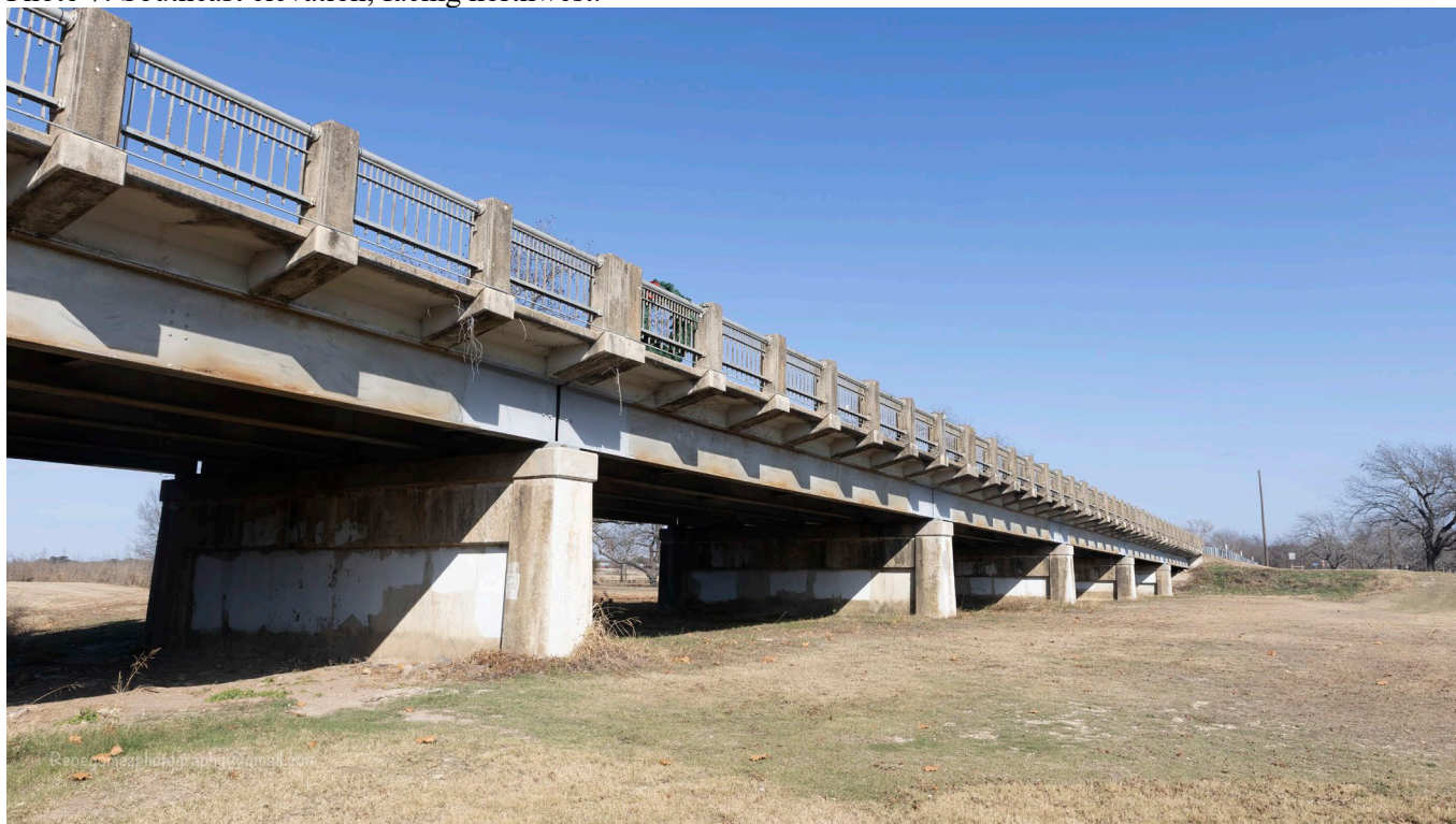
Photo 8: Balustrades are steel picket with concrete posts and are the bridge's primary ornamental feature. Camera facing south.
