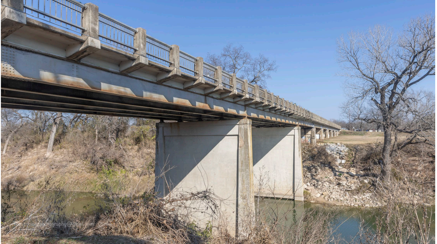
Photo 2: Concrete piers support the 265-foot-long span over the river's main channel. Camera facing northwest.
