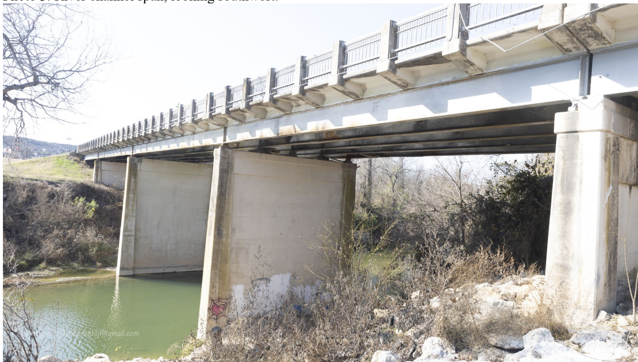
Photo 4: Steel I-beams form the superstructure. Camera facing north.
