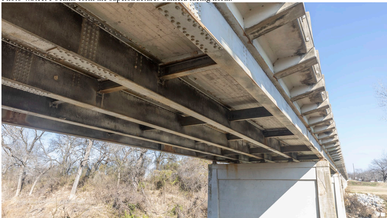
Photo 4: Steel I-beams form the superstructure. Camera facing north.
