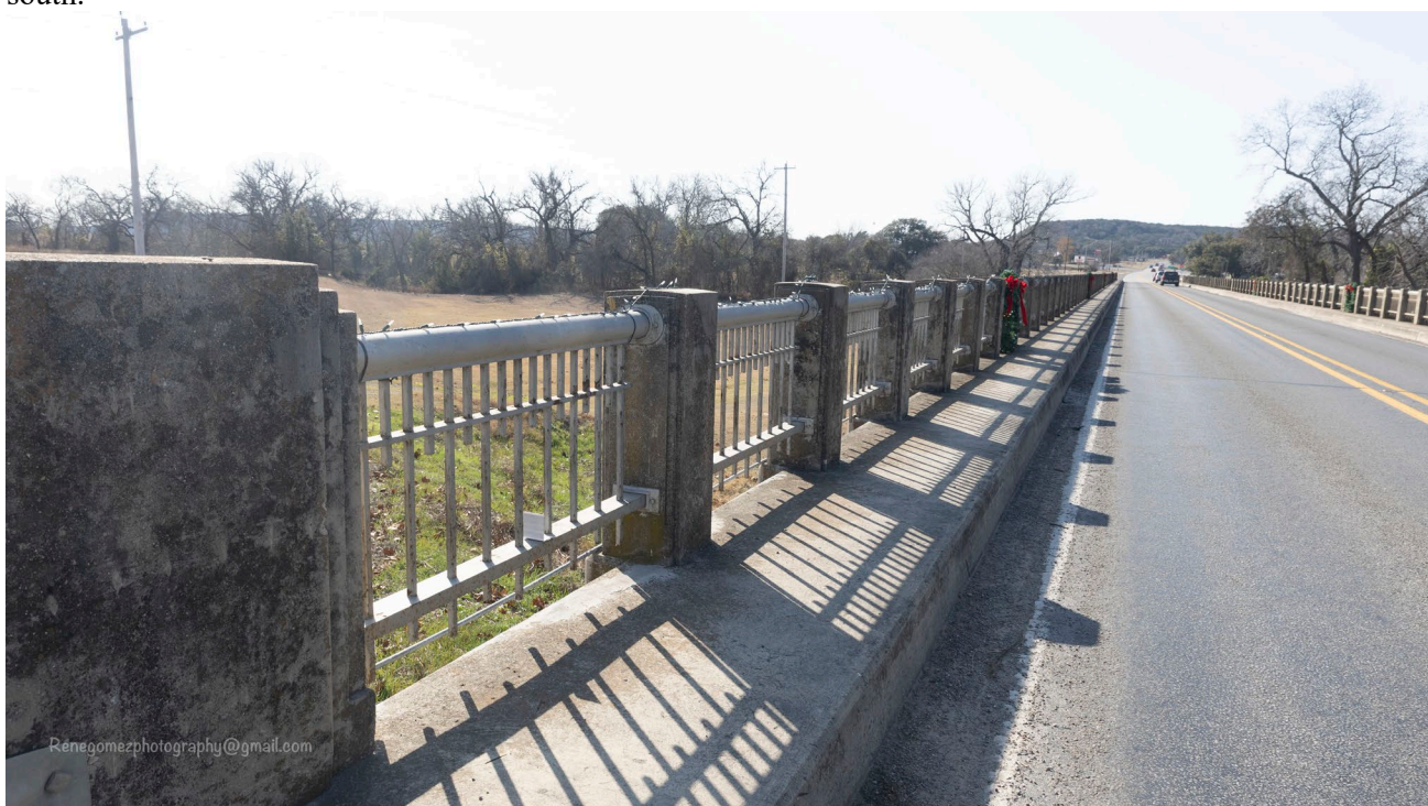
Photo 8: Balustrades are steel picket with concrete posts and are the bridge's primary ornamental feature. Camera facing south.
